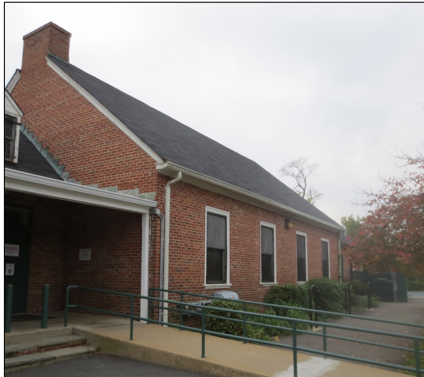
Figure 6. Front elevation of the central unit, looking west (EHT Tracerics, 2014).
