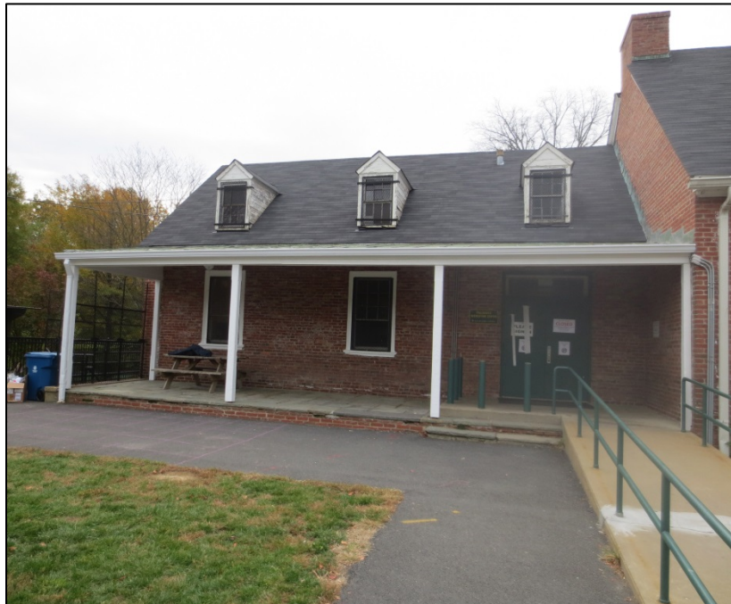
Figure 5. Front elevation of the eastern unit, looking south (EHT Traceries, 2014).
