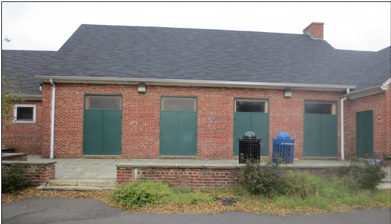
Figure 11. Rear elevation of the central unit, looking north (EHT Tracerics, 2014).
