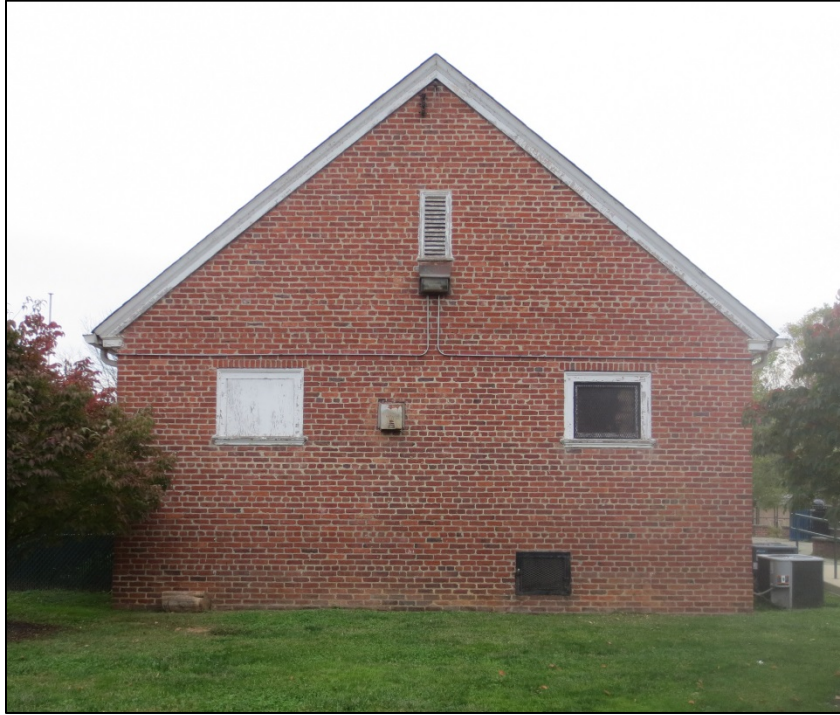
Figure 8. West elevation, looking east (EHT Tracerics, 2014).
