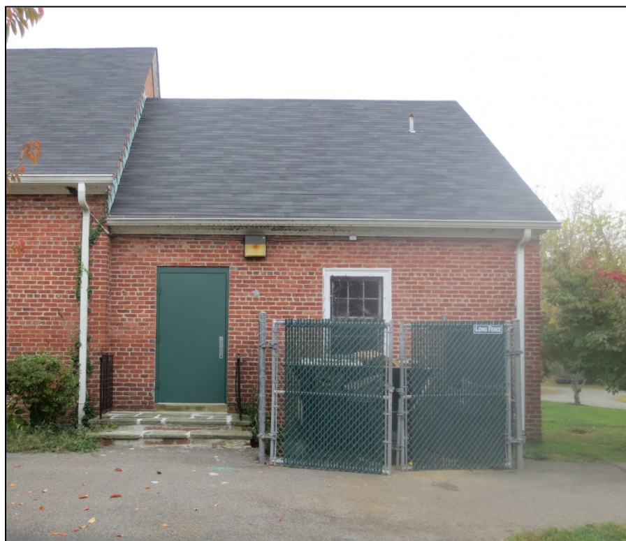
Figure 7. Front Elevation of the west unit, looking south (EHT Tracerics, 2014).
