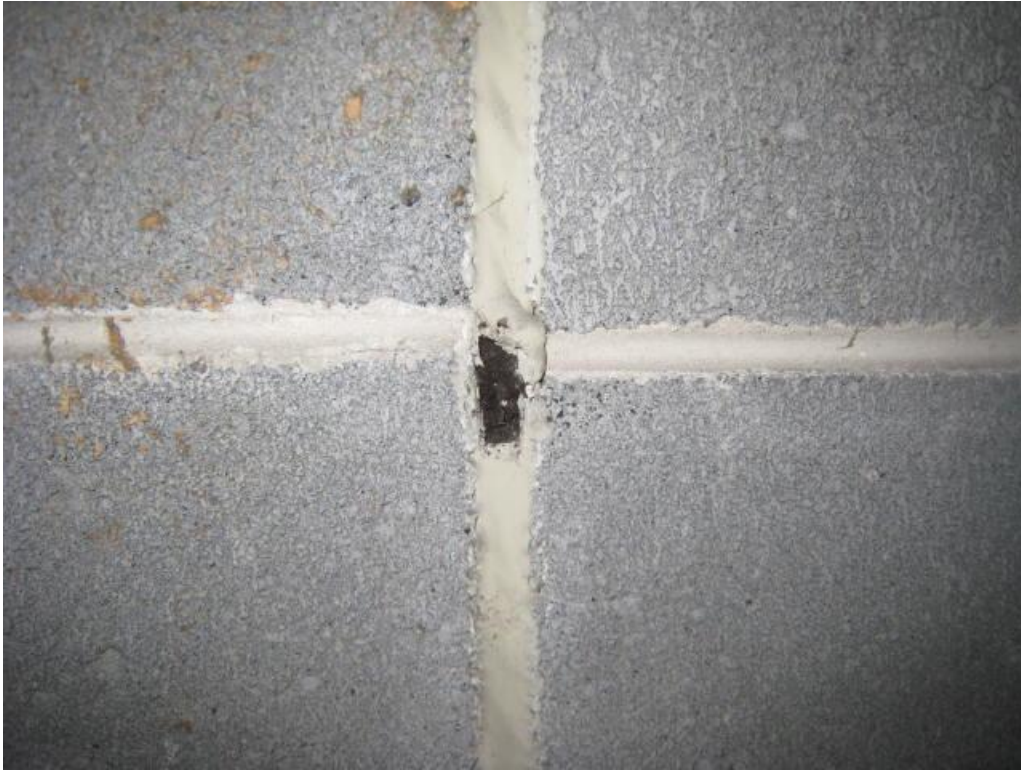
Photo 7 –View of Expansion Joint - Wall Sample 2850-0512-19
