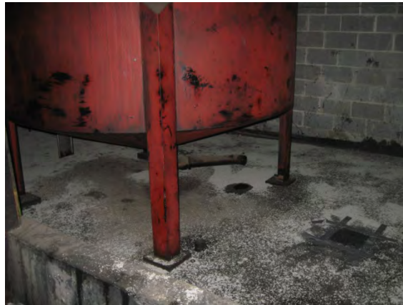
Photograph 5: Ink mixing tank berm with standing pools of ink.
