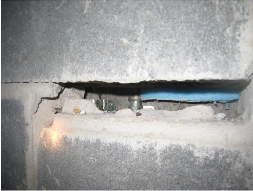
Photo 3 –View of CMU Mortar Sample 2850-0512-01
