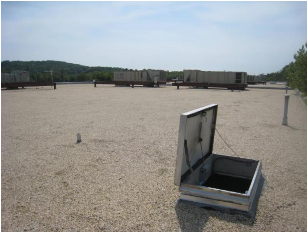
Photo 10 –View of Assumed Asbestos Roofing Materials
