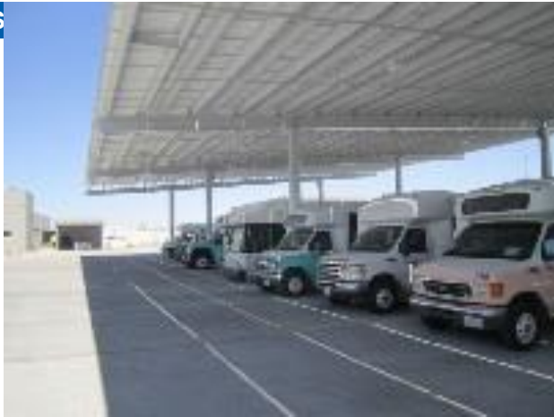
Photovoltaic shade structure
