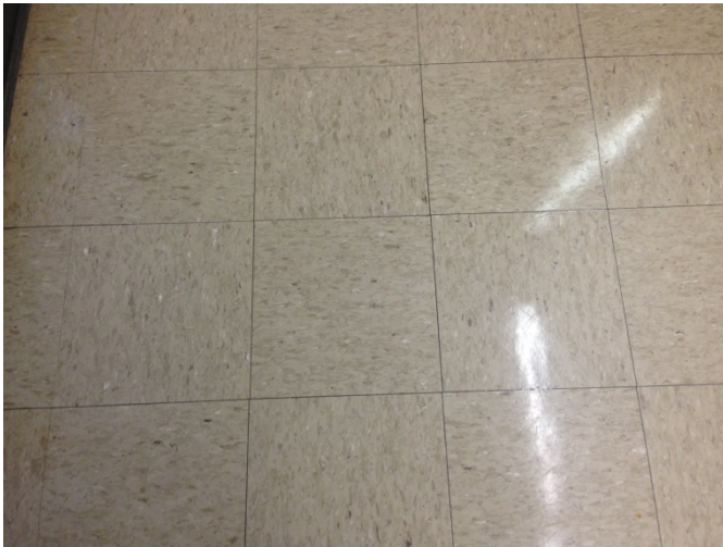
3. 12"X12" Brown Mottled Floor Tile & Associated Black Mastic - Stage
