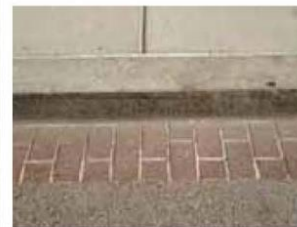
CONCRETE SIDEWALKS, GRANITE CURBS & BRICK GUTTER
