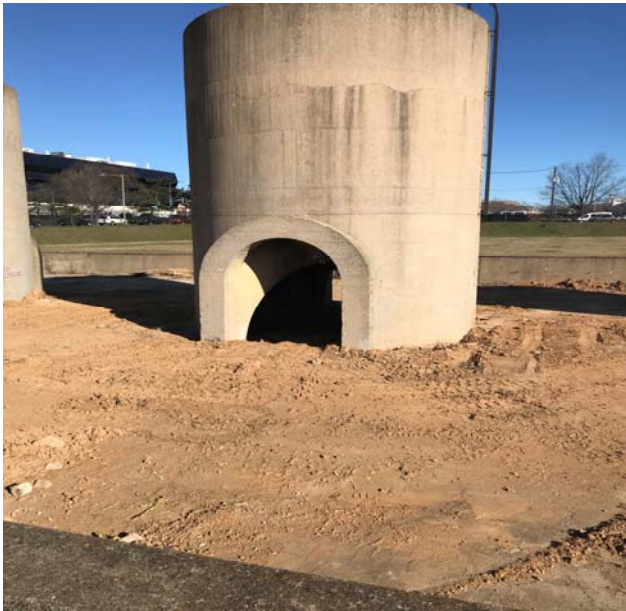
Exterior Backfill at Sand Bin after Grade Beam Pour
