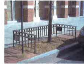
Note: 3" space between sides and bottom rail, tree box flush with grade and street sign outside of tree box. Ornamental O-rings are optional.
