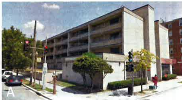
A View from intersection (Existing building to be demolished)
