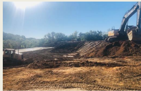
Excavation of unsuitable soils
