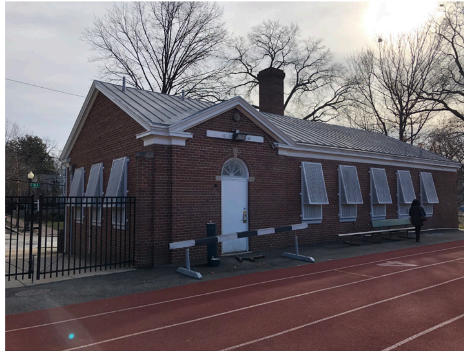
South Field House, Field-Side Facade
