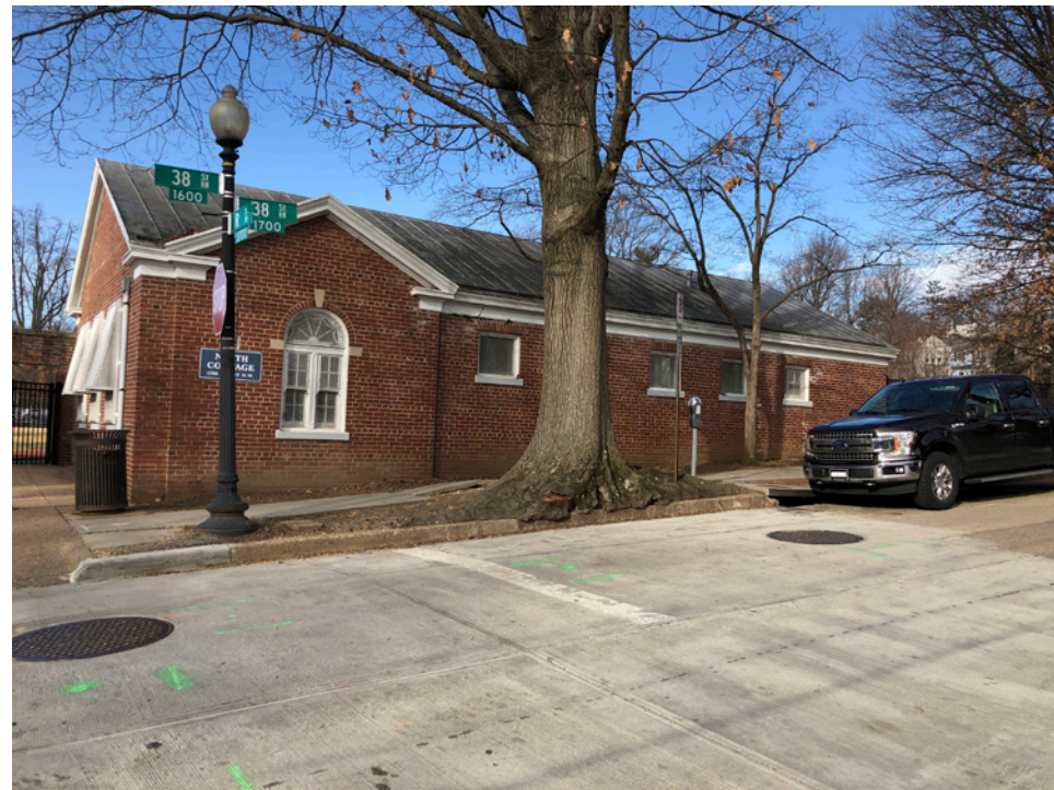
North Field House Street-Side Facade
