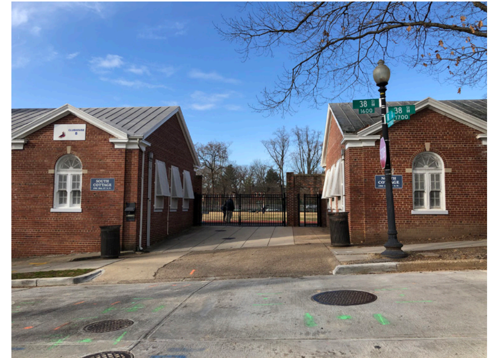
Main Entrance from 38th Street
