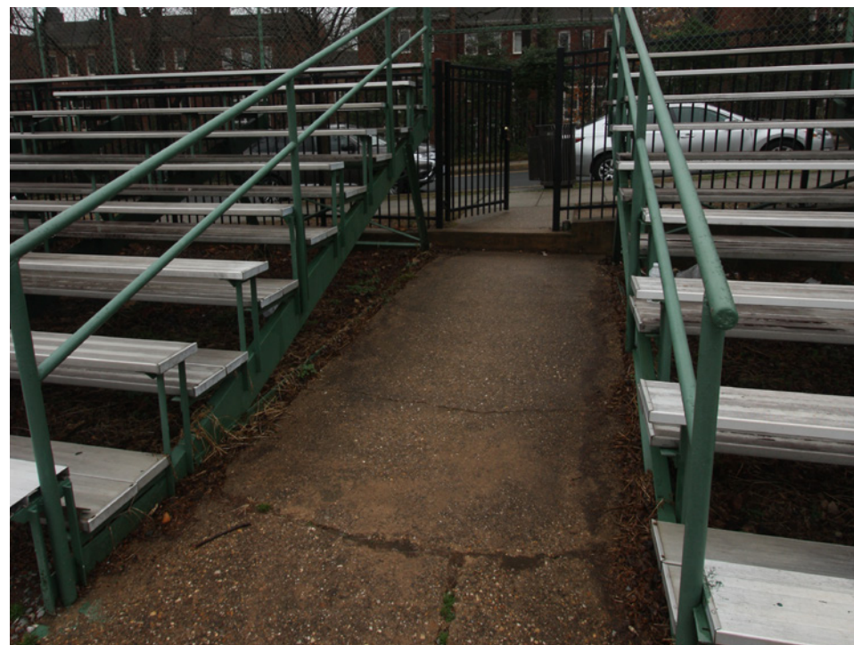
Secondary Entrance (Proposed Ramp)
