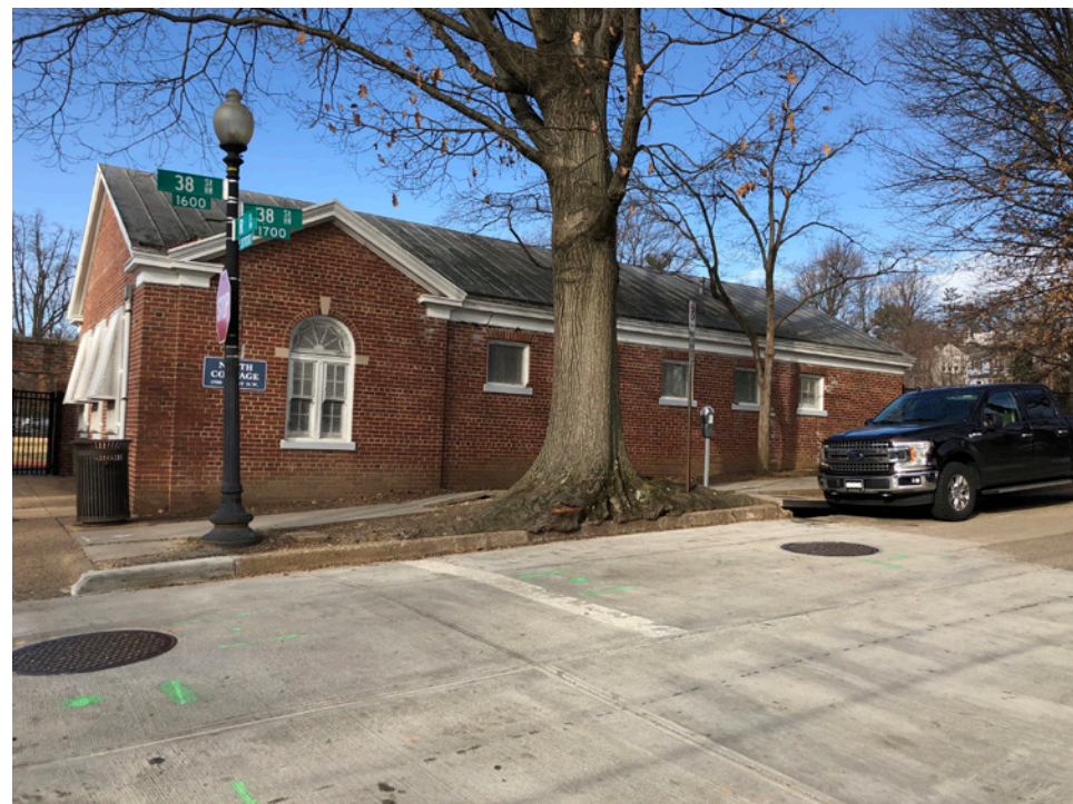
North Field House Street-Side Facade
