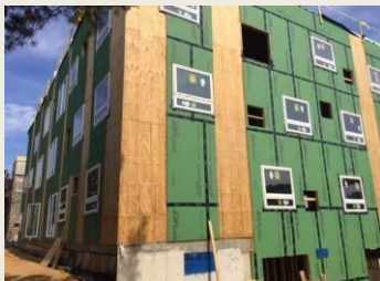
Zip System Install
