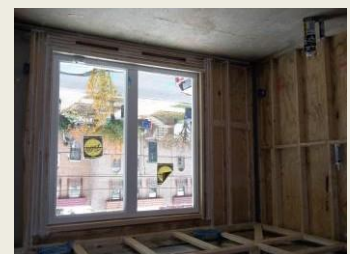
Framing and Window Install
