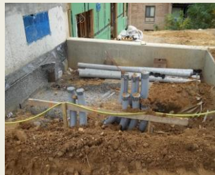
Pepco Duct Bank Install
