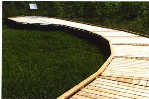
Raised Boardwalk to avoid roots
