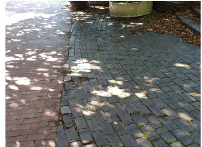
f. brick sidewalk to be repaired along Massachusetts Ave
