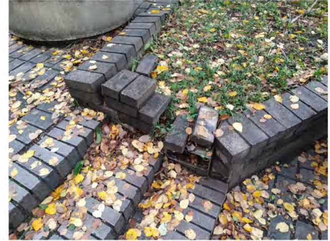
c. brick wall to be repaired
