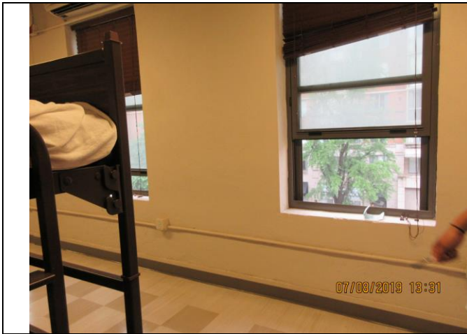
Description: windows left open.
