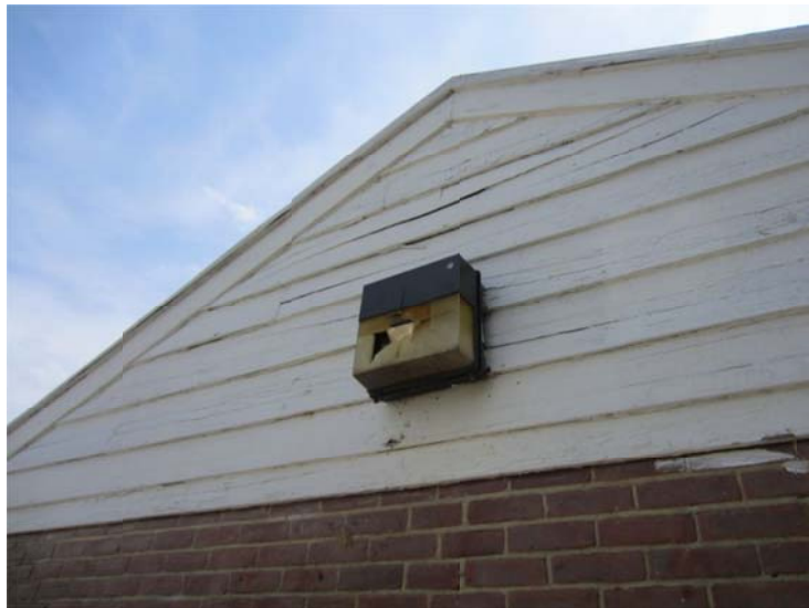
Photograph 4-8.20 (Field House) Water damage on floor in spec
