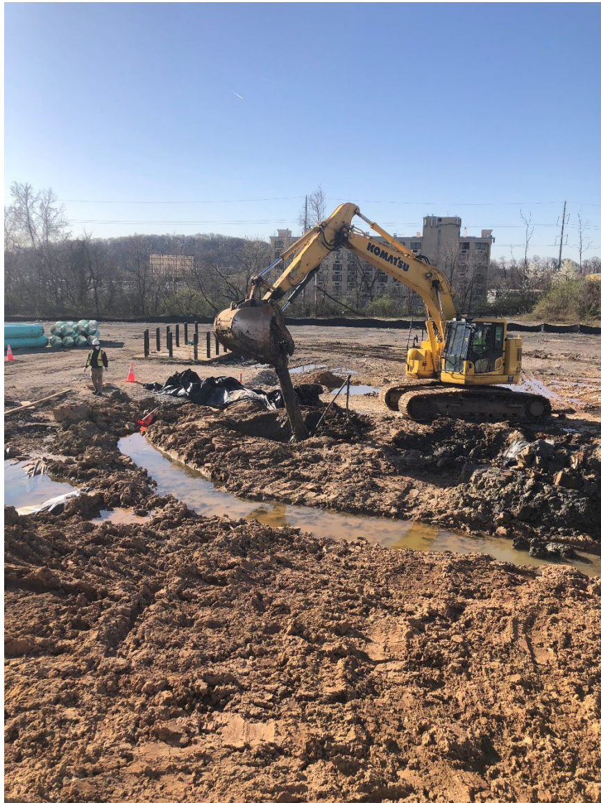
Photo of hydraulic lift area at beginning of removal and excavation
