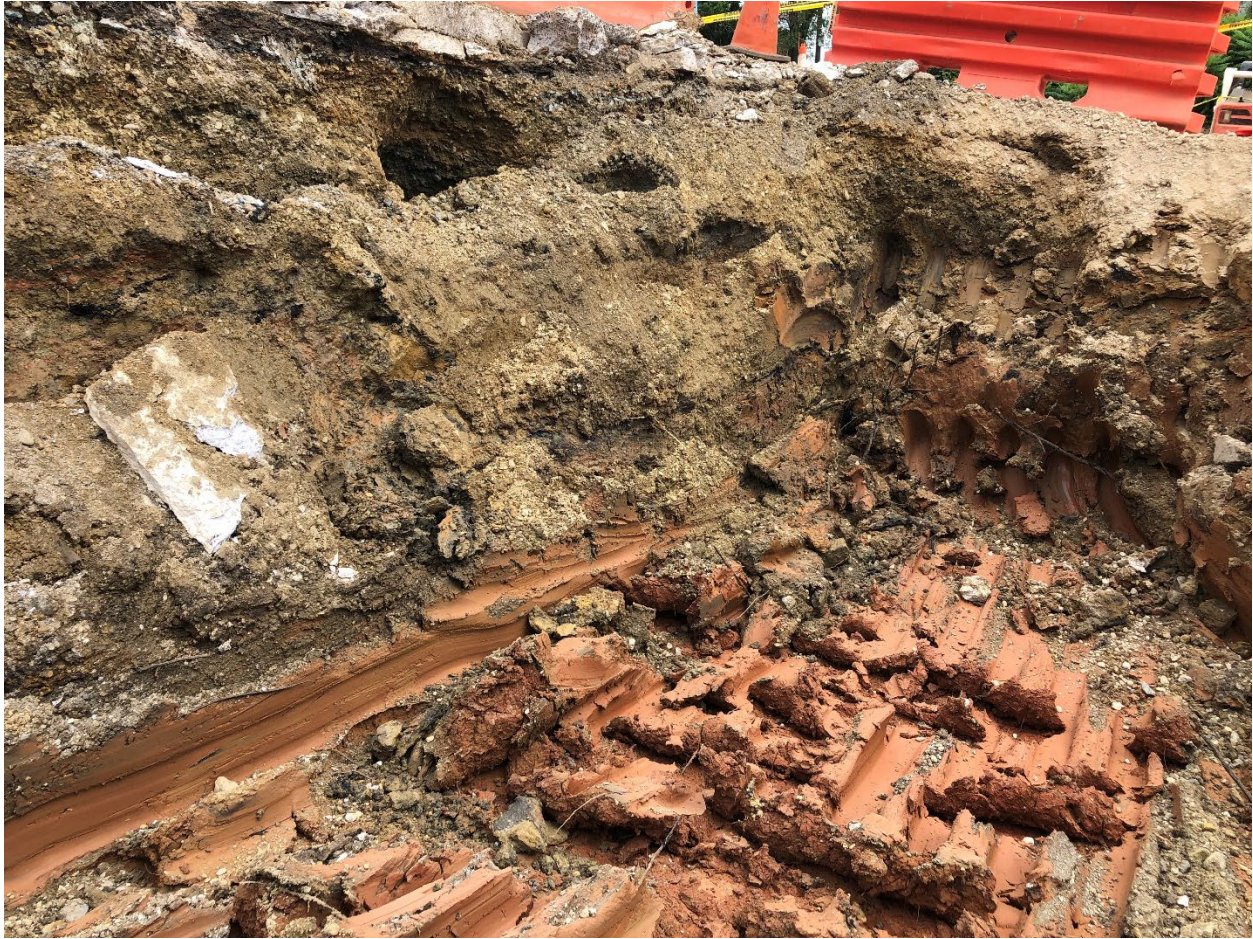
Photo of soil pit excavated down to the native clay substrate
