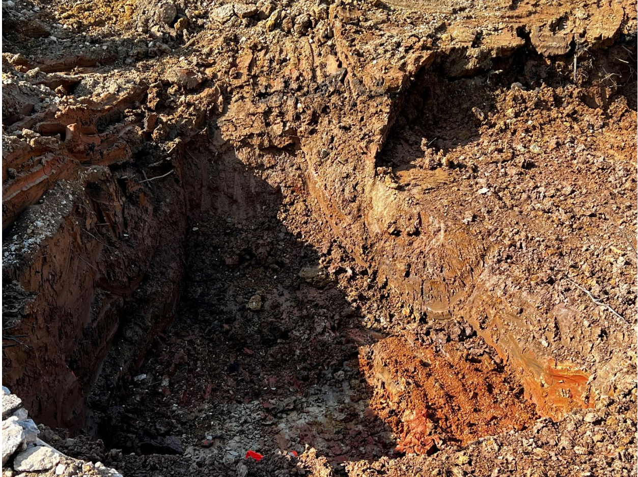
Partially excavated soil pit
