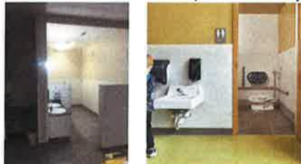
En-suite restrooms (accessible to one classrooms):
