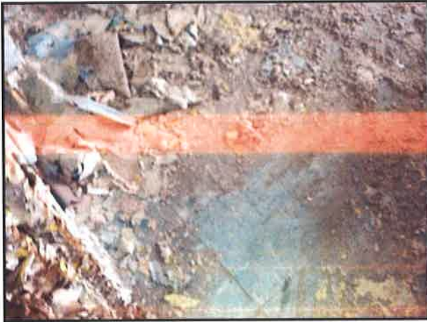
Photo 9: Green 9"x9" Floor tile with mastic (Close-up)
