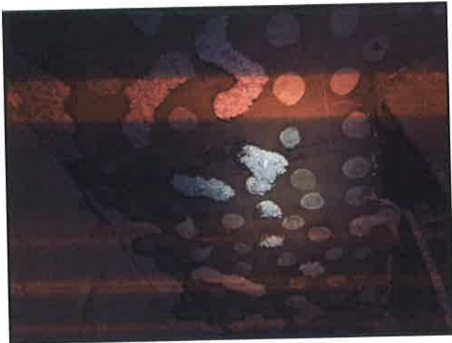
Photo 5: Glue Dots over the 1'x1' ceiling tile (Close-up)
