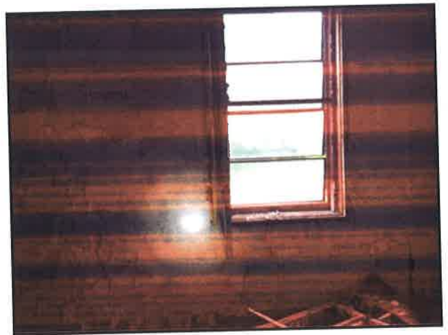
Photo 8: Gray Caulking on Windows (Wide angle)
