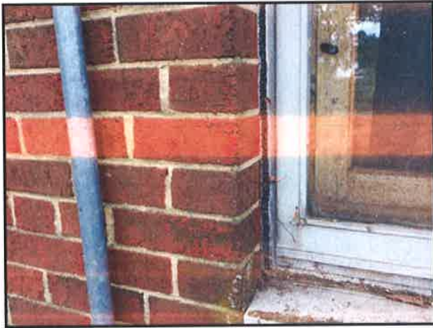
Photo 37: Gray Exterior window caulking (Close up)
