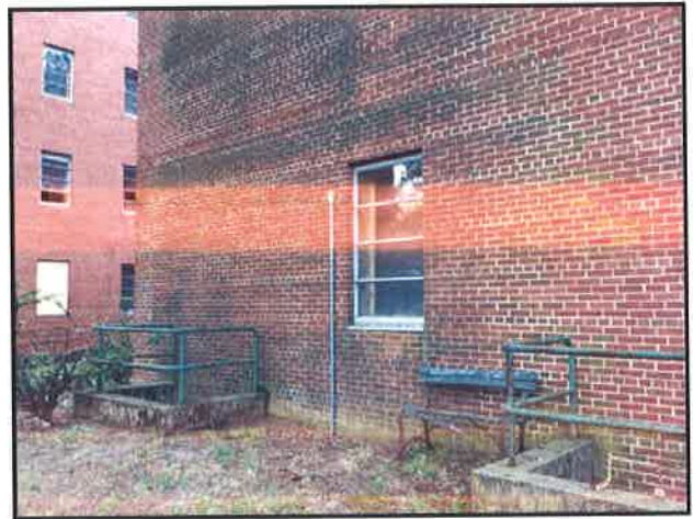
Photo 38: Gray Exterior window caulking (Wide angle)
