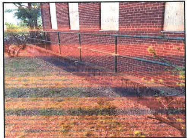
Photo 40: Black Exterior water proofing (Wide angle)
