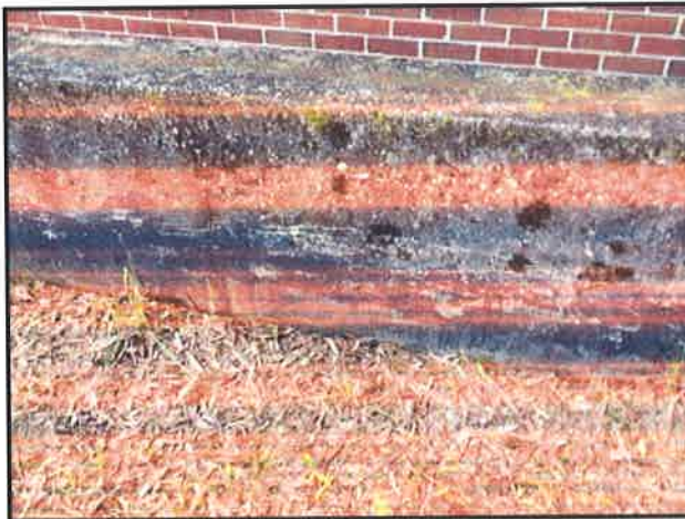
Photo 39: Black Exterior water proofing (Close up)
