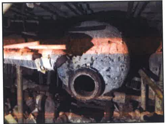
Photo 50: 12'x6' White tank insulation (Wide angle)
