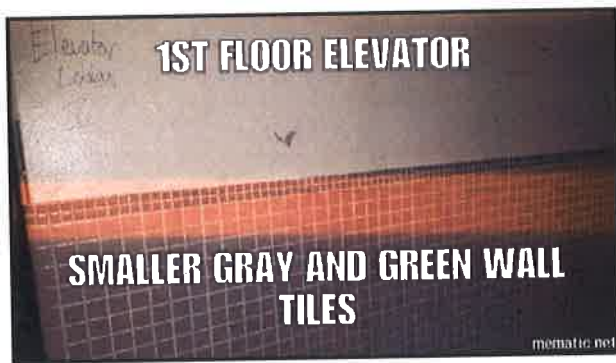
Photo 55: 1st floor, elevator lobby, ceramic wall tiles
