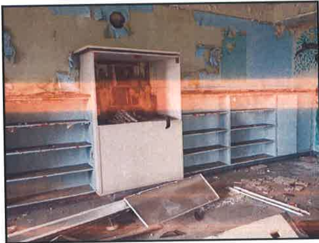
Photo 51: 4 th floor, room 413A, blue wooden shelves and cabinet
