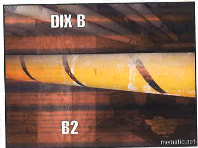
Photo 54: basement, yellow painted pipe
