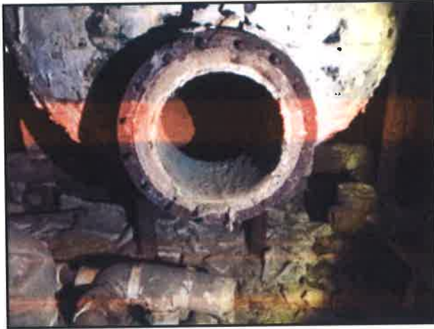
Photo 49: 12'x6' White tank insulation (Close up)
