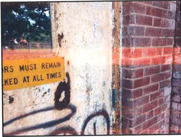
Photo 41: Gray Exterior door caulking (Close up)
