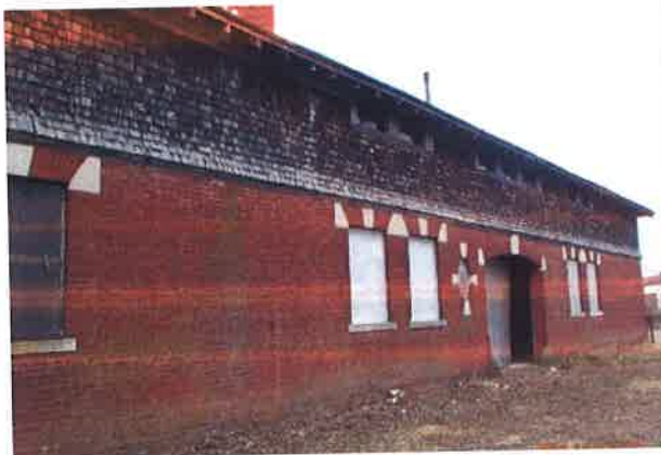
Photo 1 – Typical exterior wall – North Elevation
