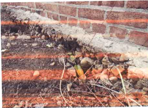
Photo 15 – Foundation work at the southeast corner
