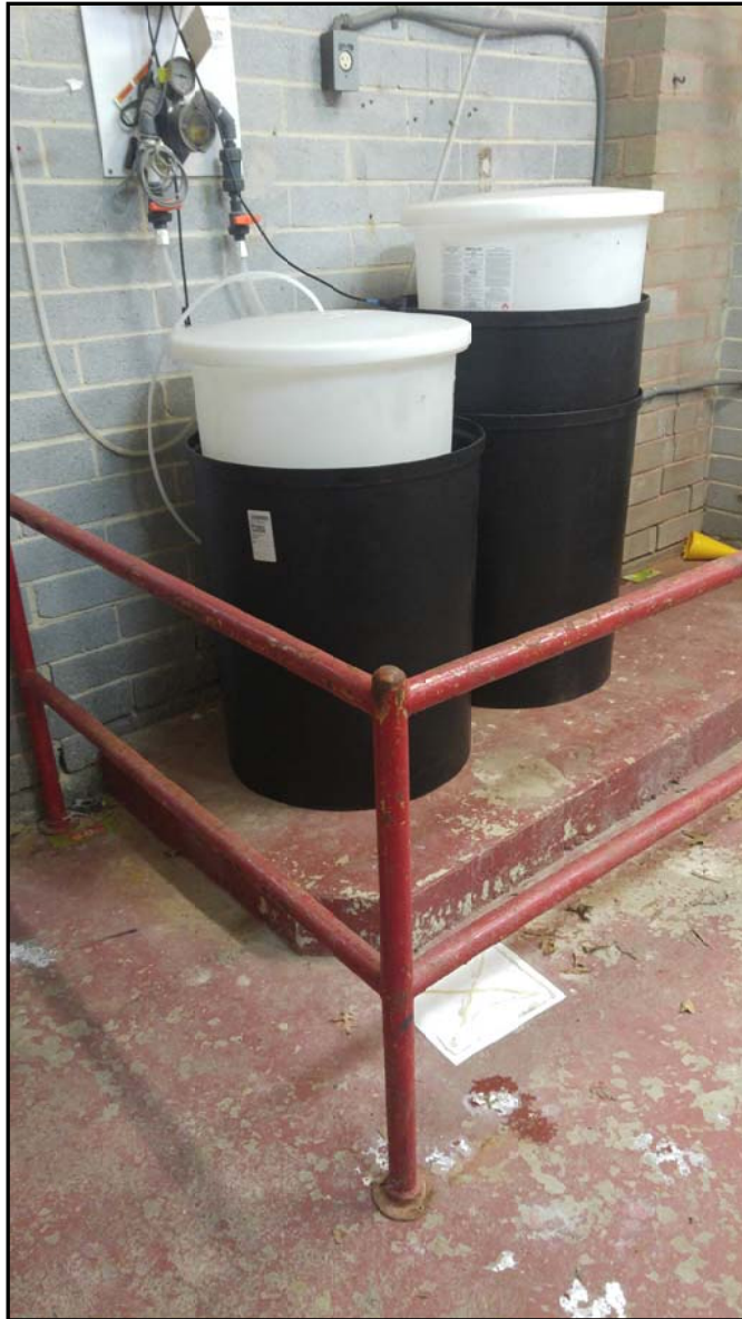
Lead-based paint railing and chemical storage within secondary containments
