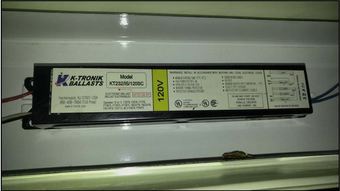
Non-PCB Containing ballast
