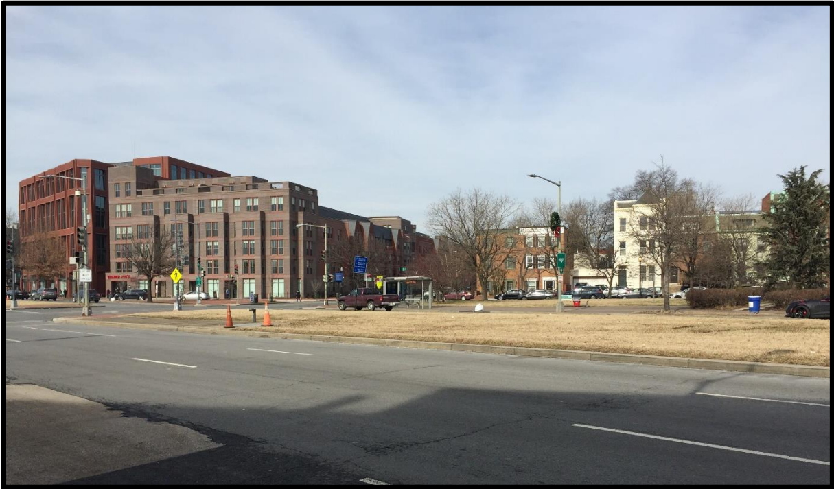
Figure 5. Intersection of Pennsylvania Avenue SE and 8 th Street SE in the approximate center of the Study Area, toward a recently-constructed commercial development. Facing northwest.
