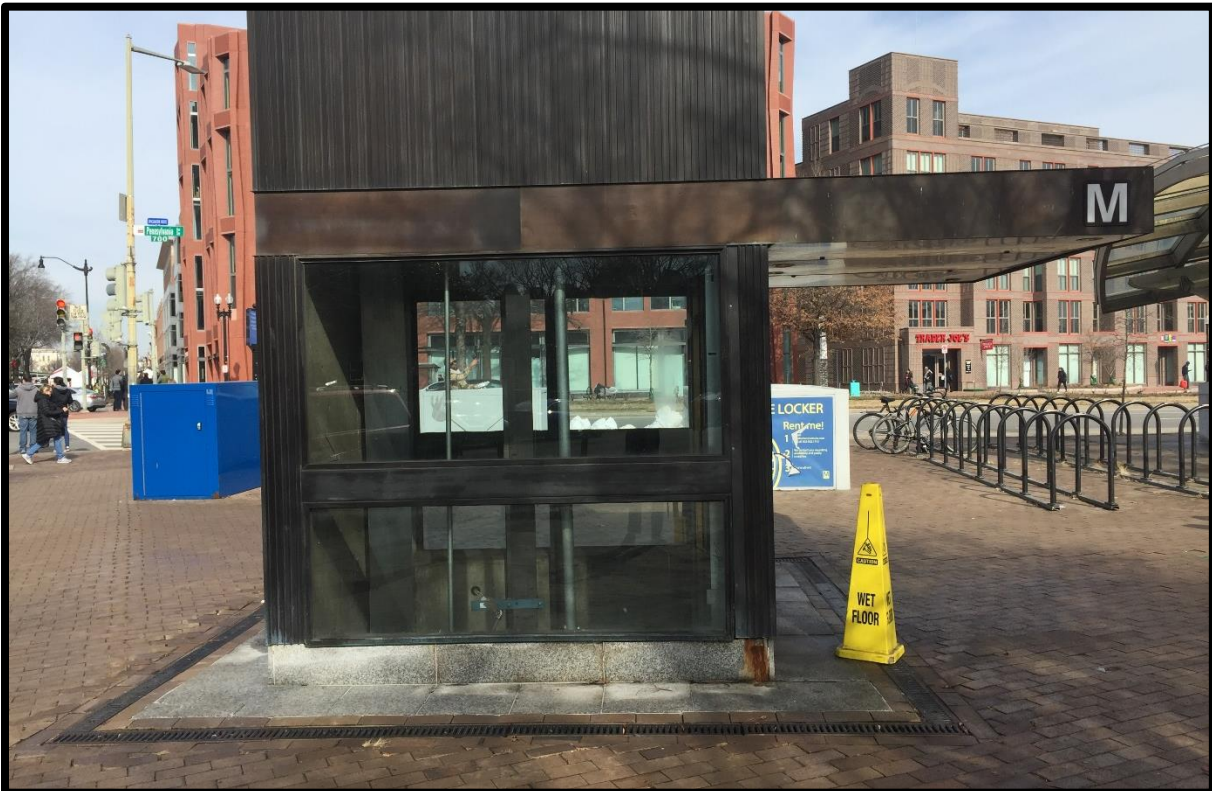
Figure 8. Eastern Market Metro Station, elevator entrance and surrounding brick walkway along 7 th Street SE. Facing north.
