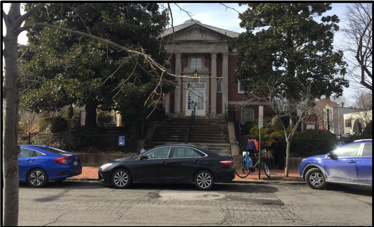
Figure 6. East façade of the Southeast Neighborhood Library across 7 th Street SE. Facing west.
