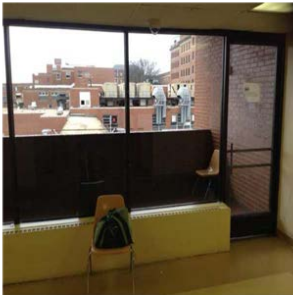
Aluminum Storefront At Patio Area
