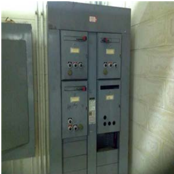
Distribution Panel Board :- Rooftop Penthouse Air Handler Distribution Panel
