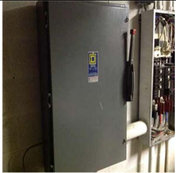
Disconnect Switch, 400 Amp:- Basement Level Electrical Disconnect Switch
