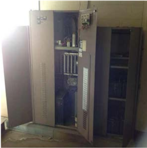
Rooftop Penthouse UPS
