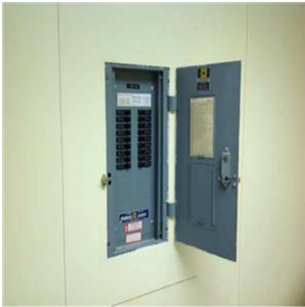
Circuit Breaker, 3 Ph., 600 V, 100 Amp :- Common Hallway 100 Amp Circuit Breaker Panel
