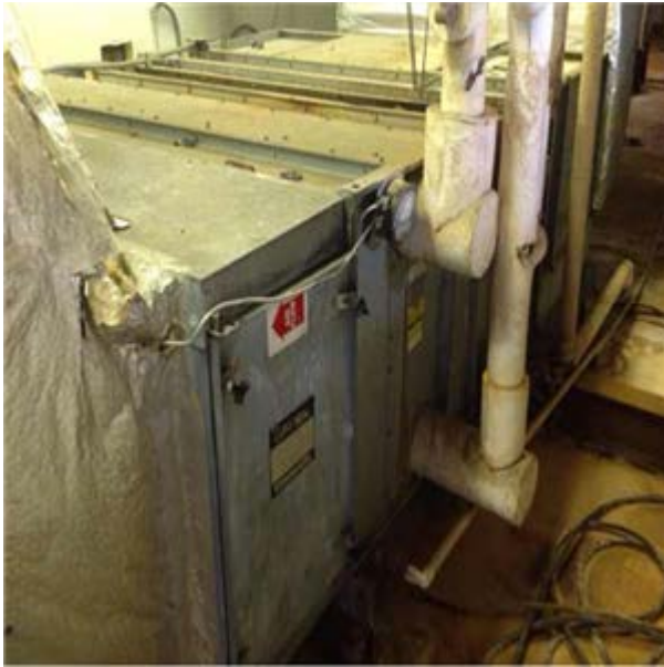
Carrier Rooftop Penthouse Air Handler
