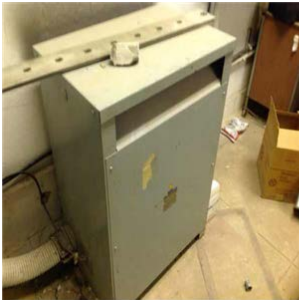
Secondary Transformer, Dry, 75 kVA :- Basement Electric Room Secondary Transformer
