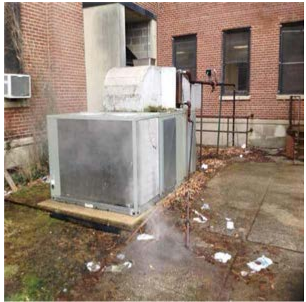
Air Conditioner Multizone Variable Volume 25 Ton:- Pad Mounted Trane Package Unit
