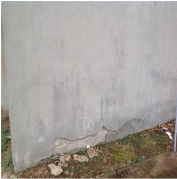
Exterior Wall Stucco Finish
