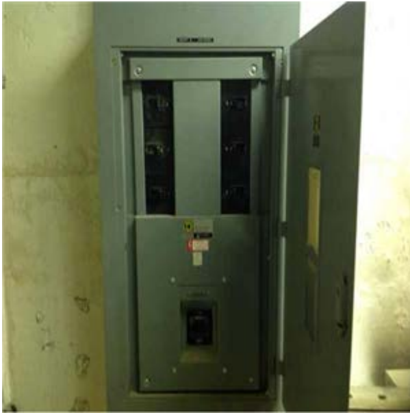
400 Amp Circuit Breaker Panel
