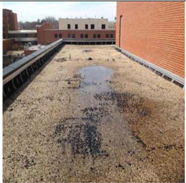
Built-up Roof:- Low Slope Built Up Asphalt Roof
