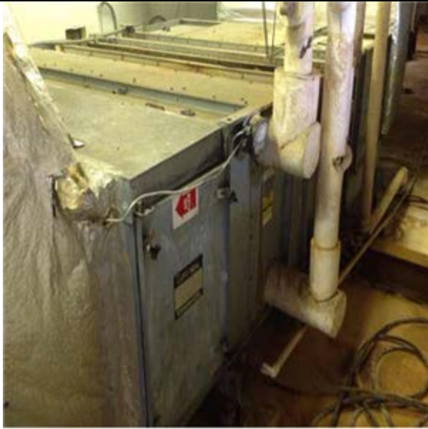
Air Handler, Multizone, 65,000 Cfm :- Carrier Rooftop Penthouse Air Handler
