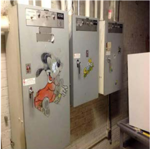
Generator Transfer Switch
