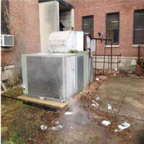
Pad Mounted Trane Package Unit
