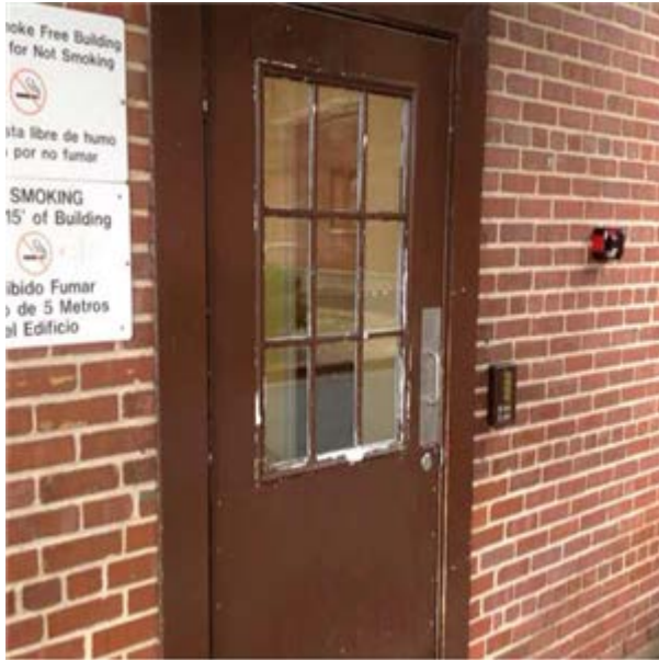
Exterior Painted Metal Door
