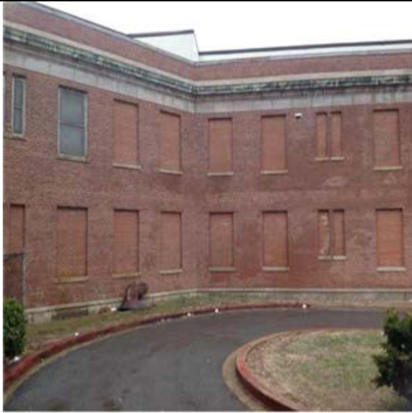
Clay Brick, Exterior, = 3 Stories :- Exterior Wall Clay Brick
