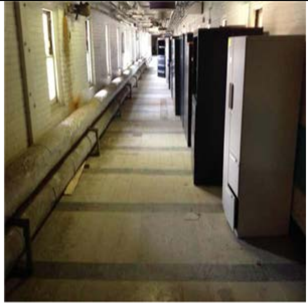
Abandoned Basement Level
