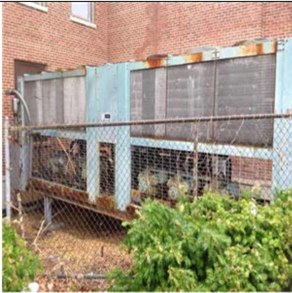
Air Conditioner Multizone Variable Volume 50 Ton :- Carrier Pad Mounted Packaged Unit
