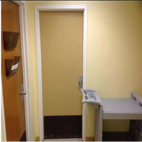
Steel, Painted, Interior Door :- Interior Painted Steel Door
