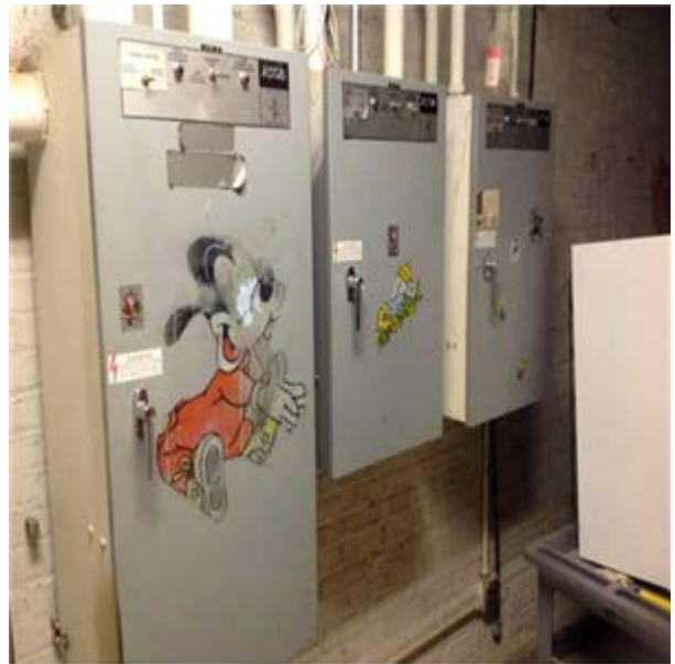
Transfer Switch, Auto, 600 V, 1,200 Amp:- Generator Transfer Switch
