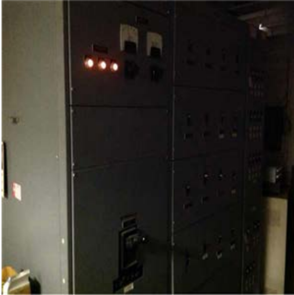
Basement Level Main Electric Disconnect
