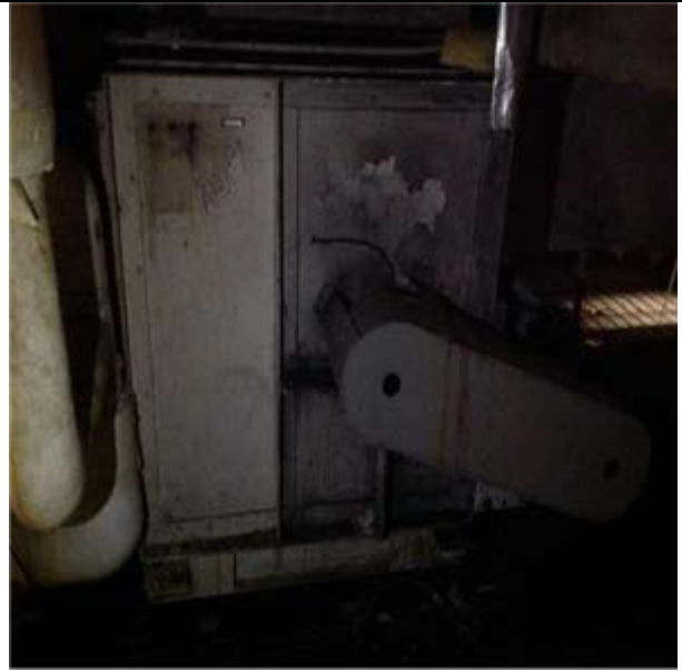
Air Handler, Multizone, 65,000 Cfm:- Basement Level Air Handler
