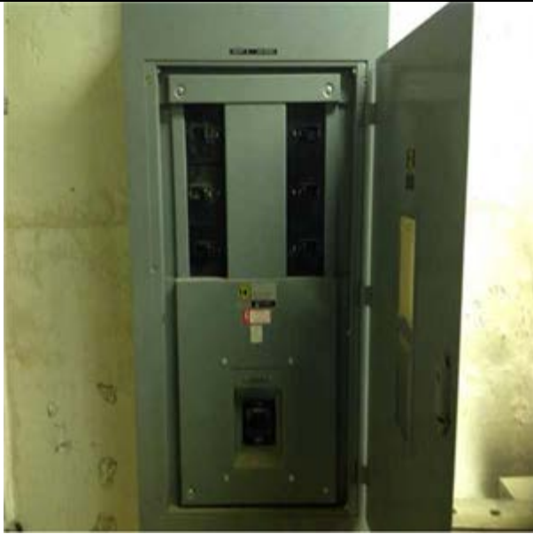
Circuit Breaker, Main, 208 Y, 120 V, 400 Amp :- 400 Amp Circuit Breaker Panel
