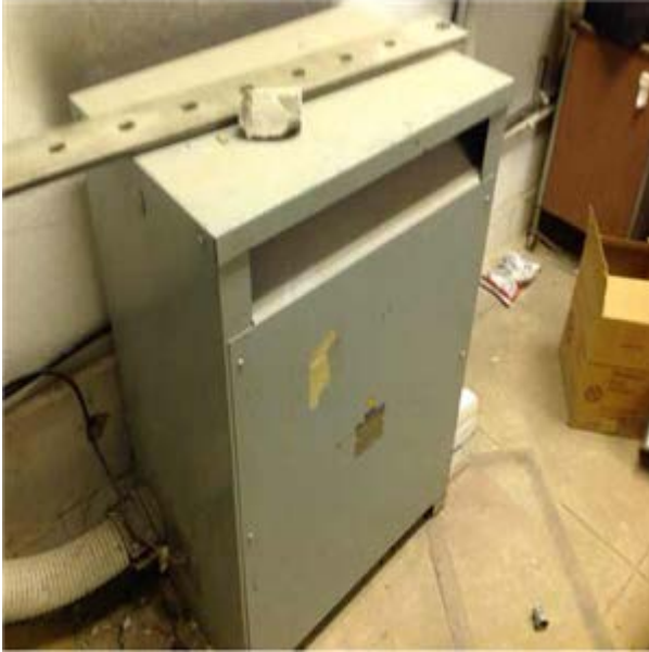
Basement Electric Room Secondary Transformer
