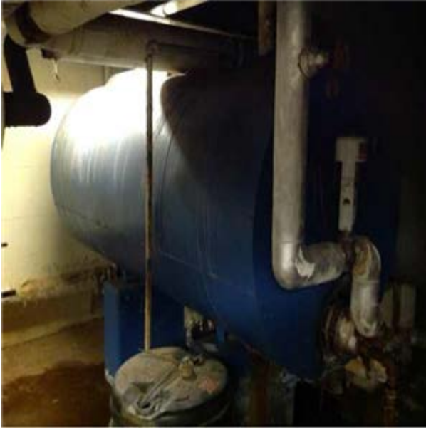
Domestic Hot Water Storage Tank
