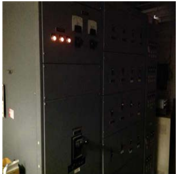
Main Switchgear, 208 Y, 120 V, 2,000 Amp:- Basement Level Main Electric Disconnect
