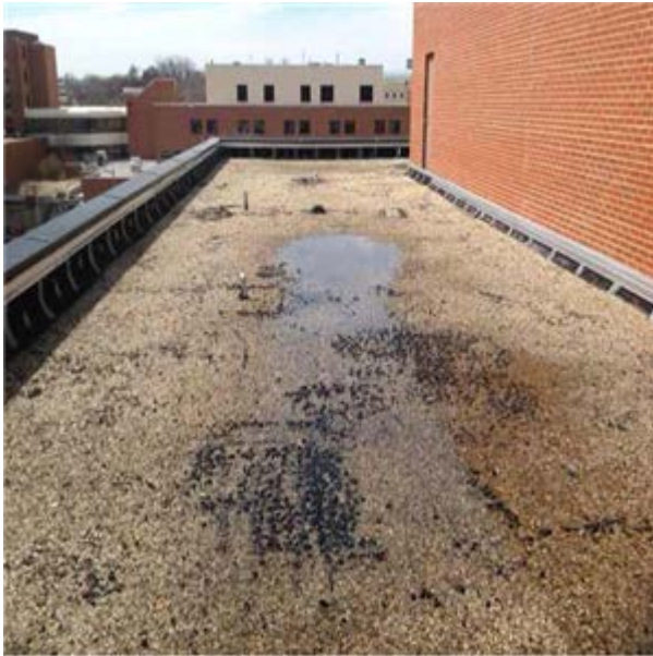
Low Slope Built Up Asphalt Roof
