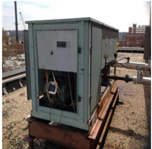
Chiller, Absorption, 30 Ton:- RooftopChiller
