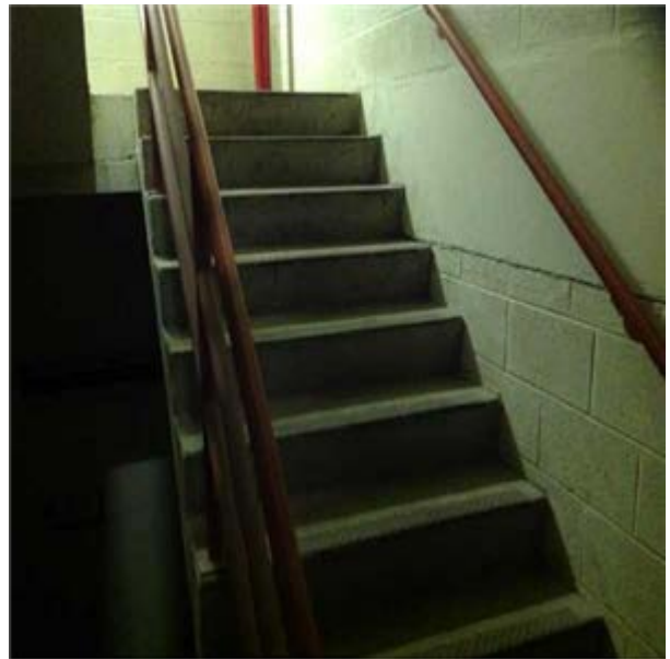
Concrete, Interior Stairs:- Concrete Interior Stair
