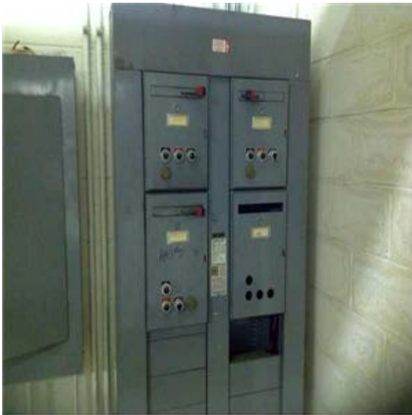
Rooftop Penthouse Air Handler Distribution Panel
