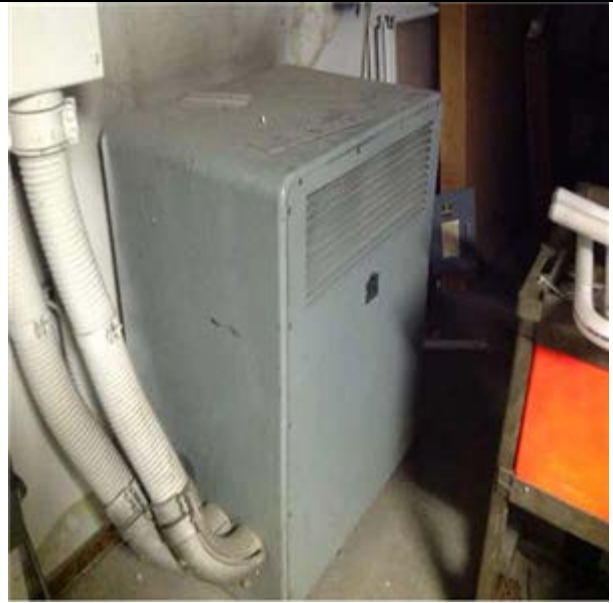
Secondary Transformer, Dry, 300 kVA:- Basement Level Electric Secondary Transformer
