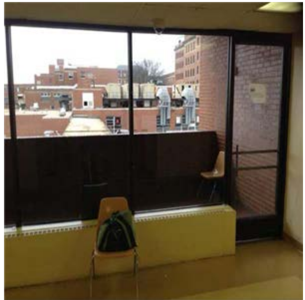
Storefronts:- Aluminum Storefront At Patio Area
