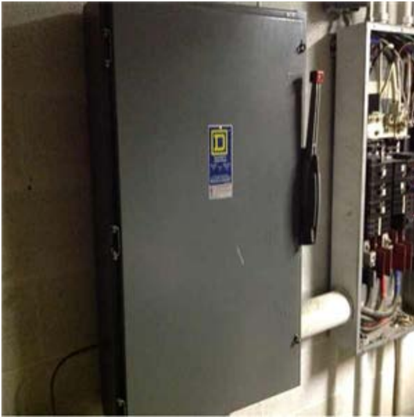
Basement Level Electrical Disconnect Switch
