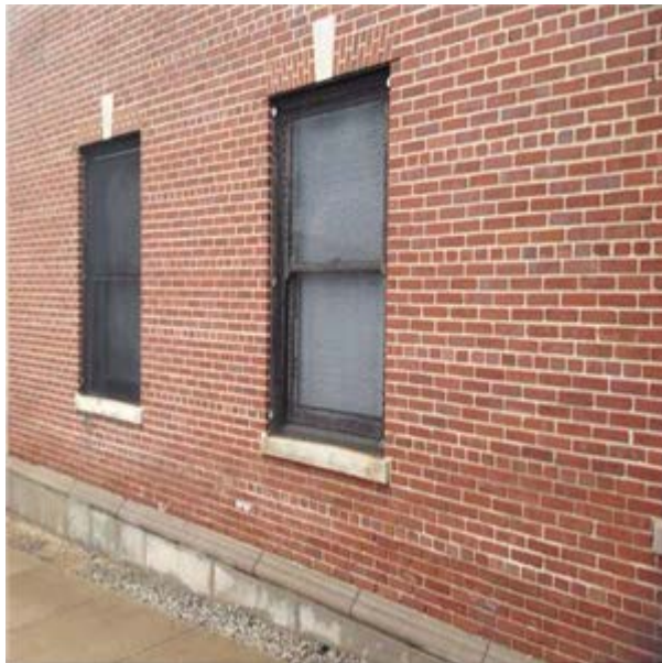
Operable Wood Windows
