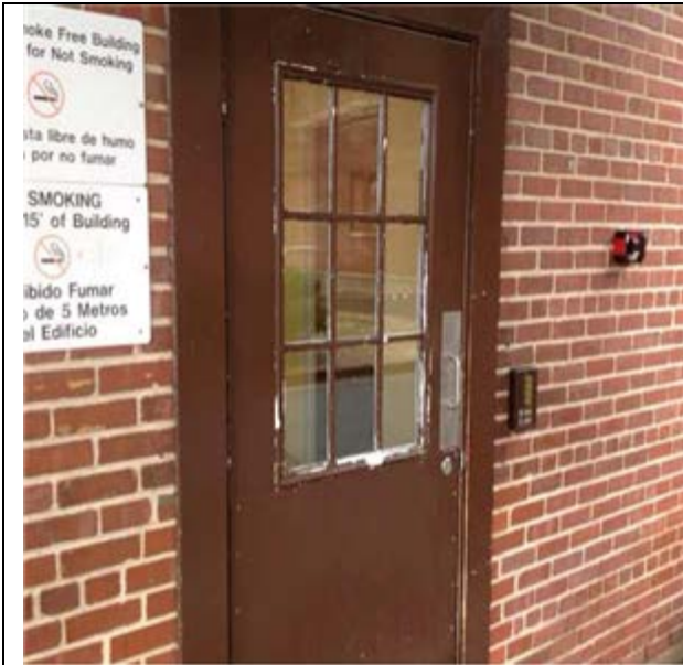
Steel, Painted, Exterior Door :- Exterior Painted Metal Door
