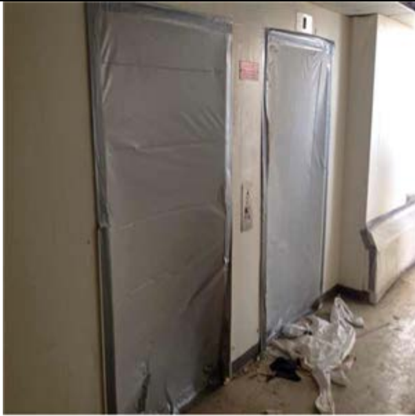
Abandoned Passenger Elevators
