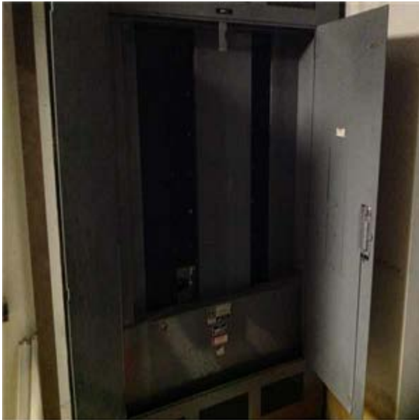
Basement Electric 1200 Amp Circuit Breaker Panel
