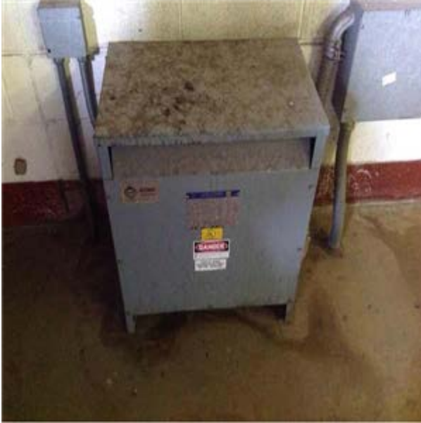
Rooftop Penthouse Transformer
