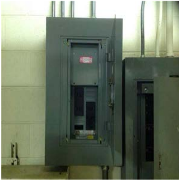
Rooftop Penthouse Circuit Breaker Panel
