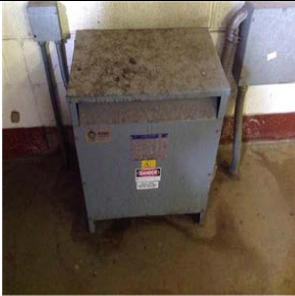
Secondary Transformer, Dry, 30 kVA :- Rooftop Penthouse Transformer
