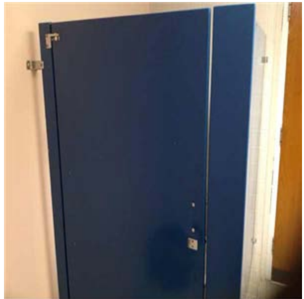
Site Built Toilet Partitions:- Bathroom Toilet Partion
