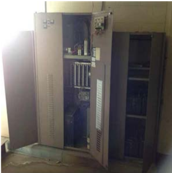
Uninterruptible Power Supply, 80 kVA :- Rooftop Penthouse UPS
