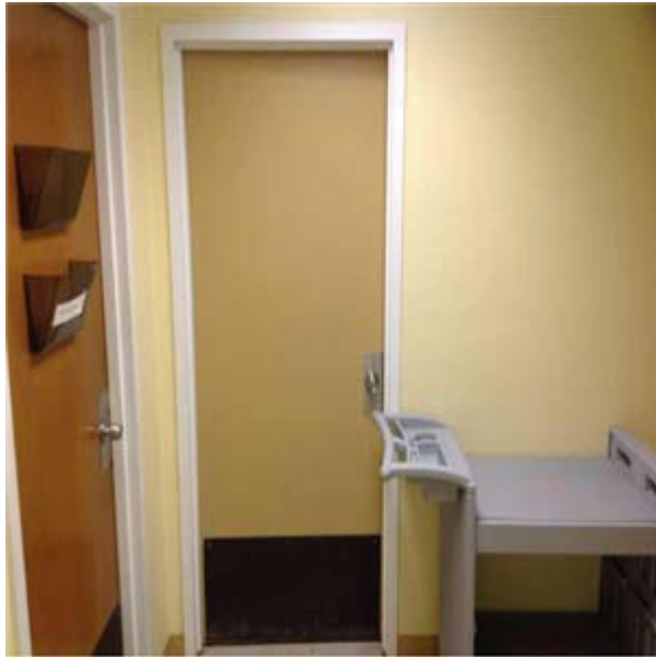
Interior Painted Steel Door
