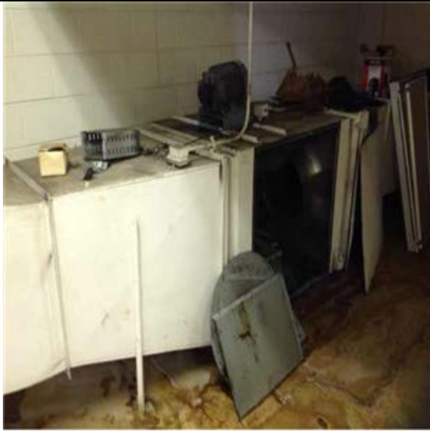
Abandoned Rooftop Penthouse Air Handler
