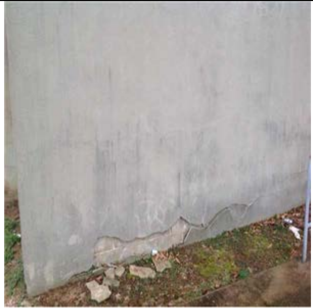
Stucco, Painted, Exterior, 2 Stories:- Exterior Wall Stucco Finish
