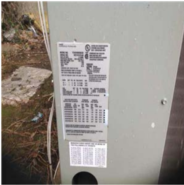
Air Conditioner Multizone Variable Volume 25 Ton :- Pad Mounted Trane Package Unit Nameplate
