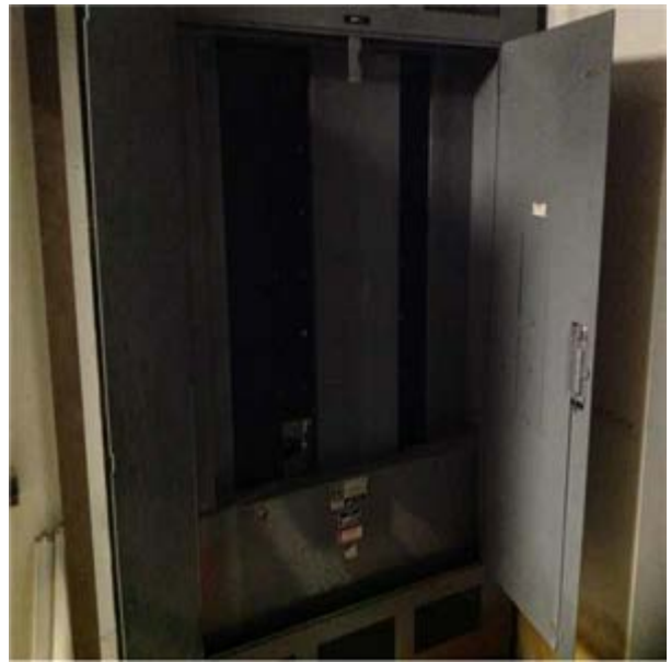
Circuit Breaker, Main, 208 Y, 120 V, 1,200 Amp:- Basement Electric 1200 Amp Circuit Breaker Panel
