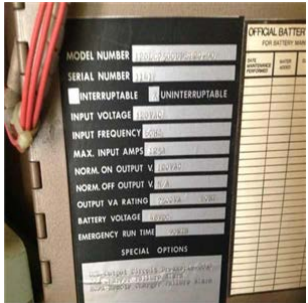
Uninterruptible Power Supply, 80 kVA:- UPS Nameplate
