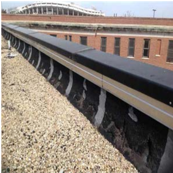
Built-up Roof :- Roof Parapet Flashings
