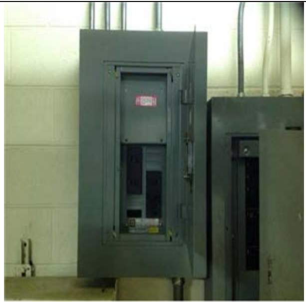
Circuit Breaker, 3 Ph., 600 V, 100 Amp:- Rooftop Penthouse Circuit Breaker Panel
