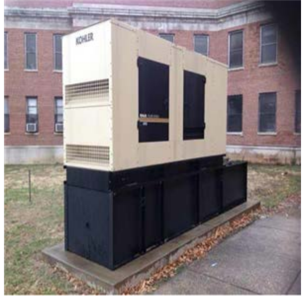
Generator, Diesel, 375 kW:- Kohler Pad Mounted Generator
