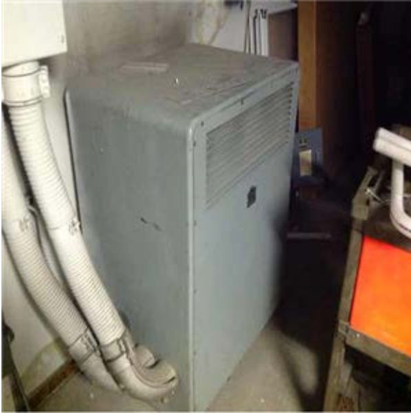
Basement Level Electric Secondary Transformer
