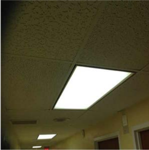
Recessed Ceiling Mounted Fluorescent Light Fixture
