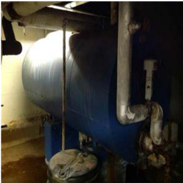
2000 Gallon Domestic Hot Water tank :- Domestic Hot Water Storage Tank
