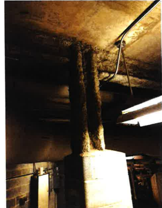
CONCRETE PLANKS ON STEEL COLUMNS & BEAMS
