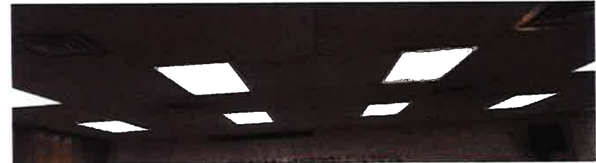
MULTIPURPOSE ROOM LIGHTING
