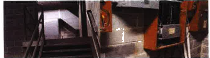
STAIRS TO ELECTRICAL ROOM
