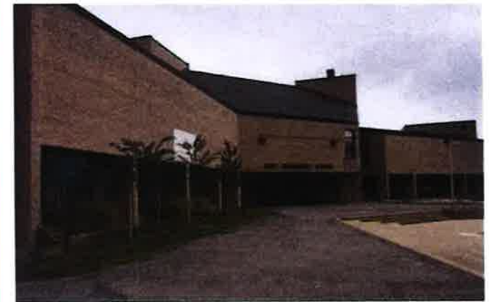
VIEW TOWARDS MAIN ENTRANCE
