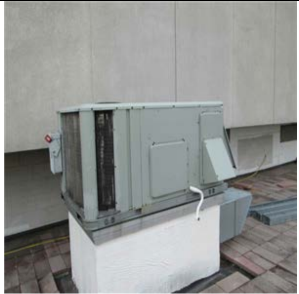
Air Conditioner, Rooftop, Multizone, 3 Ton:- Rooftop packaged unit
