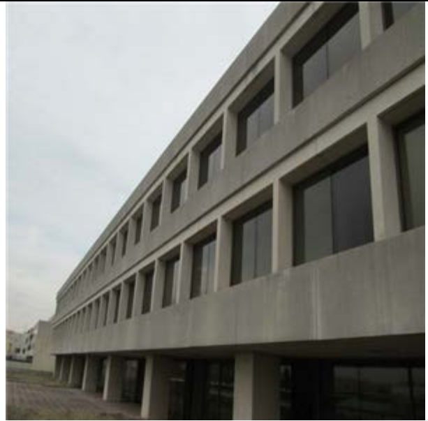
Alum Fixed Therm Break, Dbl Glaz, Gas 3 Story 24SF:- Exterior fixed windows
