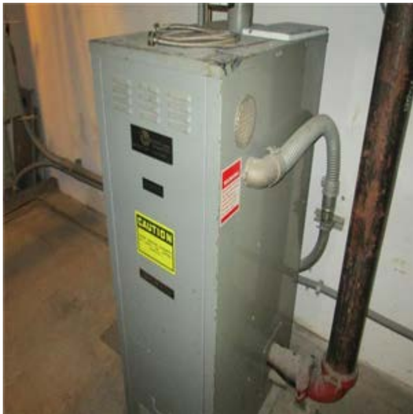
Boiler, Electric, 100 kW :- Electric boiler
