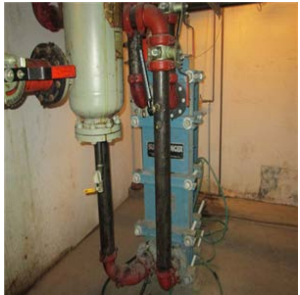
Heat Exchanger, Water-to-Water, 40 Gpm:- Plate heat exchanger
