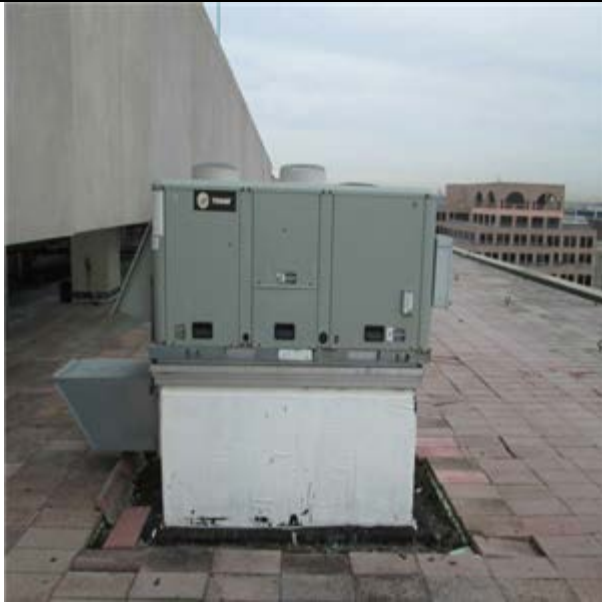
Air Conditioner, Rooftop, Multizone, 3 Ton :- Packaged RTU
