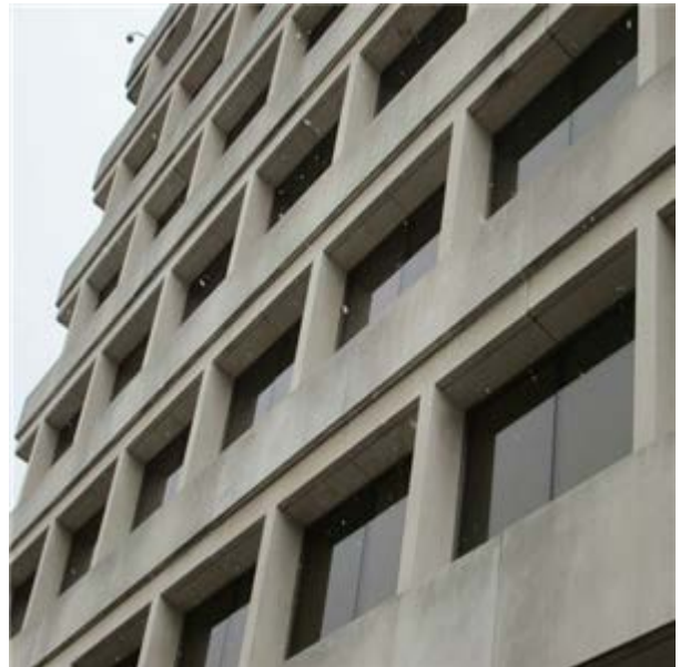
Concrete, Exterior, = 3 Stories:- Exterior wall
