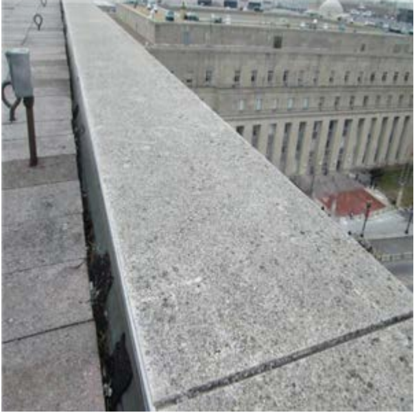
Stone roof coping
