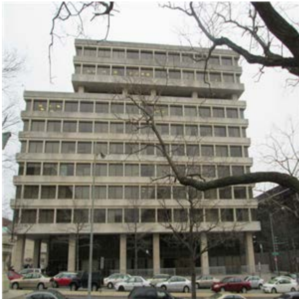
Concrete, Exterior, = 3 Stories :- Exterior wall
