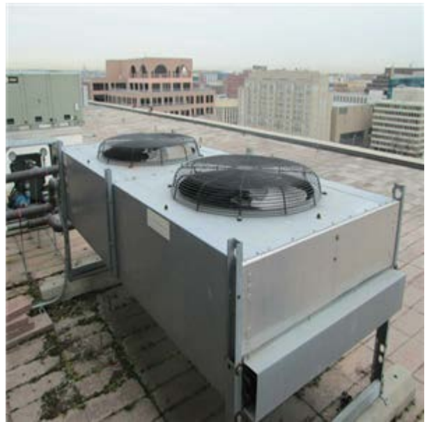
Condenser, Dry-Cooled, 10 Ton:- Dry cooler
