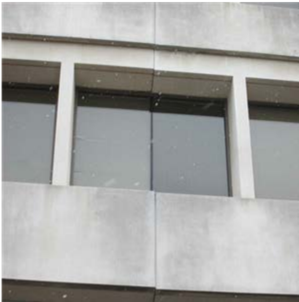
Fixed exterior window
