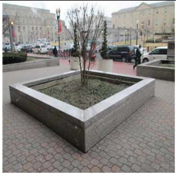
Paving & Surfacing:- Stone pavers
