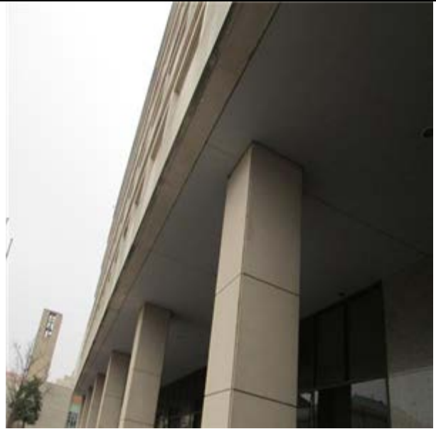
Concrete Frame Structure:- Concrete column
