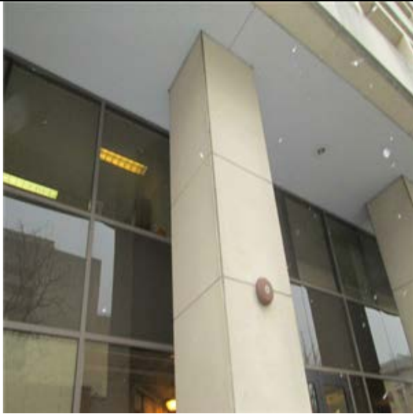
Concrete Frame Structure :- Concrete column
