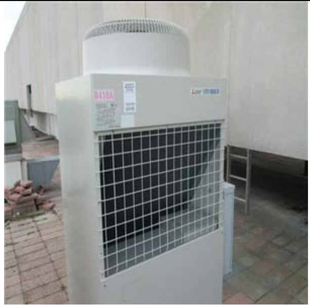
Condenser, Air-Cooled, 10 Ton:- Condensing unit
