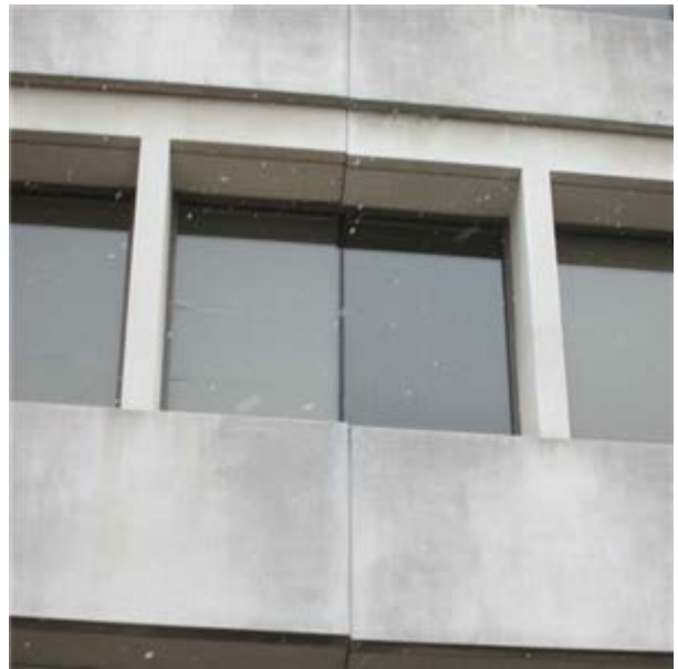
Alum Fixed Therm Break, Dbl Glaz, Gas 3 Stry, 12SF:- Fixed exterior window
