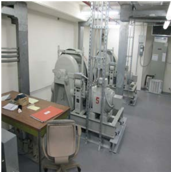
Elevator, Geared, 3-5 Floor, 3,000 Lbs, 300 fpm :- Elevator equipment
