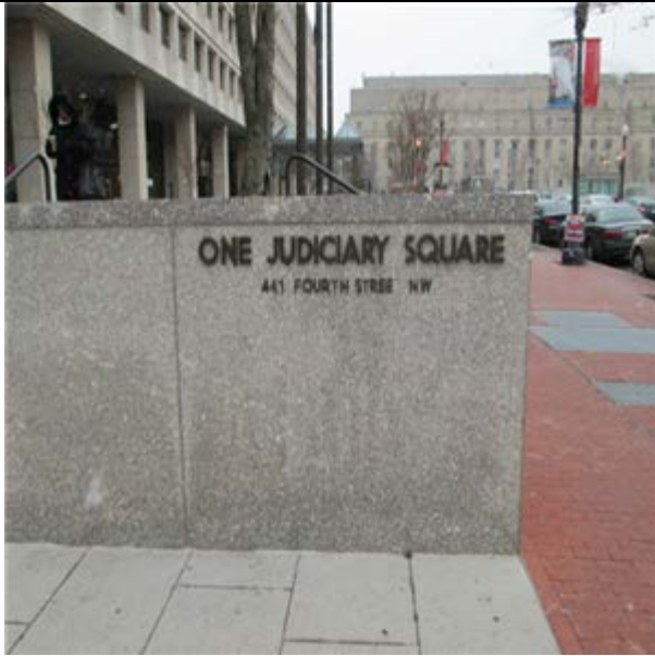
Paving & Surfacing :- Brick pavers
