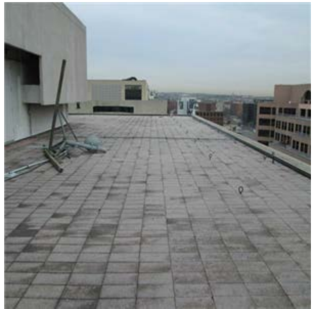
Single-Ply Modified Bituminous/Thermoplastic Roof:- Roof overview
