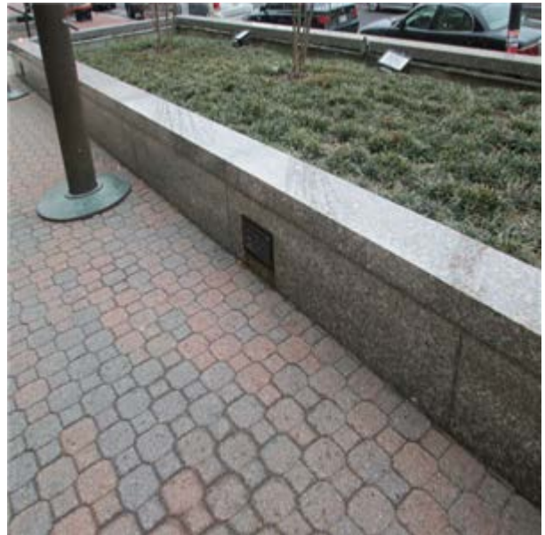
Paving & Surfacing:- Stone pavers
