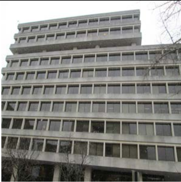
Concrete, Exterior, = 3 Stories :- Exterior Wall
