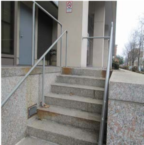
Exterior Steps :- Exterior stairs
