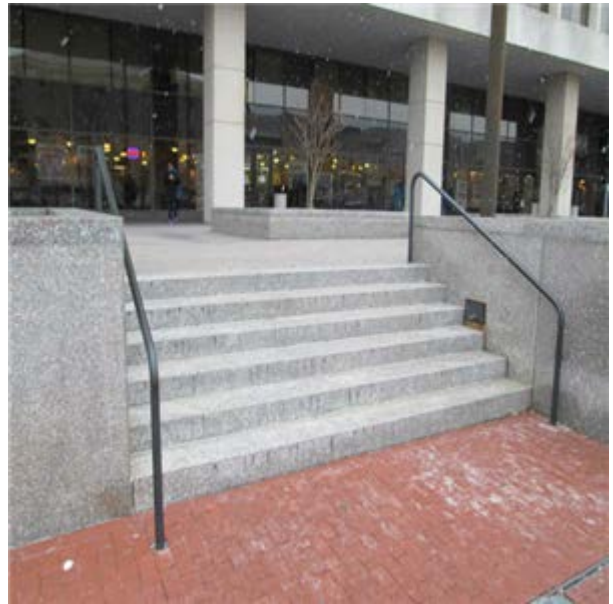
Exterior Steps:- Exterior stairs
