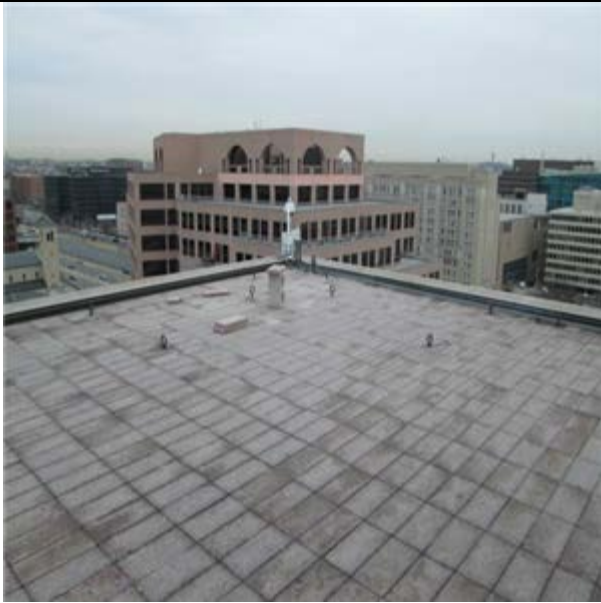
Single-Ply Modified Bituminous/Thermoplastic Roof :- Roof
