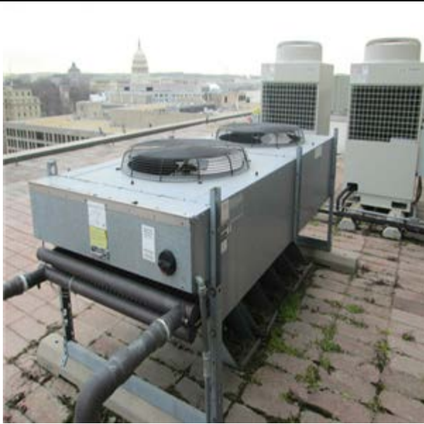
Condenser, Dry-Cooled, 10 Ton :- Dry cooler
