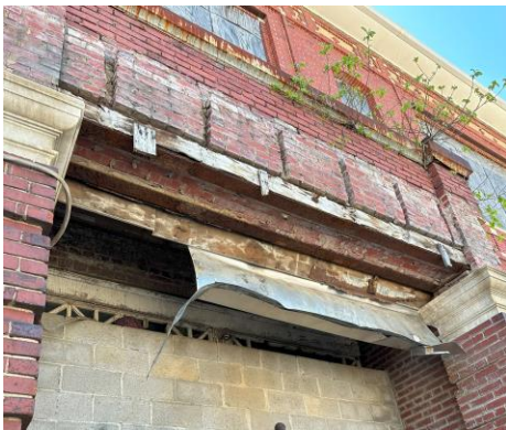
Figure 3: Lintels supporting brick over northern entrance
