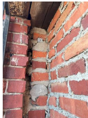
Figure 4: Temporary repair/infills
