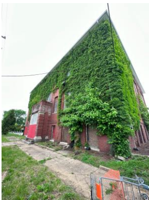
Figure 5: View of building from SE
