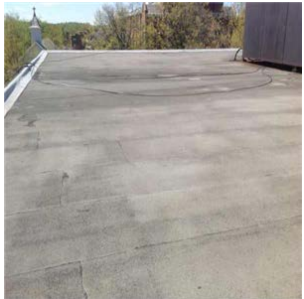
Built-up Roof:- (null)
