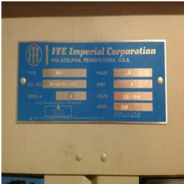
Power Panel Board, 208 Y, 120 V, 125 Amp :- (null)
