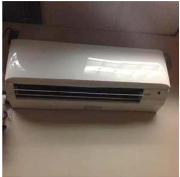
Indoor Unit Only - Cooling, Heating Coils and Circulation Fan:- mini split indoor unit
