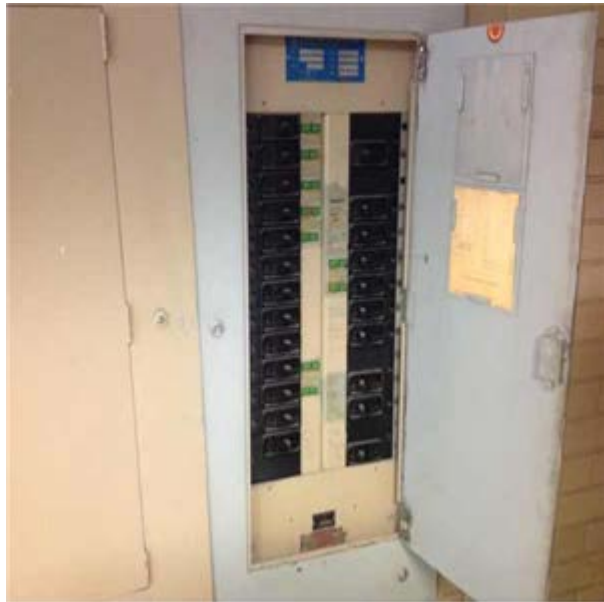
Power Panel Board, 208 Y, 120 V, 225 Amp :- (null)
