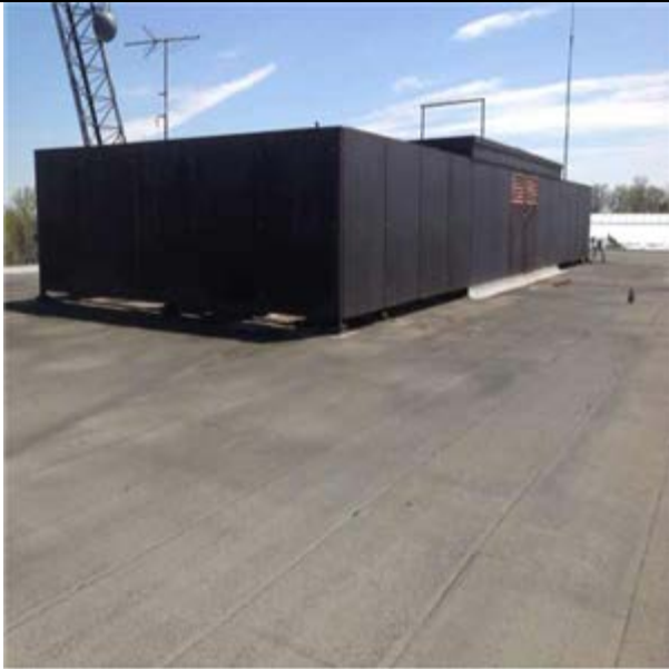
Built-up Roof :- (null)
