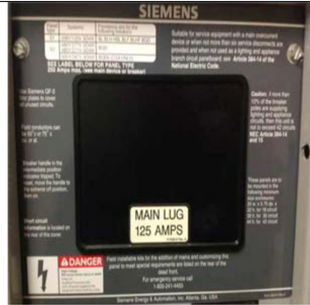
Power Panel Board, 208 Y, 120 V, 125 Amp :- (null)
