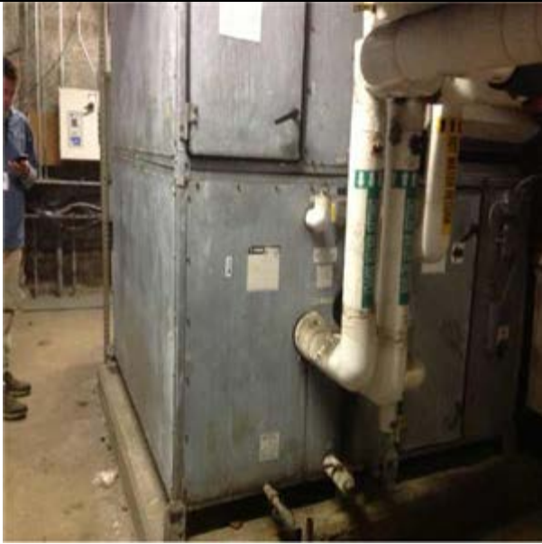
Air Handler, Multizone, 20,000 Cfm :- ahu-1
