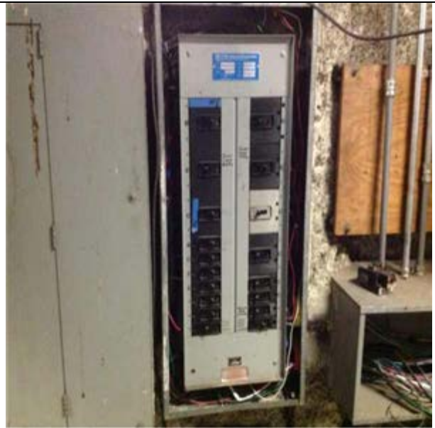
Power Panel Board, 208 Y, 120 V, 125 Amp:- in penthouse
