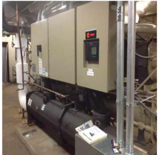
Chiller, Absorption, 50 Ton:- (null)
