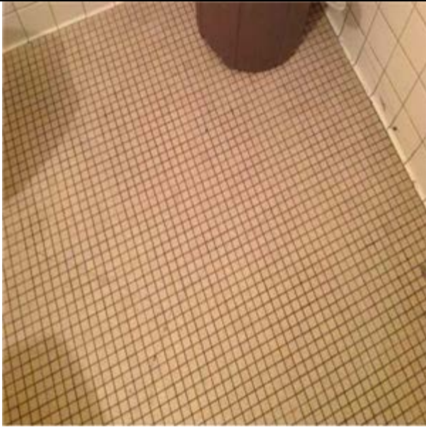
Ceramic Tile Flooring :- bathroom flooring
