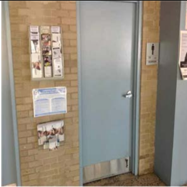
Steel, Painted, Interior Door
