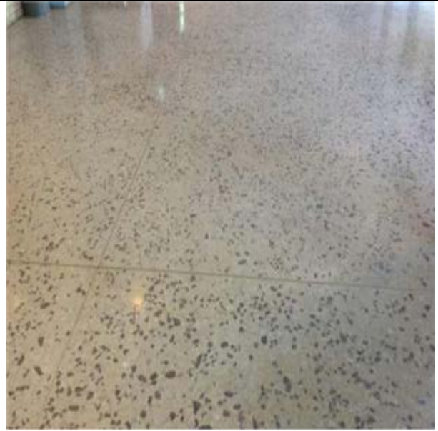
Terrazzo Flooring:- lobby floor
