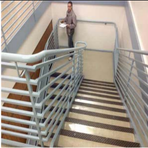
Metal, Painted, Interior Stairs :- (null)
