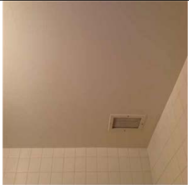
Plaster Ceiling:- plaster ceiling
