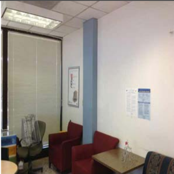
concrete Columns and Beams Frame :- concrete column
