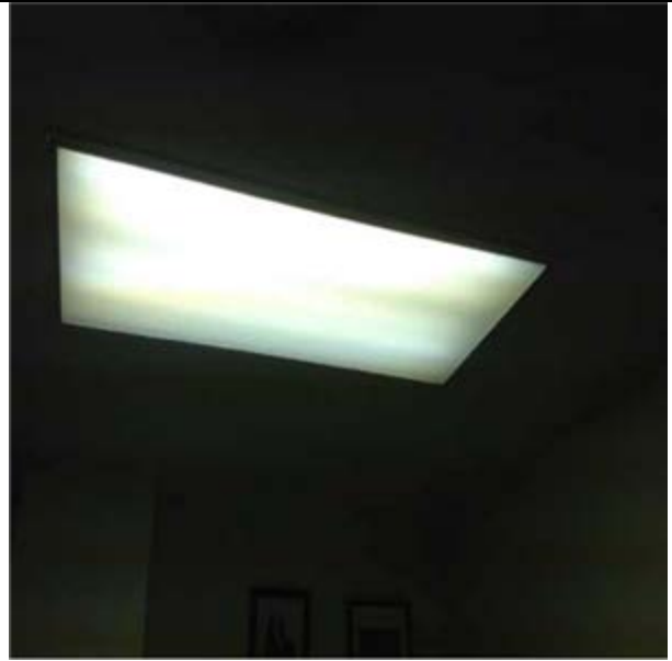
Fluorescent Lighting Fixture, T8, 32w:- (null)
