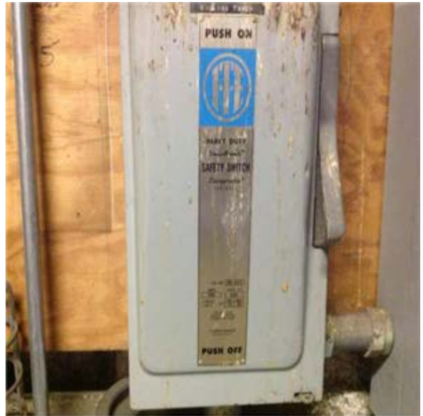
Safety Switch, Fused, 100 Amp, 3 Ph
