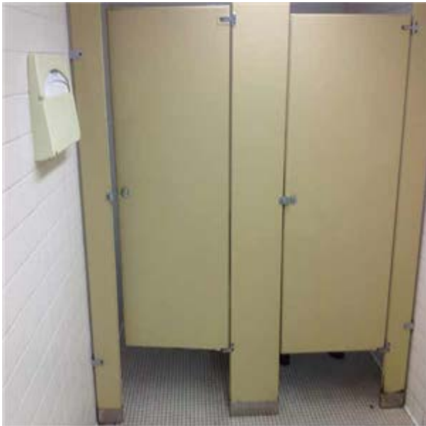
Site Built Toilet Partitions :- metal toilet partitions
