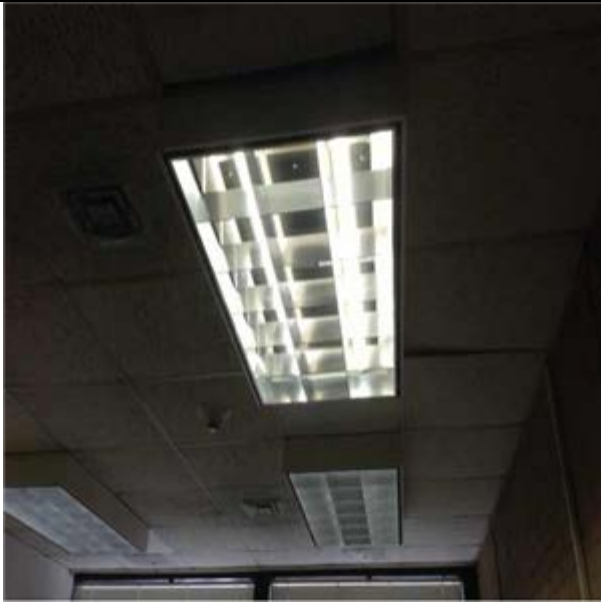
Fluorescent Lighting Fixture, T8, 32w :- (null)
