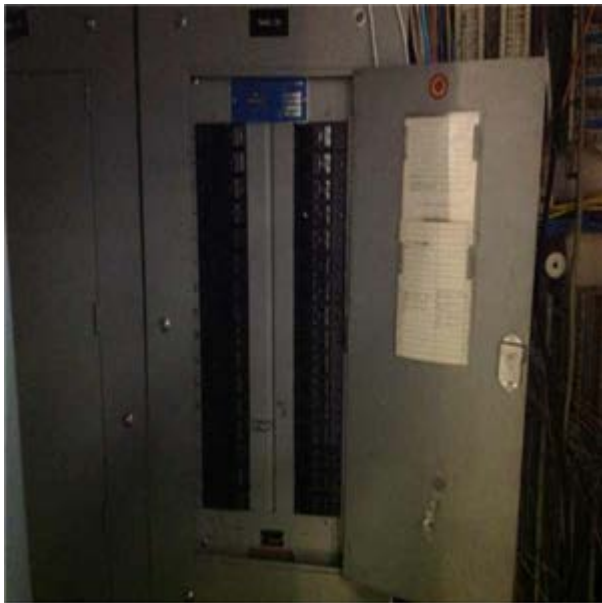
Power Panel Board, 208 Y, 120 V, 100 Amp :- (null)
