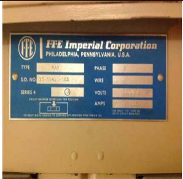
Power Panel Board, 208 Y, 120 V, 225 Amp:- (null)
