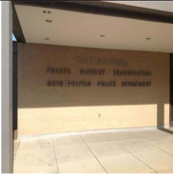
Brick Veneer, Exterior, 1 Story :- at front of building
