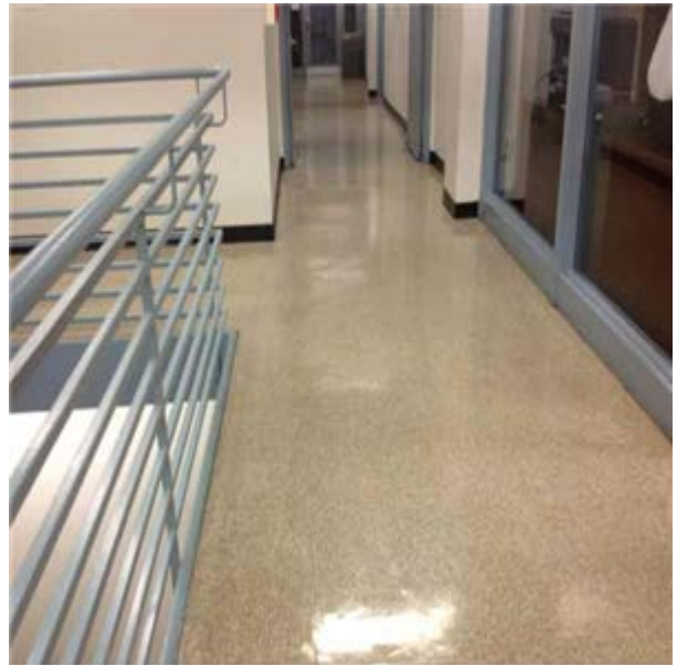
Vinyl Tile Flooring:- 2nd floor vct
