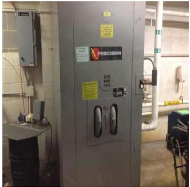
Boiler, Gas, 1,000 Mbh:- 3rd boiler
