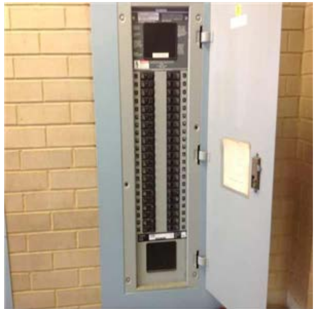
Power Panel Board, 208 Y, 120 V, 225 Amp:- (null)
