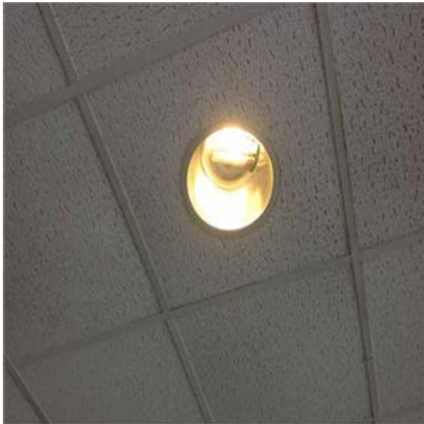
Compact Fluorescent Lighting Fixture Ballast 32 W :- (null)
