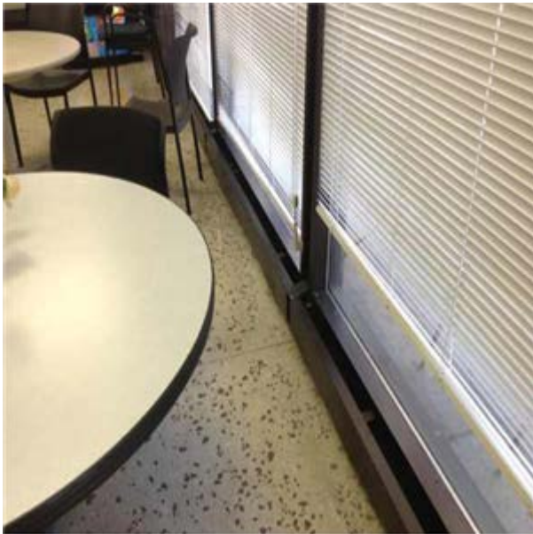
Radiator, Finned, Wall :- baseboard hot water fin tube radiators
