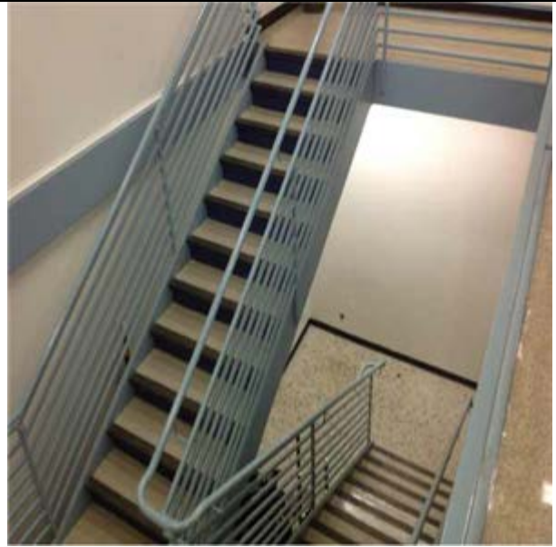
Metal, Painted, Interior Stairs:- (null)
