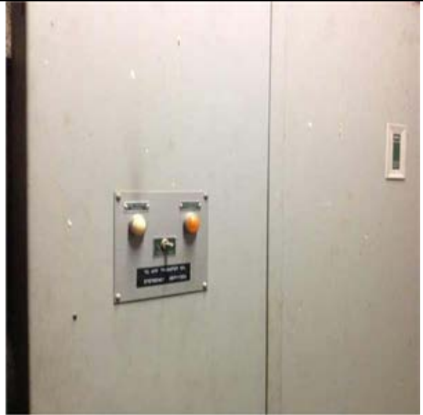
Transfer Switch, Auto, 600 V, 70 Amp:- (null)
