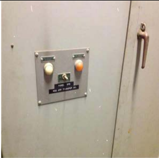
Transfer Switch, Auto, 600 V, 400 Amp :- (null)
