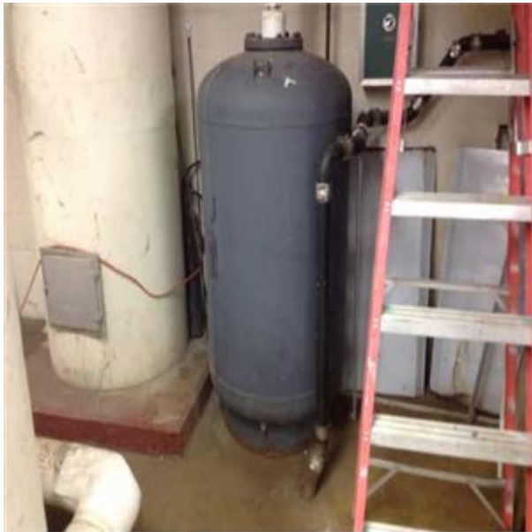
boiler bag tank :- (null)
