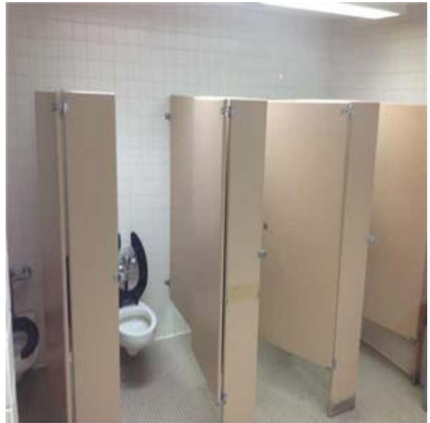
Site Built Toilet Partitions
