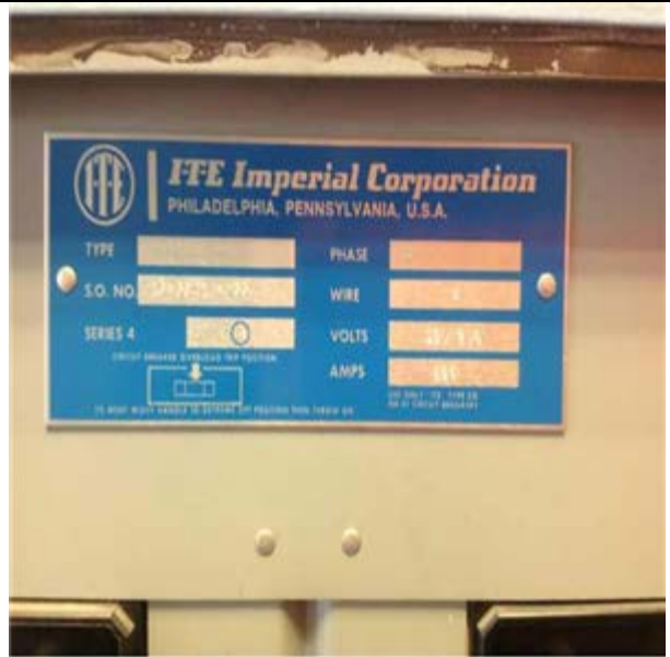
Power Panel Board, 208 Y, 120 V, 225 Amp:- (null)
