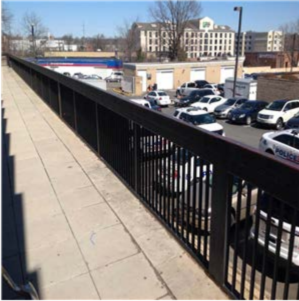
Steel Railing At Rear Patio Area
