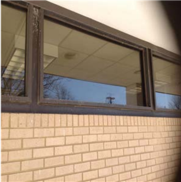
First Floor Aluminum Fixed Pane Window
