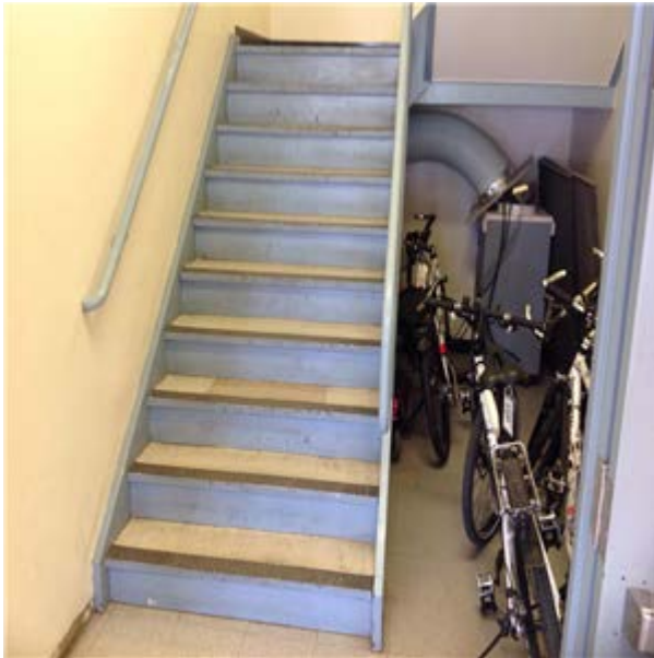
Steel Framed Interior Stair
