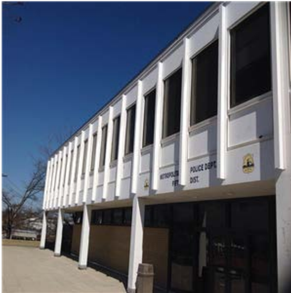
Exterior Wall Steel Panel Finishes
