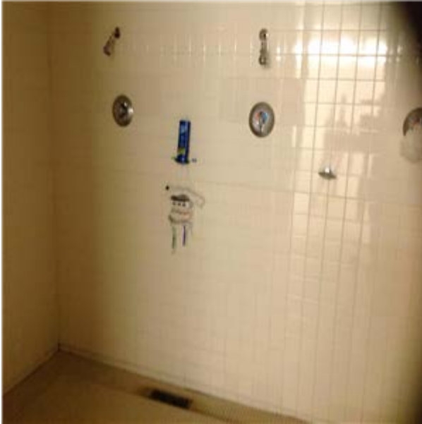
Communal Shower - Locker Room
