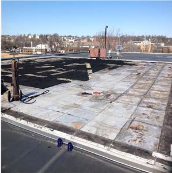
Main Roof Modified Bitumen Membrane
