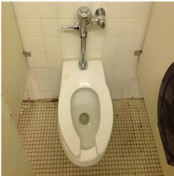
Locker Room Water Closet
