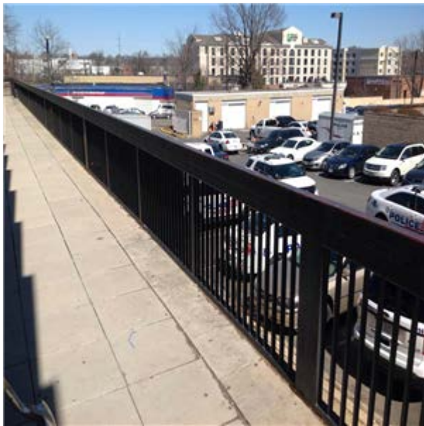
Metal, Painted, Exterior Railing :- Steel Railing At Rear Patio Area
