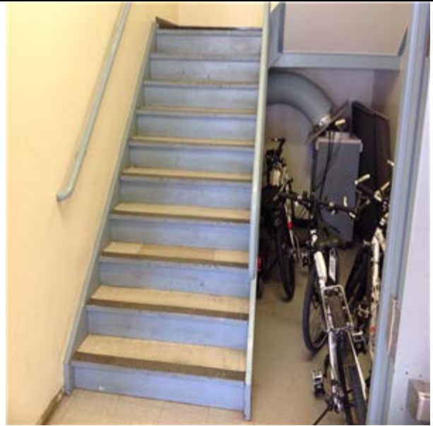
Steel Construction:- Steel Framed Interior Stair
