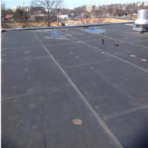
Main Roof EPDM Membrane
