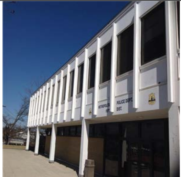
Steel, Painted, Exterior, 2 Stories:- Exterior Wall Steel Panel Finishes
