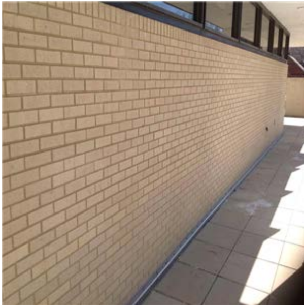
Exterior Wall First Floor Brick Veneer
