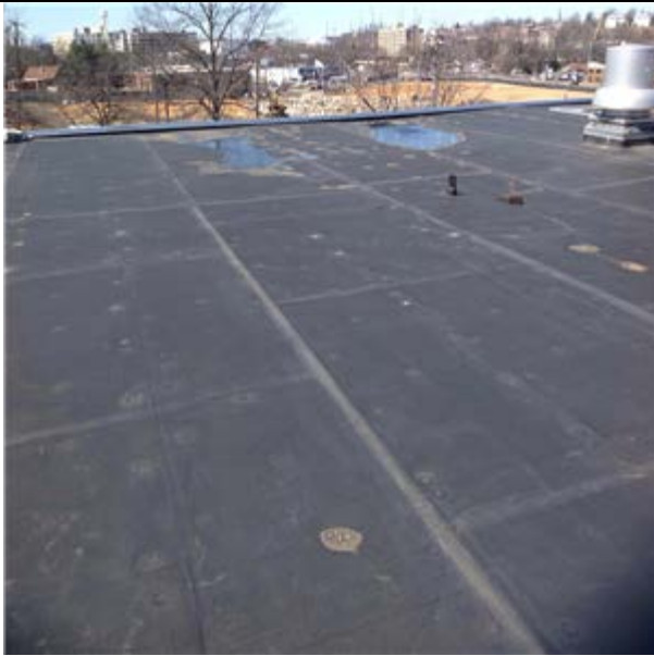
EPDM single-ply membrane :- Main Roof EPDM Membrane
