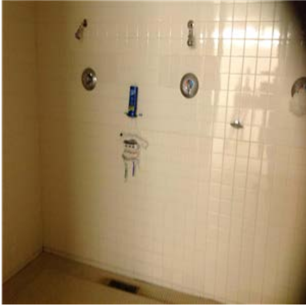
Shower, Ceramic Tile :- Communal Shower - Locker Room
