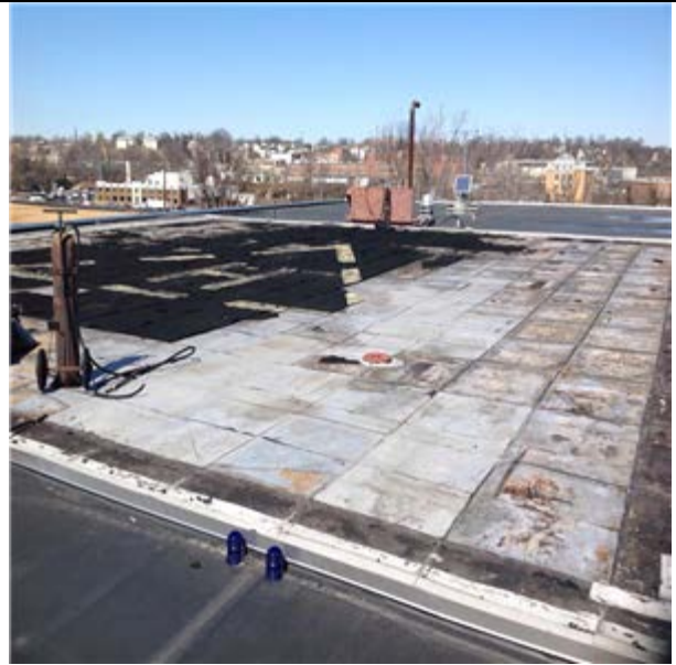
Single-Ply Modified Bituminous/Thermoplastic Roof:- Main Roof Modified Bitumen Membrane
