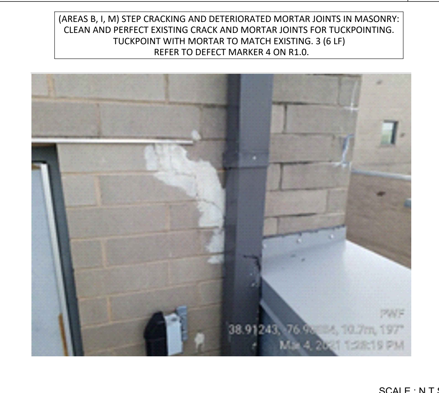
Defect Group #4: Step Cracking 5
