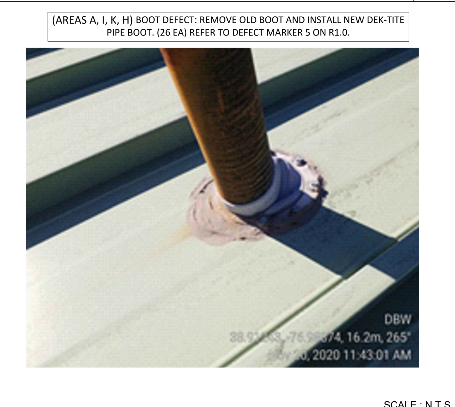
Defect Group #5: Boot Defect 6
