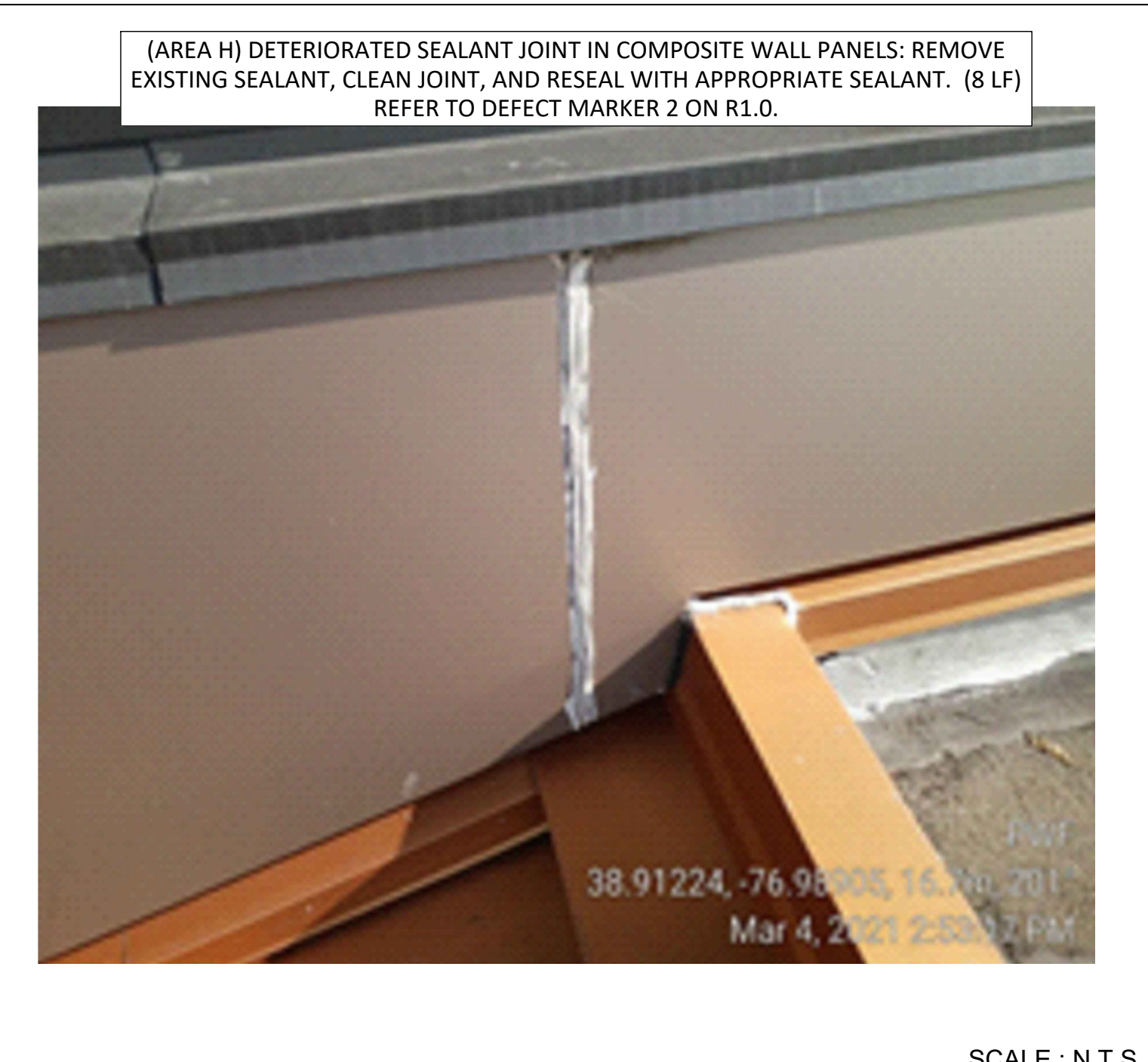
Defect Group #2: Deteriorated Sealant Joint 2
