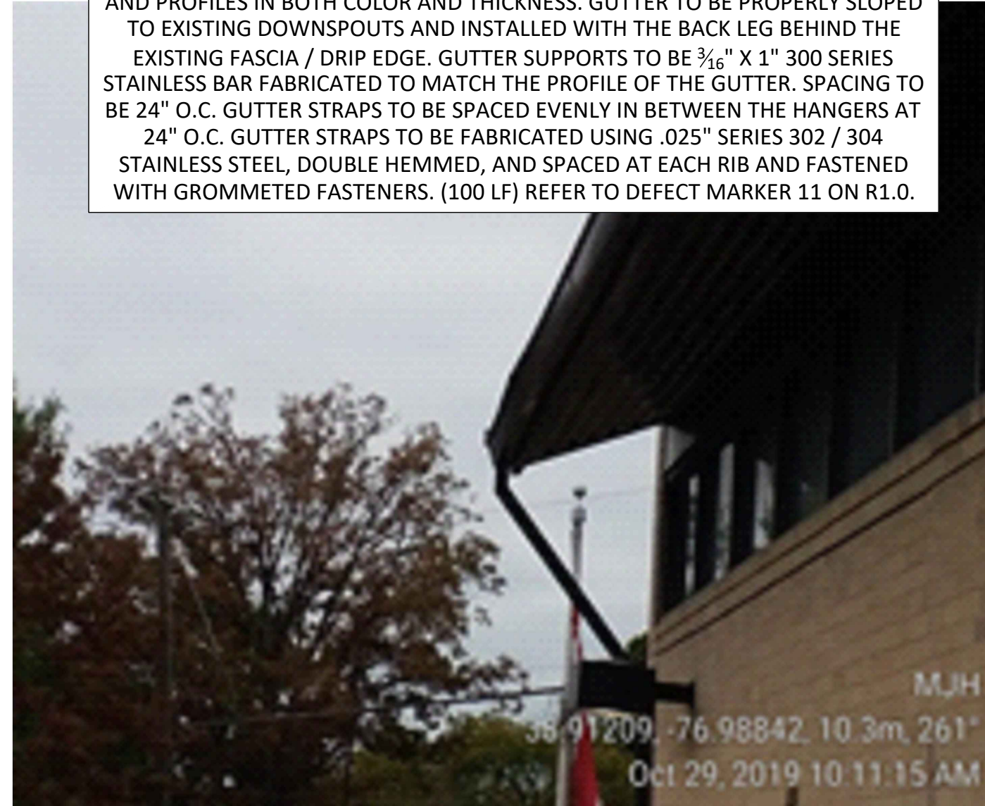
Defect Group #11: Gutter Damage
