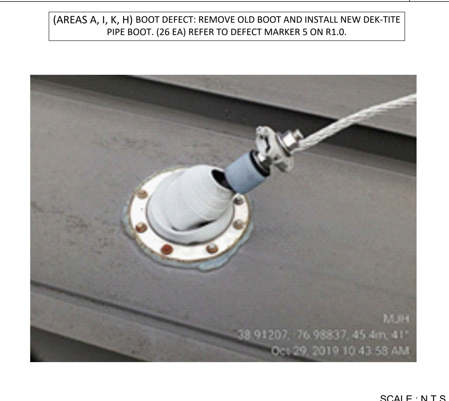
Defect Group #5: Boot Defect 7
