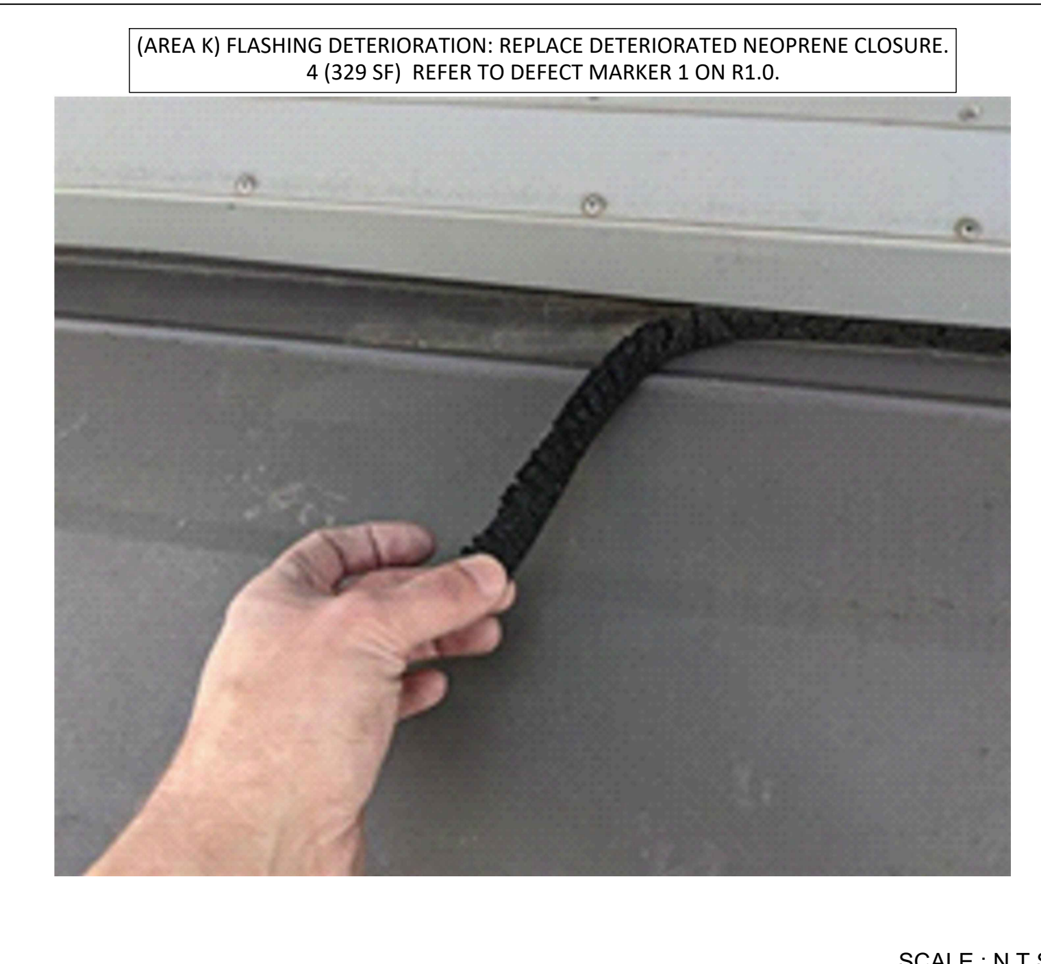
Defect Group #1: Flashing Deterioration 1
