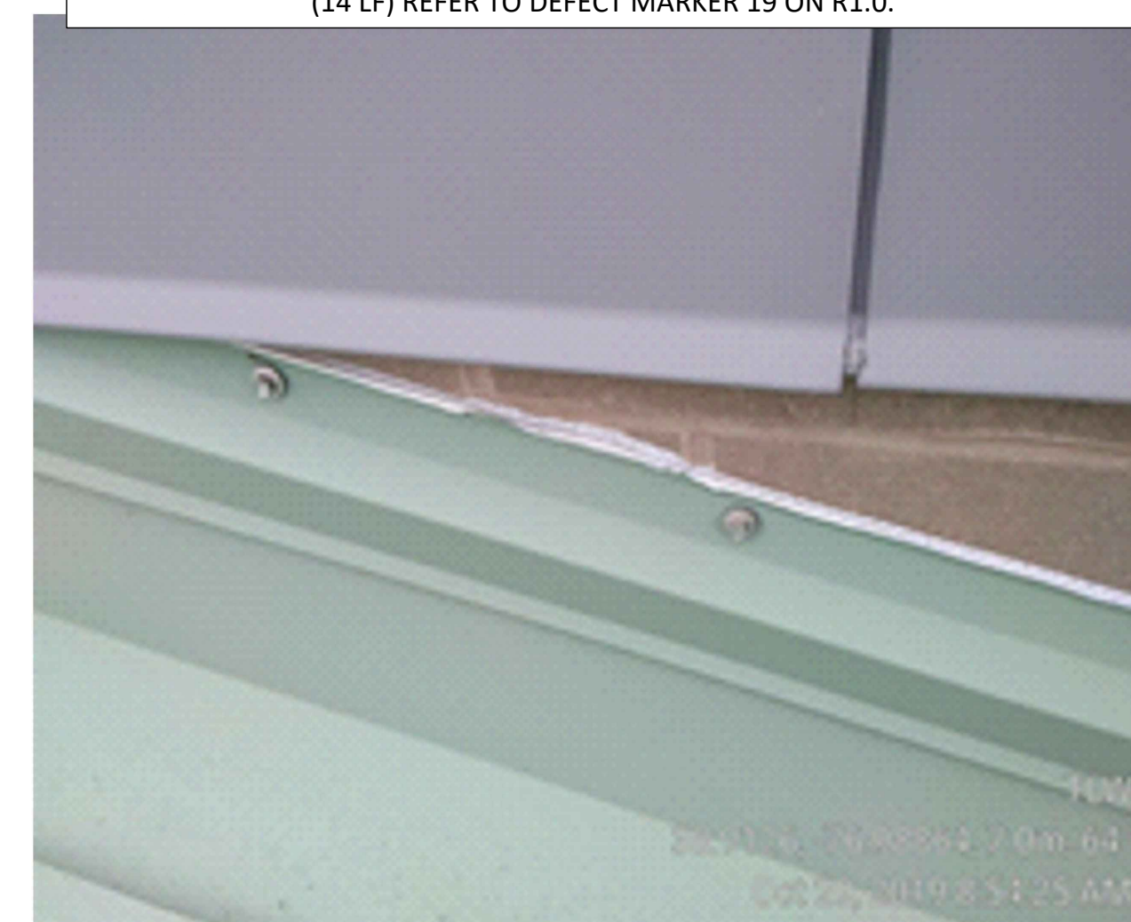
Defect Group #19: Deteriorated Sealant
