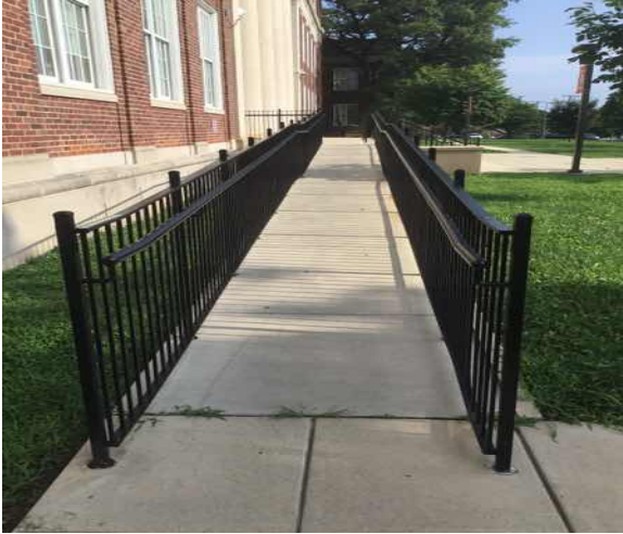
B1014 Ramps:- View of Exterior Concrete Ramps
