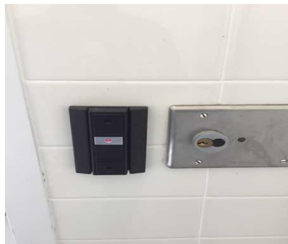
D5038 Security and Detection Systems:- Card Reader
