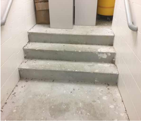
C2011 Regular Stairs:- View of Concrete Interior Stairs
