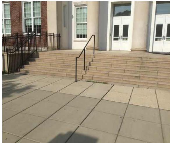
C2011 Regular Stairs:- View of Concrete Exterior Stairs
