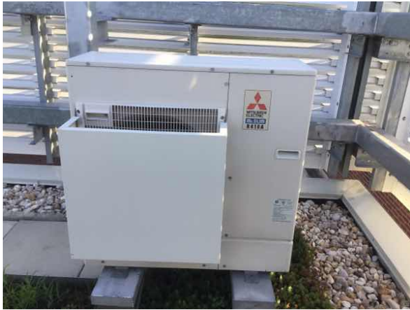
Air-Cooled Condenser
