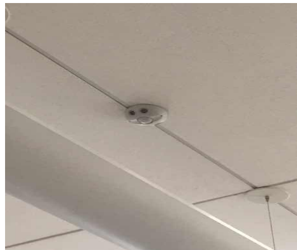
D5021 Branch Wiring Devices:- Occupancy Sensor
