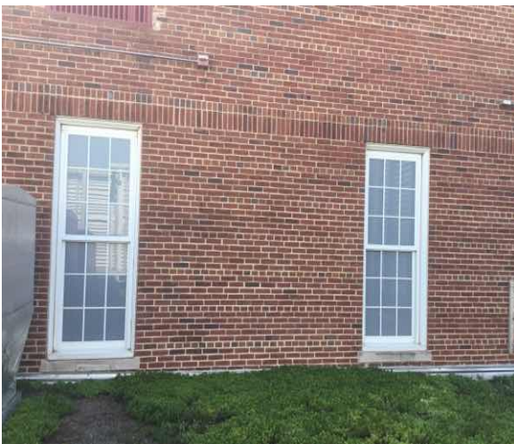
B2021 Windows:- View of Aluminum Fixed Window
