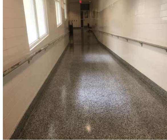
B1014 Ramps:- View of Interior Concrete Ramp
