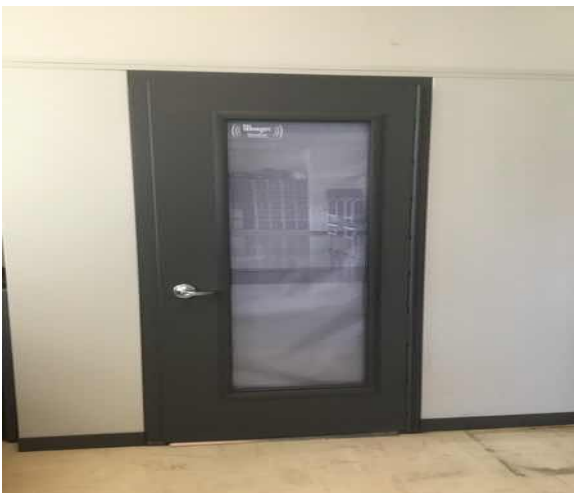
C1021 Interior Doors:- View of Aluminum Fully Glazed Interior Door
