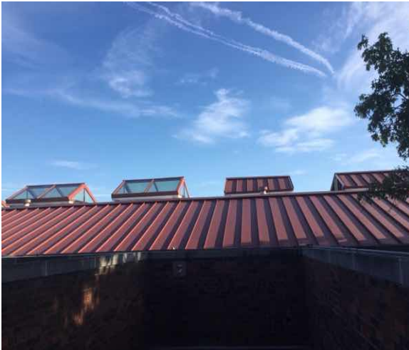
B3011 Roof Finishes:- View of Corrugated Roof Covering
