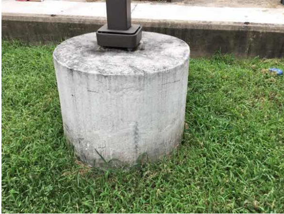
Site Light Foundation
