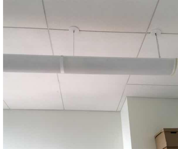
D5022 Lighting Equipment:- Fluorescent Light
