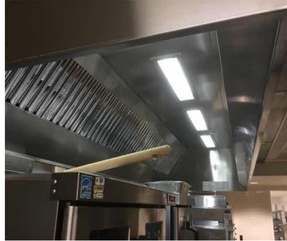
D3042 Exhaust Ventilation Systems:- Kitchen Hood
