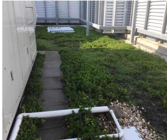
B3011 Roof Finishes:- View of Green Roof w Growing Medium
