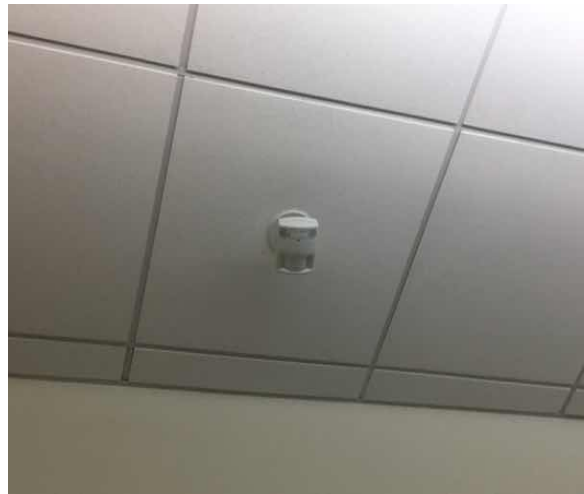
D5038 Security and Detection Systems:- Motion Detector
