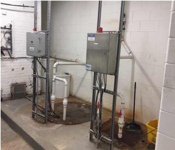
D2043 Rainwater Drainage Equipment:- Sump Pumps
