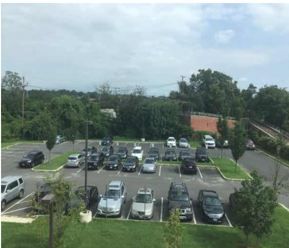
G2022 Paving & Surfacing:- View of Asphalt Paved Parking Lot
