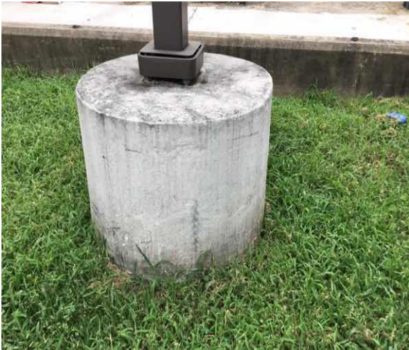
G4022 Poles:- Site Light Foundation
