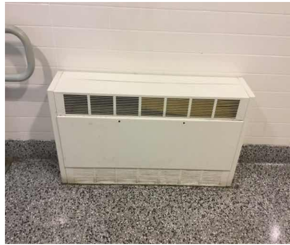
D3051 Terminal Self-Contained Units:- Fan Coil Unit
