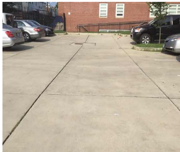
G2022 Paving & Surfacing:- View of Concrete Parking Lots
