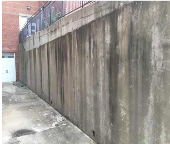
G2042 Retaining Walls:- View of Retaining Wall Cast in Place Concrete
