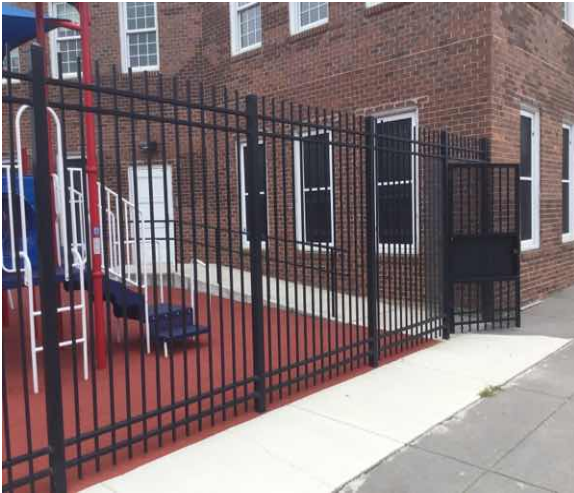
G2041 Fences & Gates:- View of Metal Fence
