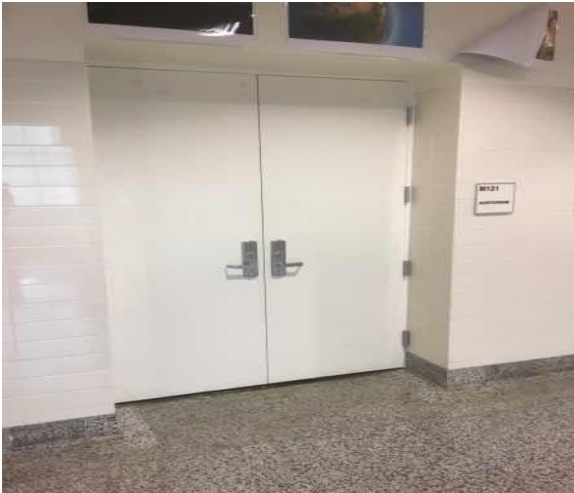
C1021 Interior Doors:- View of Wood Solid Core Interior Door
