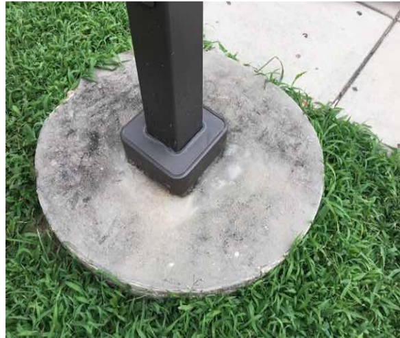
G4022 Poles:- Site Light Foundation
