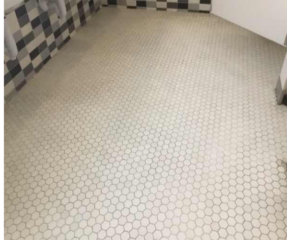
C3024 Flooring:- View of Ceramic Tile Flooring
