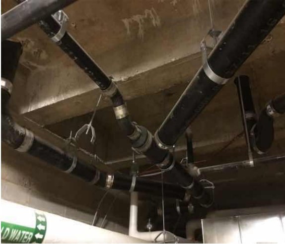
D2031 Waste Piping:- Sanitary Waste Piping
