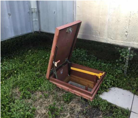
B3022 Roof Hatches:- View of Aluminum Roof Hatch
