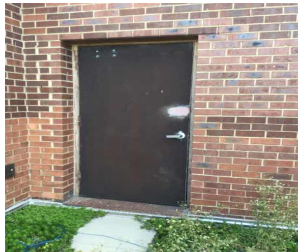
B2031 Glazed Doors & Entrances:- View of Steel Exterior Door
