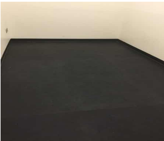
C3024 Flooring:- View of Rubber Floor Finish
