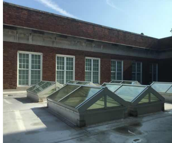
B3021 Glazed Roof Openings:- View of Metal Frame Skylights
