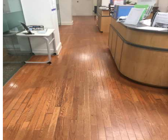
C3024 Flooring:- View of Wood Strip Floor Finishes
