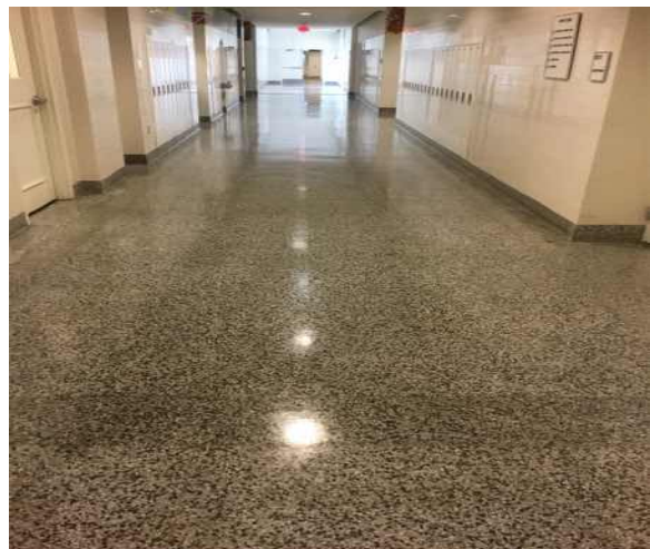
C3024 Flooring:- View of Terrazzo Floor Finish
