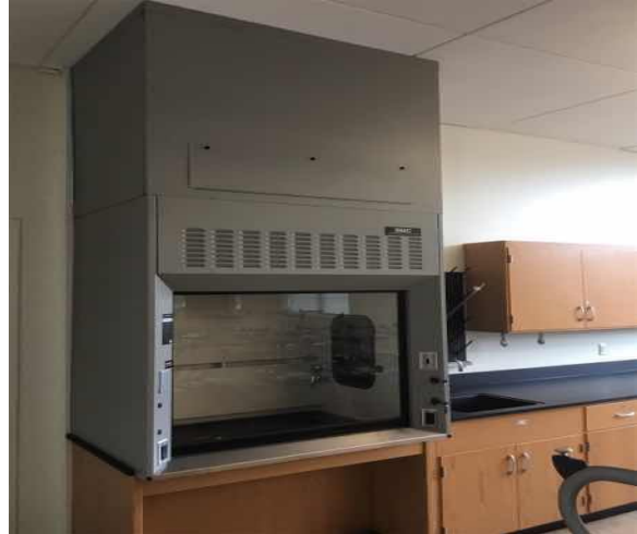
E1027 Laboratory Equipment:- Laboratory Exhaust Hood
