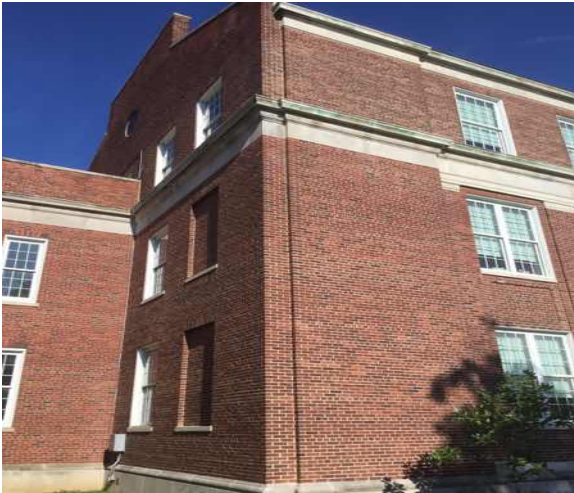
B2011 Exterior Wall Construction:- View of Clay Brick Exterior Wall
