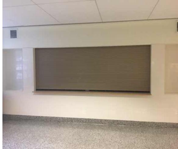
B2039 Other Doors & Entrances:- View of Steel Doors & Entrances, Rolling Door
