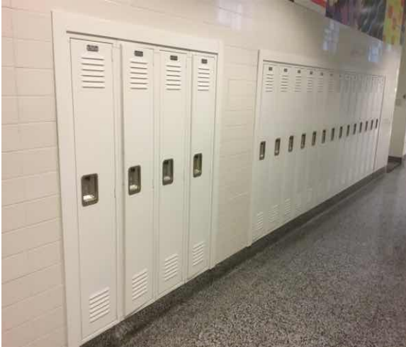
E2012 Fixed Casework:- View of Painted Metal Lockers
