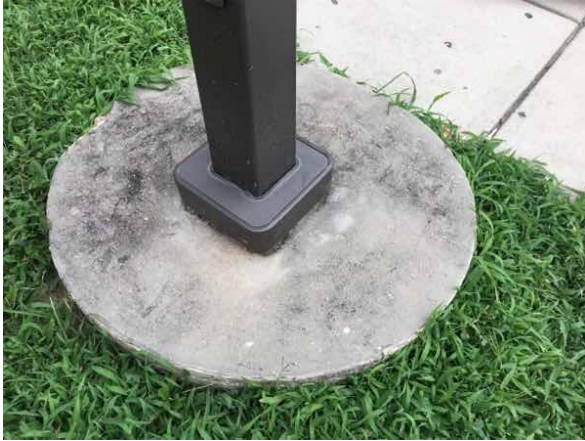
Site Light Foundation
