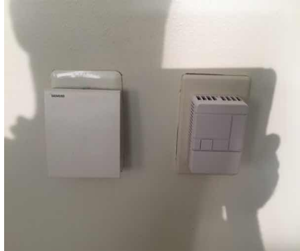
D3068 Building Automation Systems:- Thermostats
