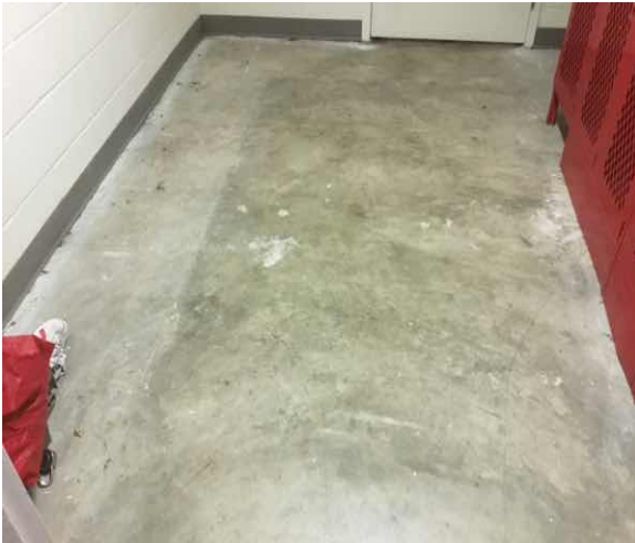
C3024 Flooring:- View of Concrete Flooring
