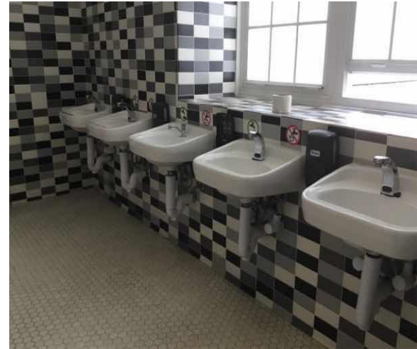
D2010.0 Water_Fixtures:- Laboratory Sink
