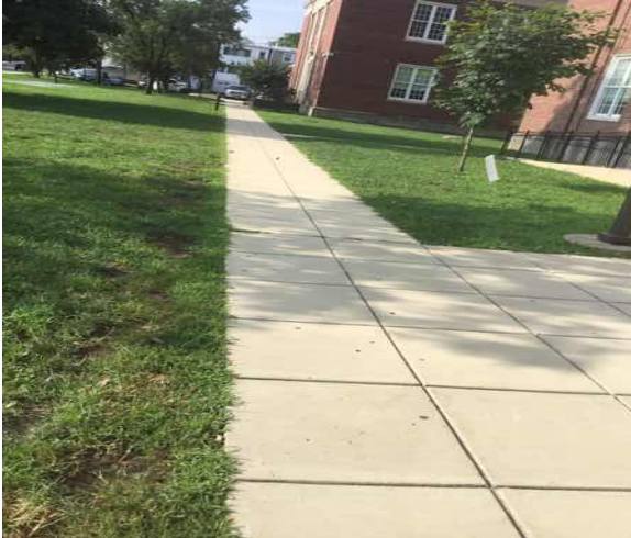
G2022 Paving & Surfacing:- View of Concrete Pavement
