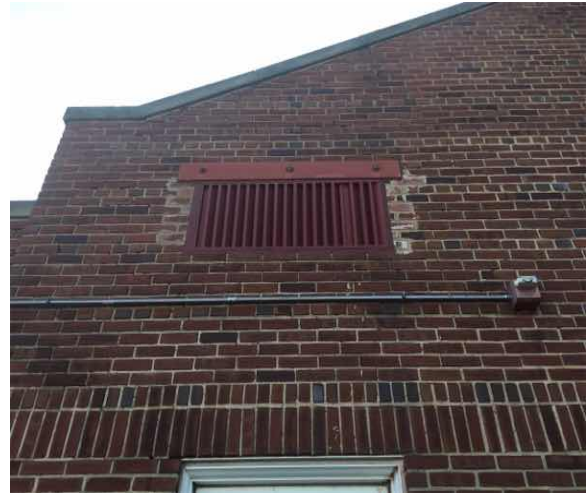
B2013 Exterior Louvers, Screens, and Fencing:- View of Aluminum Louver
