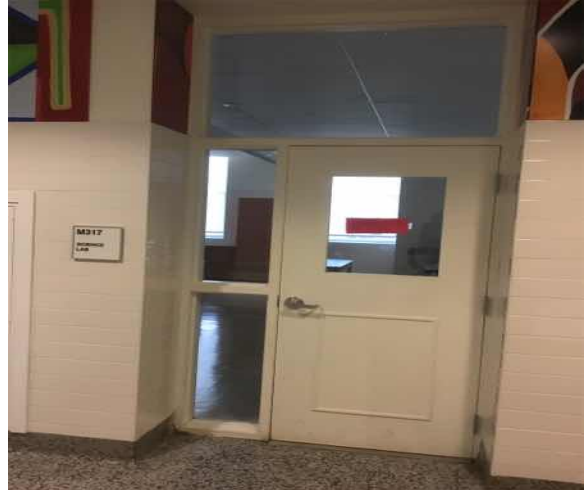
C1021 Interior Doors:- View of Wood Safety Glass Painted Interior
