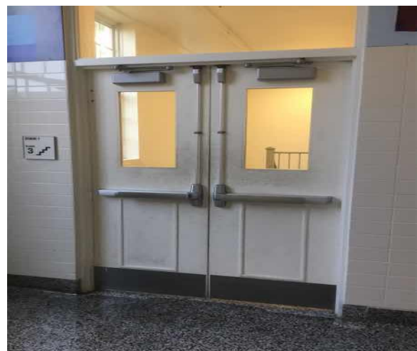
C1021 Interior Doors:- View of Fire Doors
