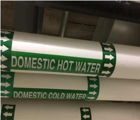
D2021 Cold Water Service:- Domestic Water Piping
