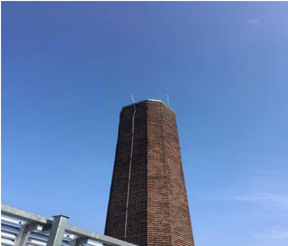
D5091 Grounding Systems:- Lightning Protection
