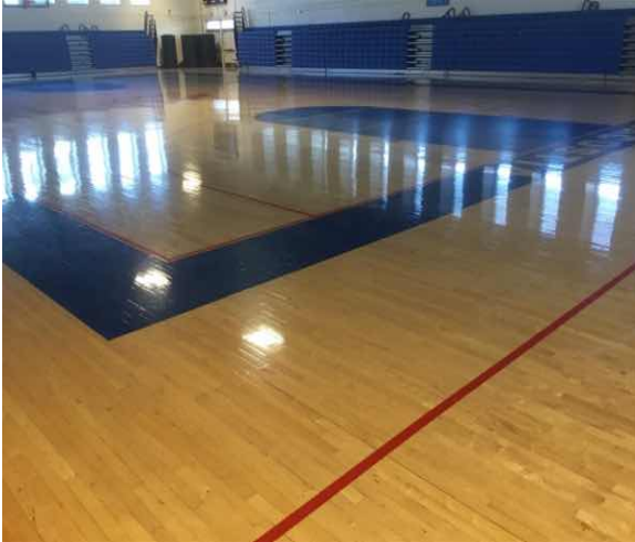
C3024 Flooring:- View of Athletic Wood Floor Finish
