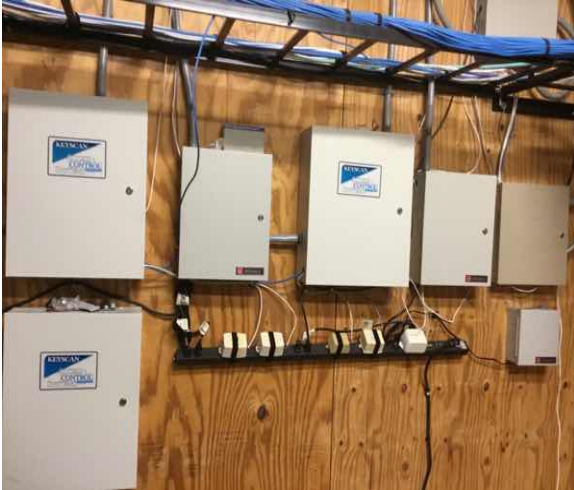
D5038 Security and Detection Systems:- Access Control Panel
