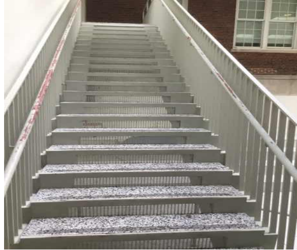
C2011 Regular Stairs:- View of Metal Interior Stairs
