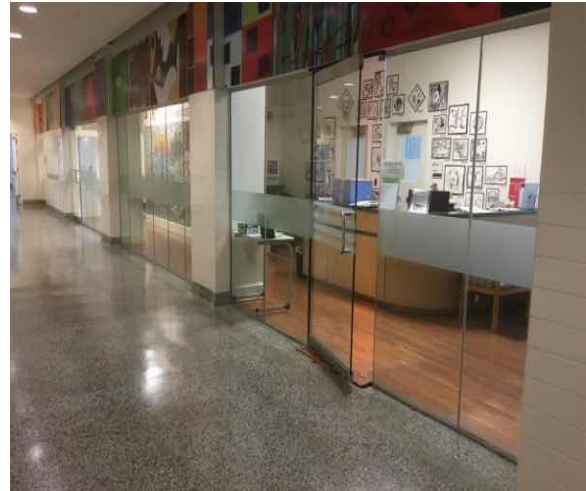
C1017 Interior Windows & Storefronts:- View of Interior Windows & Storefronts - Standard
