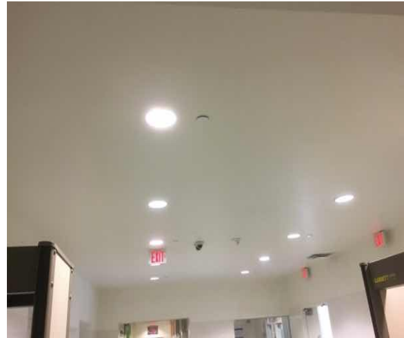
C3031 Ceiling Finishes:- View of Gypsum Board Ceiling Finishes
