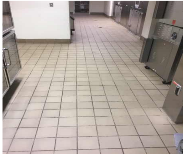
C3024 Flooring:- View of Quarry Tile Flooring
