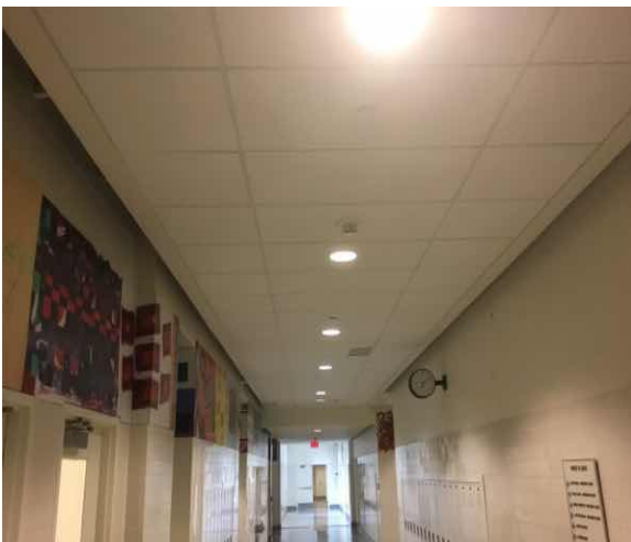
C3032 Suspended Ceilings:- View of Acoustical Tile Ceiling
