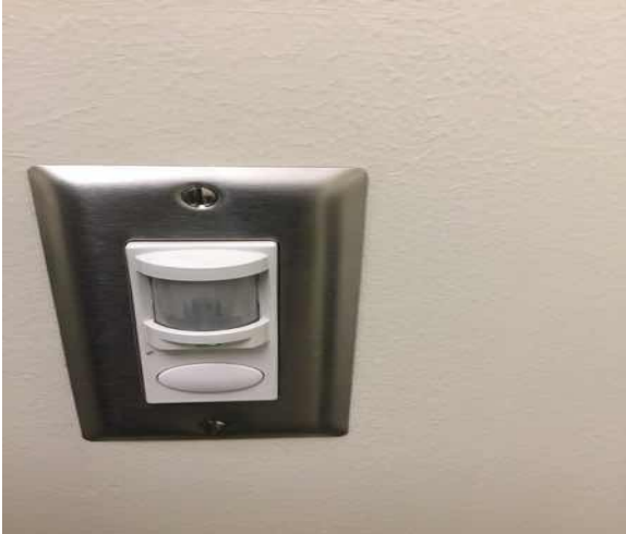
D5021 Branch Wiring Devices:- Occupancy Sensor Receptacle
