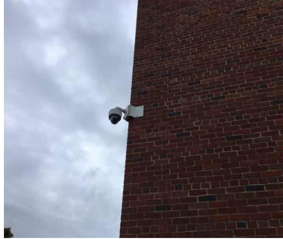
D5038 Security and Detection Systems:- Surveillance Camera
