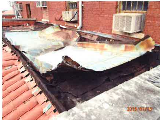
Photo 4. Area 2: Loss of roofing and waterproofing membrane
