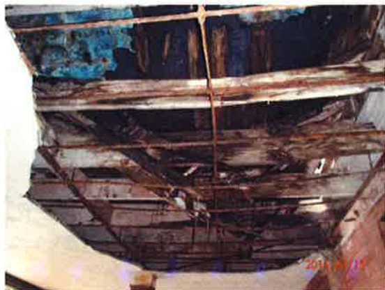
Photo 6. Area 2: Deterioration and failure of rafters
