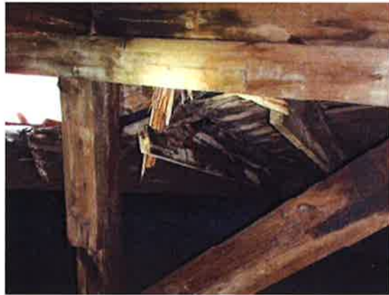
Photo 2. Area 1: Deterioration of rafters and decking
