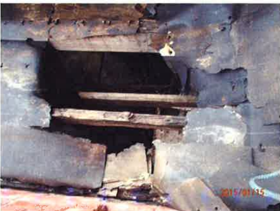
Photo 5. Area 2: Opening in the roofing to exposing rafters
