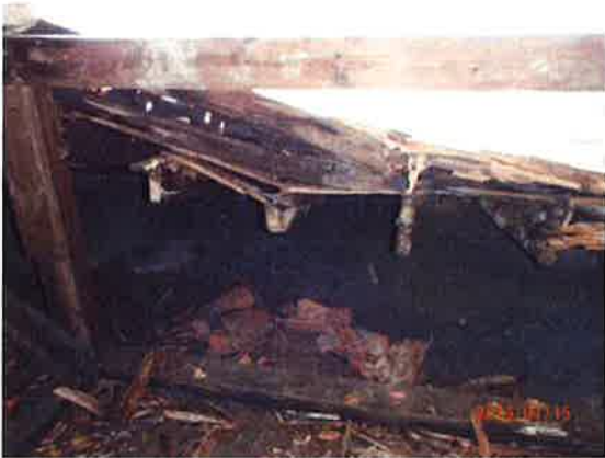
Photo 1. Area 1: Failure of wood frame
