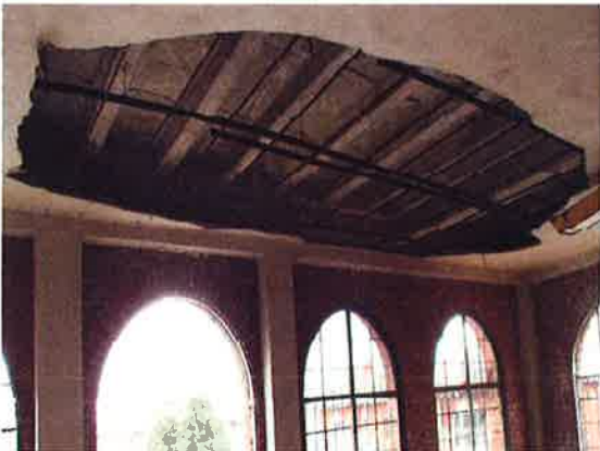
Photo 3. Underside of Area 1 showing concrete joists
