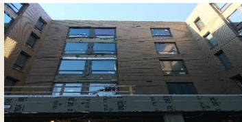
View of finished masonry from interior of courtyard.
