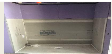
View of shower compartment install before drywall finishes are applied.
