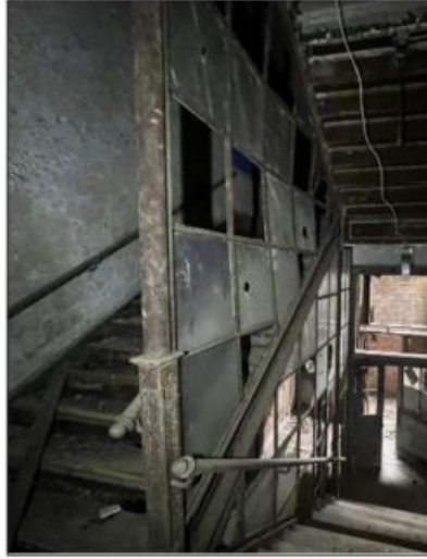
Figure 6: Glass and metal frame enclosures at southern stair.
