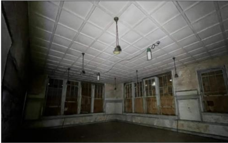
Figure 7: Second floor classroom, note intact ceiling.
