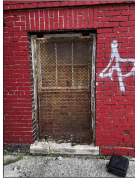
Figure 4: Basement level window with security screen, infilled with brick.
