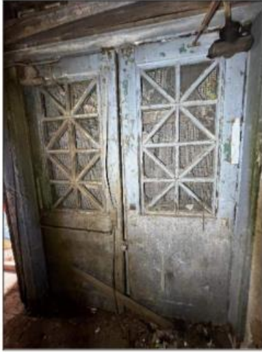
Figure 5: Wooden door at northern entrance.
