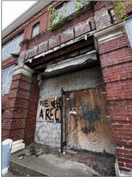
Figure 3: Entrance on north elevation.
