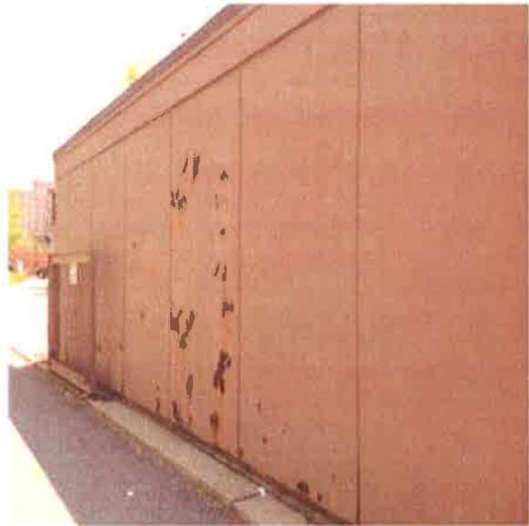
Steel, Exterior, 2 Stories:- Typical Deteriorated Paint and Oxidation at Exterior Steel
