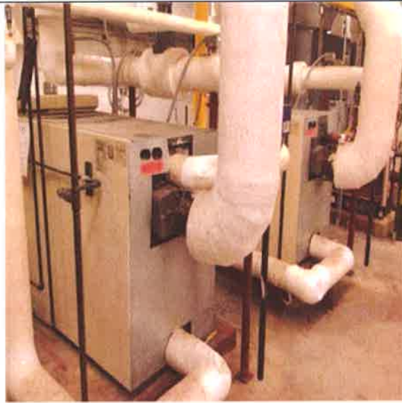
Boiler, Gas, 4,200 Mbh :- Central Heating Boilers
