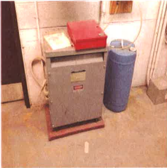
Secondary Transformer
