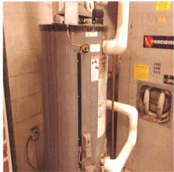
Domestic Hot Water Heater - Gas:- Domestic Hot Water Storage Tank
