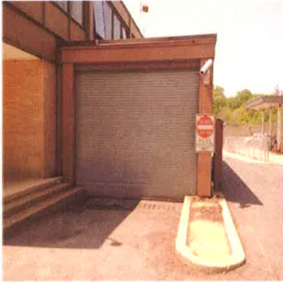
Typical Aluminum Roll Up Door
