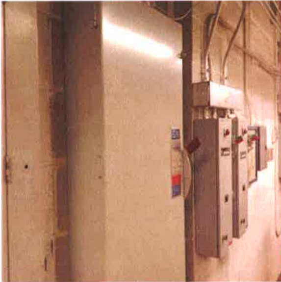
Chiller 400 Amp Disconnect Switch
