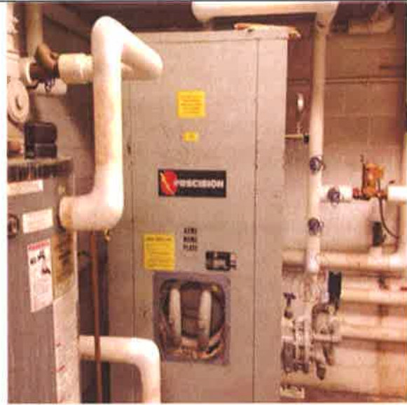
Boiler, Gas, 2,000 Mbh:- Domestic Hot Water Boiler
