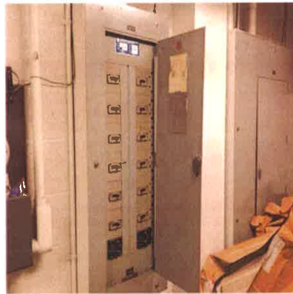
Power Panel Board, 480 Y, 277 V, 200 Amp :- 225 Amp Circuit Breaker Panel
