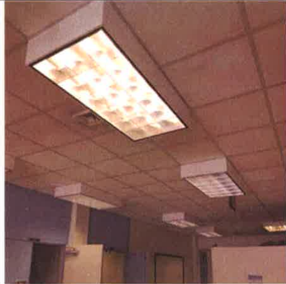
Fluorescent Lighting Fixture, T8, 32 W:- Typical Fluorescent Light Fixture
