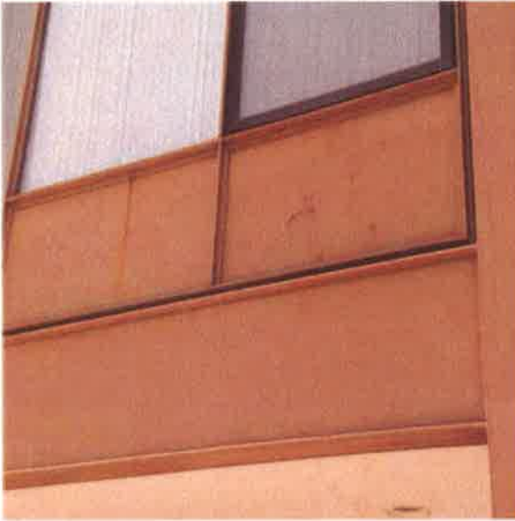
Typical Deteriorated Paint and Oxidation at Exterior Sterl
