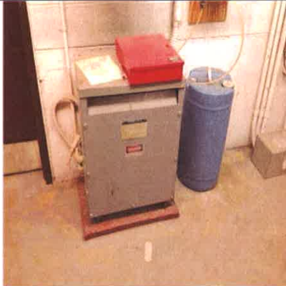
Secondary Transformer, Dry, 30 kVA :- Secondary Transformer
