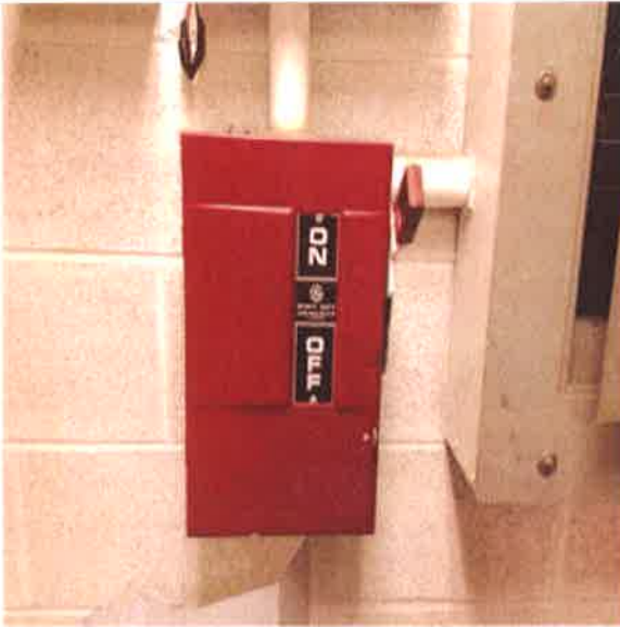
100 Amp Electric Disconnect Switch
