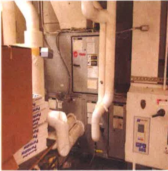
Boiler Room Air Handler Unit
