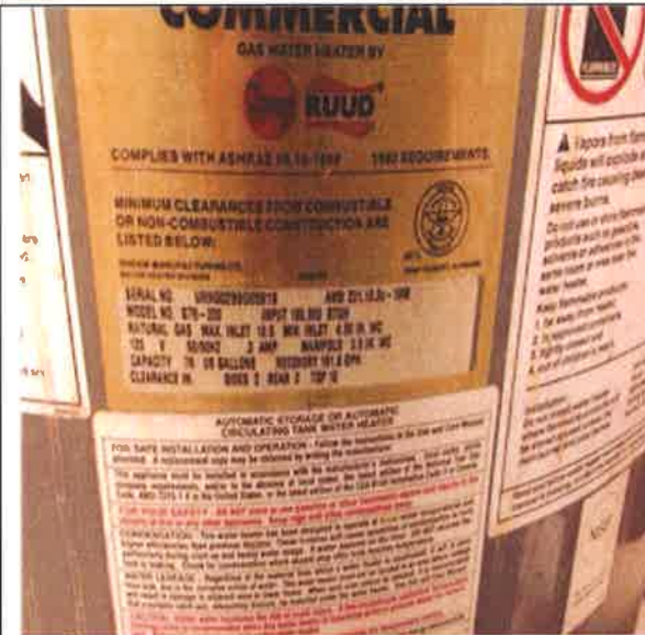
Domestic Hot Water Heater - Gas :- Domestic Hot Water Storage Tank Nameplate
