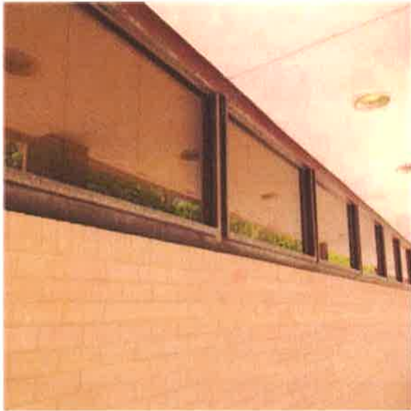
First Floor Aluminum Framed Windows
