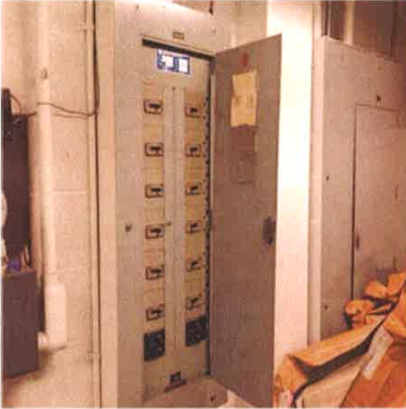
225 Amp Circuit Breaker Panel
