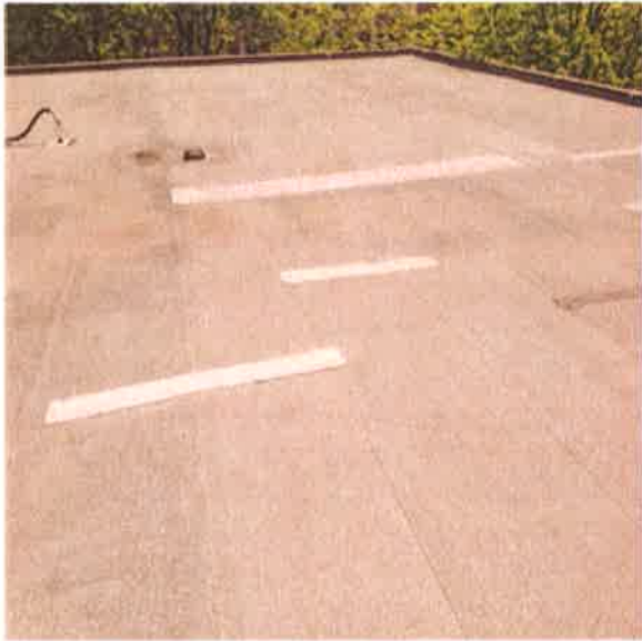
Modified Bitumen Roof Coverings
