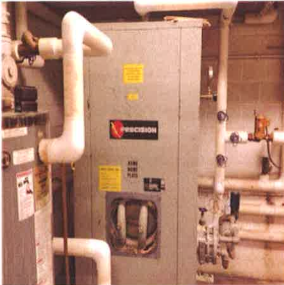
Domestic Hot Water Boiler
