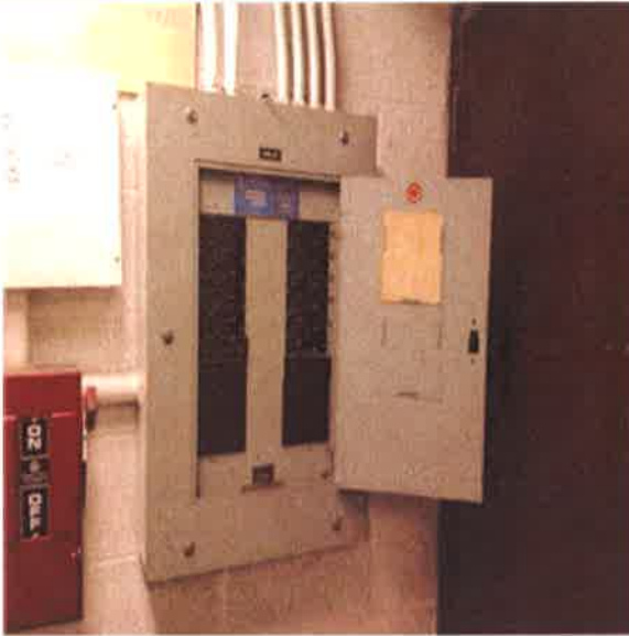
100 Amp Circuit Breaker Panel
