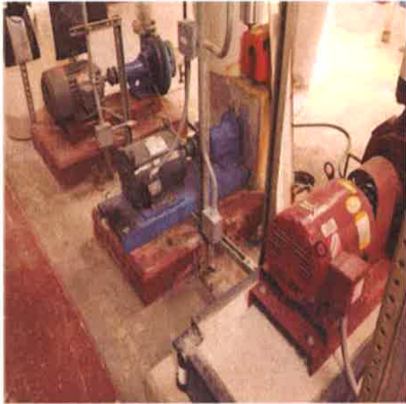
Conditioned Water Circulation Pumps
