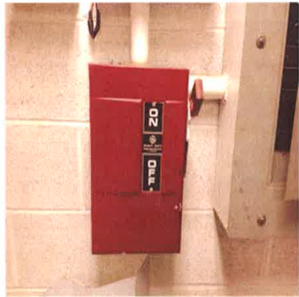
Disconnect Switch, 100 Amp:- 100 Amp Electric Disconnect Switch
