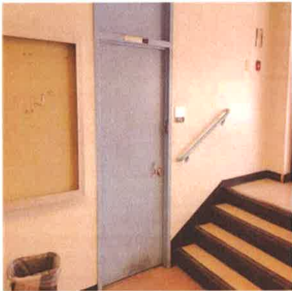
Typical Interior Painted Steel Door
