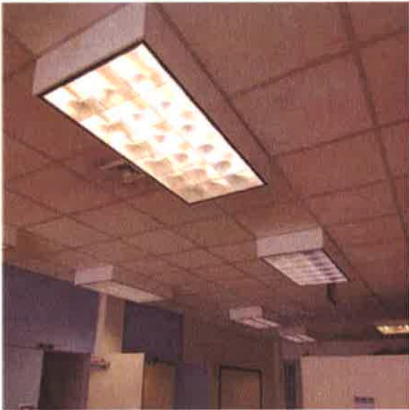
Typical Fluorescent Light Fixture
