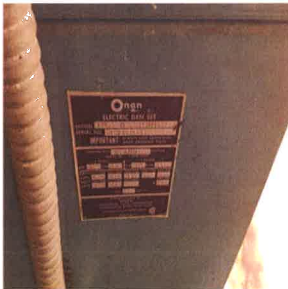
Generator, Diesel, 175 kW :- Backup Generator Nameplate
