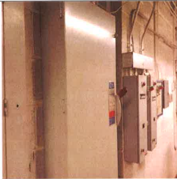
Disconnect Switch, 400 Amp:- Chiller 400 Amp Disconnect Switch
