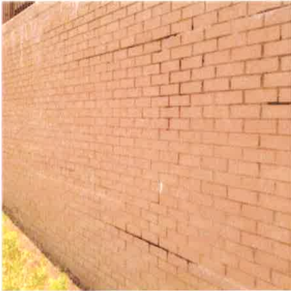
Typical Exterior Brick Mortar Deterioration
