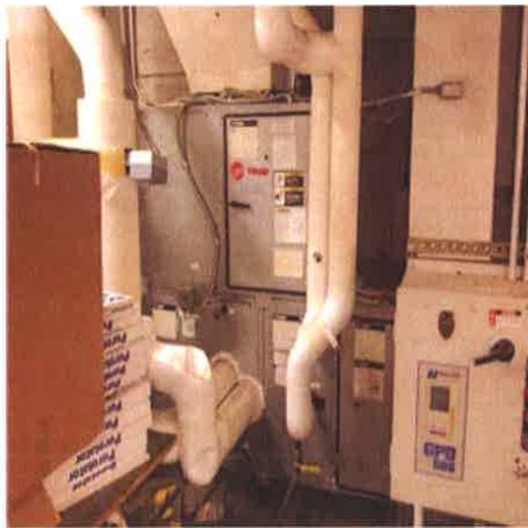
Air Handler, Multizone, 40,000 Cfm :- Boiler Room Air Handler Unit
