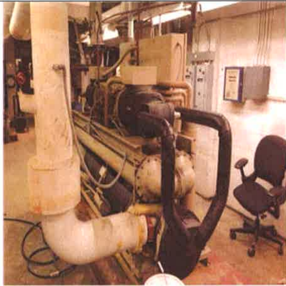
Chiller, Reciprocal Air-Cooled Hermetic, 200 Ton :- Central Chiller Unit
