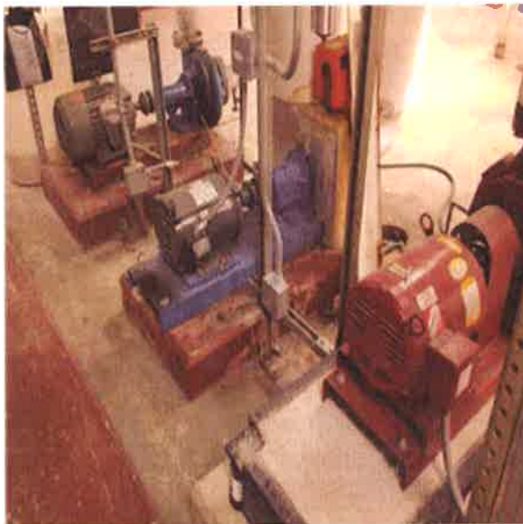
Circulation Pump, Hot Water, 7.500 HP :- Conditioned Water Circulation Pumps
