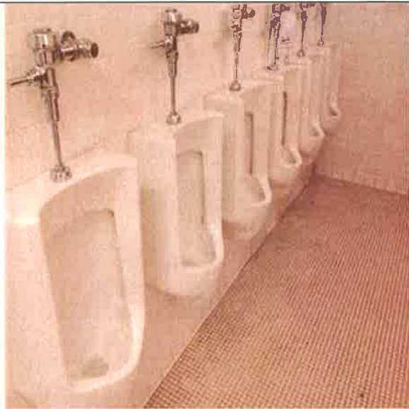
Urinal, Vitreous China :- Typical Wall Hung Urinals
