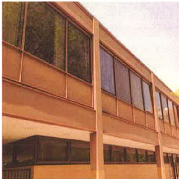
Alum Fixed Thermal Break, Double Glazing, 2 Story, 24SF :- Second Floor Aluminum Framed Windows and Painted Steel Exterior
