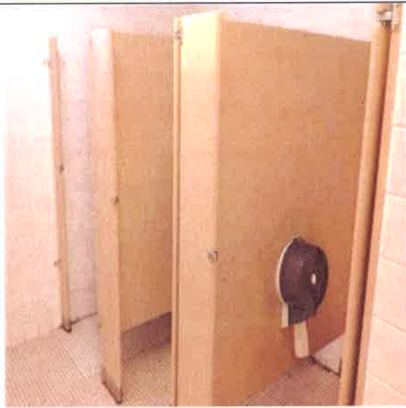
Site Built Toilet Partitions :- Typical Toilet Partitions
