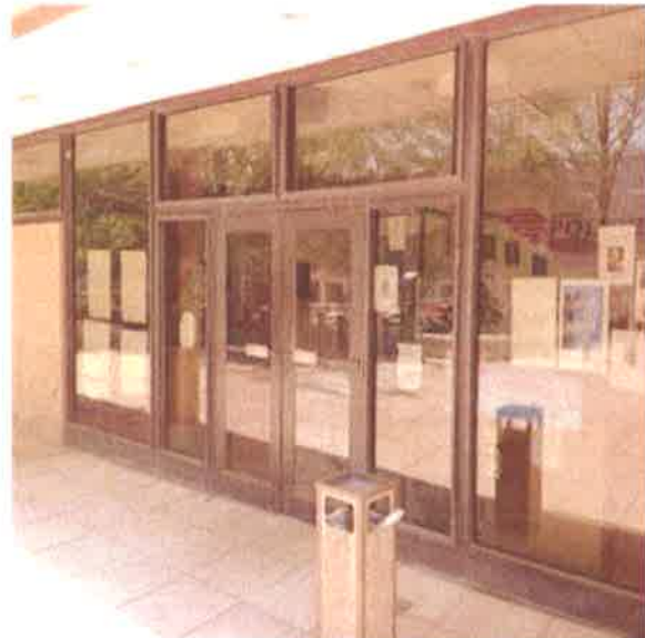
Glazed Aluminum Framed with Swing Doors:- Main Building Entry Storefront
