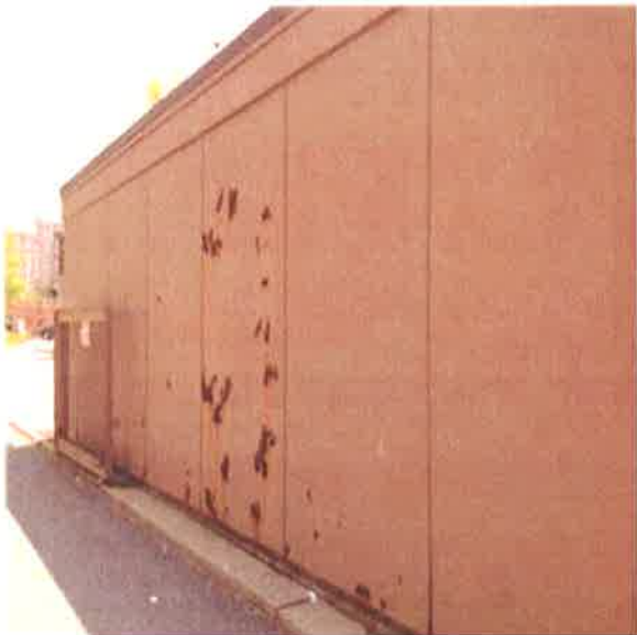
Typical Deteriorated Paint and Oxidation at Exterior Steel
