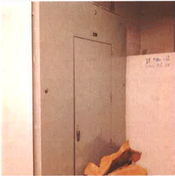
400 Amp Circuit Breaker Panel
