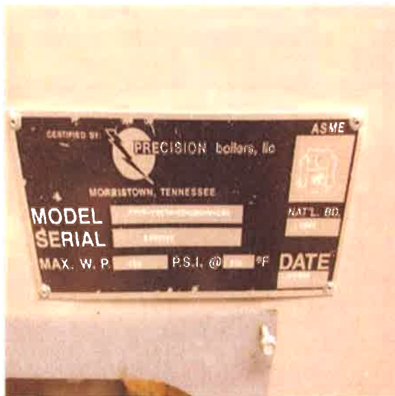
Boiler, Gas, 2,000 Mbh :- Domestic Hot Water Boiler Nameplate
