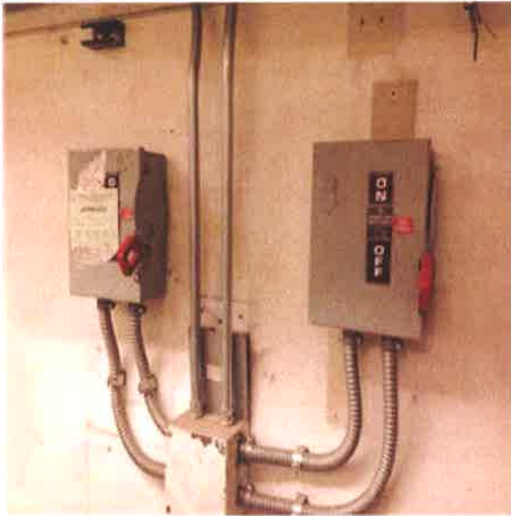
Typical 30 Amp Electric Disconnect Switches
