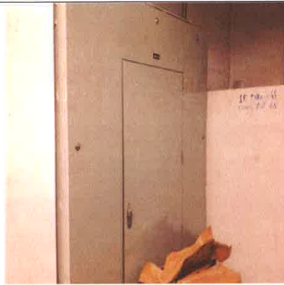
Power Panel Board, 208 Y, 120 V, 400 Amp :- 400 Amp Circuit Breaker Panel
