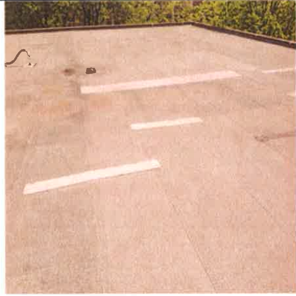
Modified Bitumen - Single Ply:- Modified Bitumen Roof Coverings
