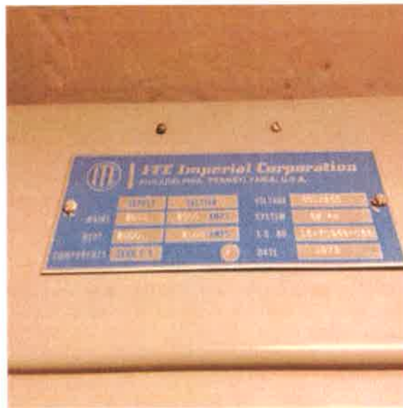
Main Switchgear, 208 Y, 120 V, 2,000 Amp:- Main Electric Switchgear Nameplate
