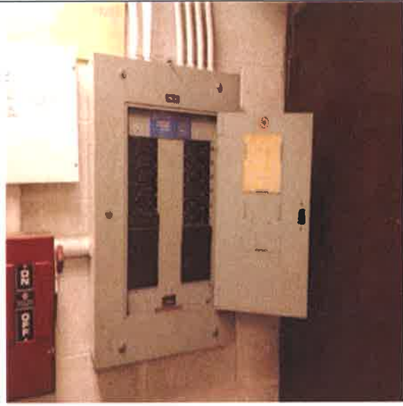
Power Panel Board, 480 Y, 277 V, 100 Amp:- 100 Amp Circuit Breaker Panel
