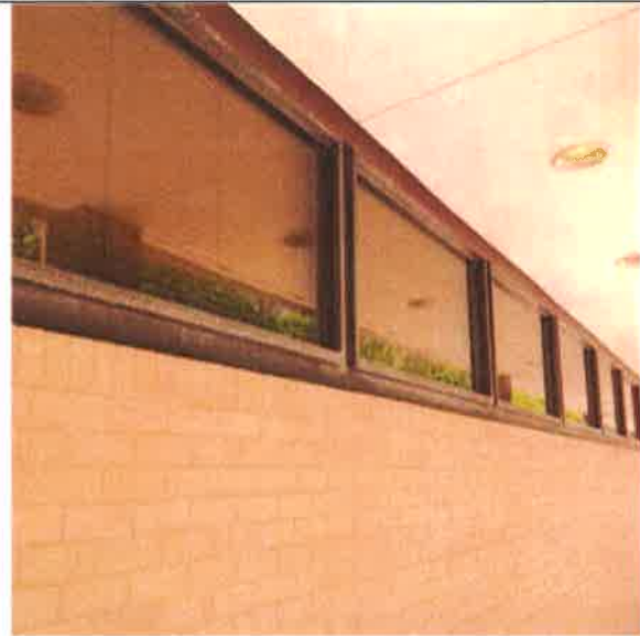
Alum Fixed Thermal Break, Double Glazing, 1 Story, 12SF:- First Floor Aluminum Framed Windows
