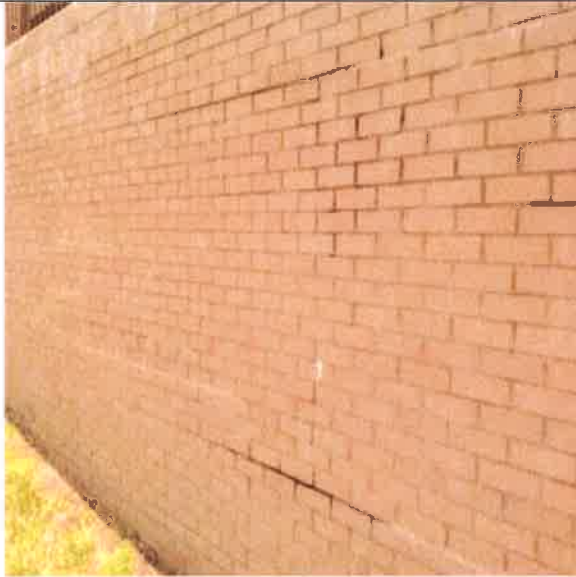
Brick Veneer, Exterior, 1 Story :- Typical Exterior Brick Mortar Deterioration
