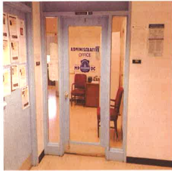
Wood, Painted, Fully Glazed, Interior Door:- Typical Glazed Interior Door
