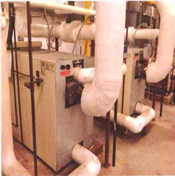
Central Heating Boilers
