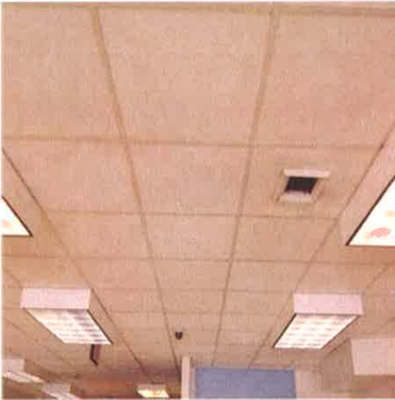
Typical Acoustic Ceiling Tiles
