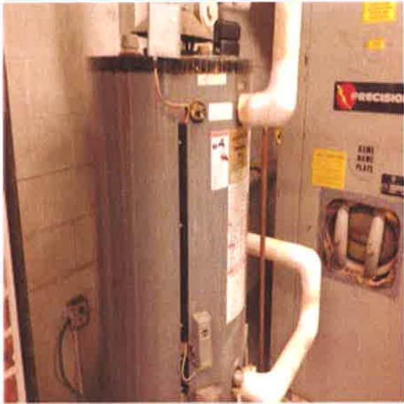
Domestic Hot Water Storage Tank
