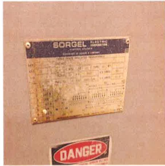
Secondary Transformer, Dry, 30 kVA:- Secondary Transformer Nameplate
