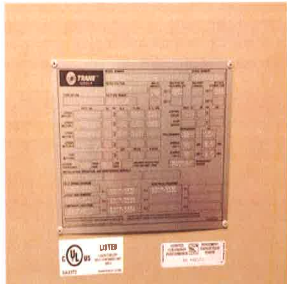
Chiller, Reciprocal Air-Cooled Hermetic, 200 Ton:- Central Chiller Nameplate
