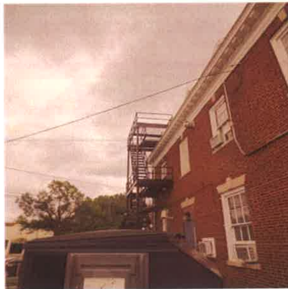
Metal, Exterior Stairs :- Emergency Exit Stairs from Second and third floor
