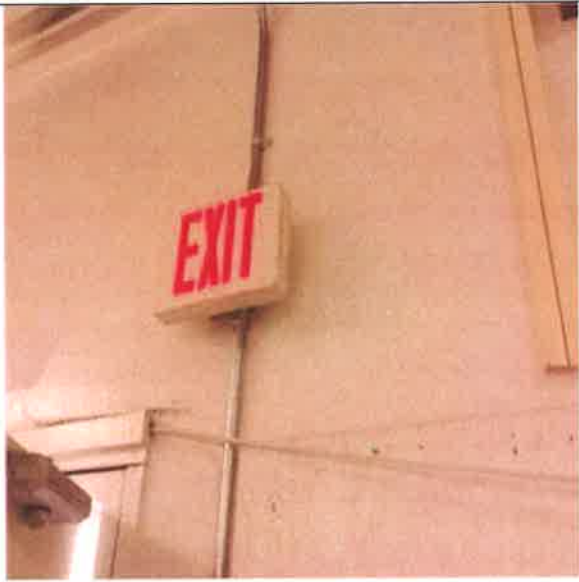
Exit Signs, Illuminated, w/ Battery (per SF) :- Emergency Exit Sign
