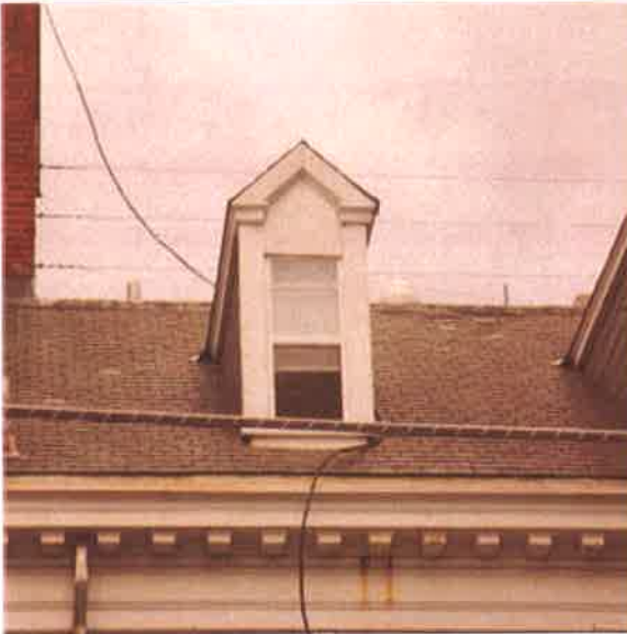
Asphalt Shingle Roof Covering
