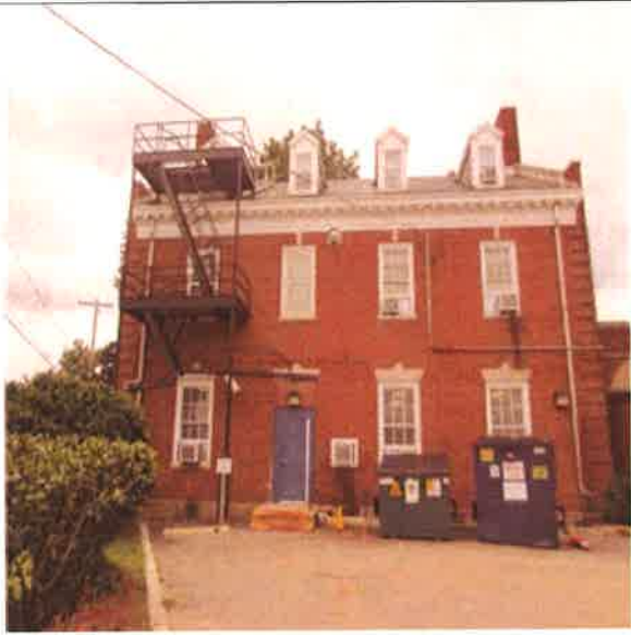
Exterior Walls, Brick Masonry, Solid, Multi-Wythe :- Exterior Brick
