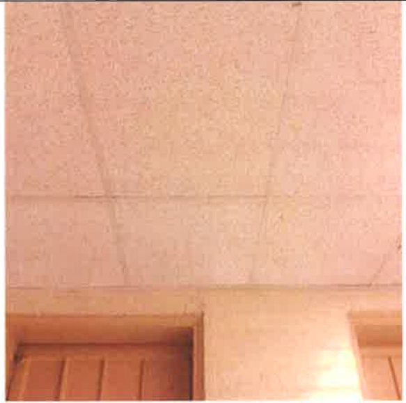
Ceiling Finish, Suspended Acoustical Tiles in Grid:- Suspended Ceiling Tiles
