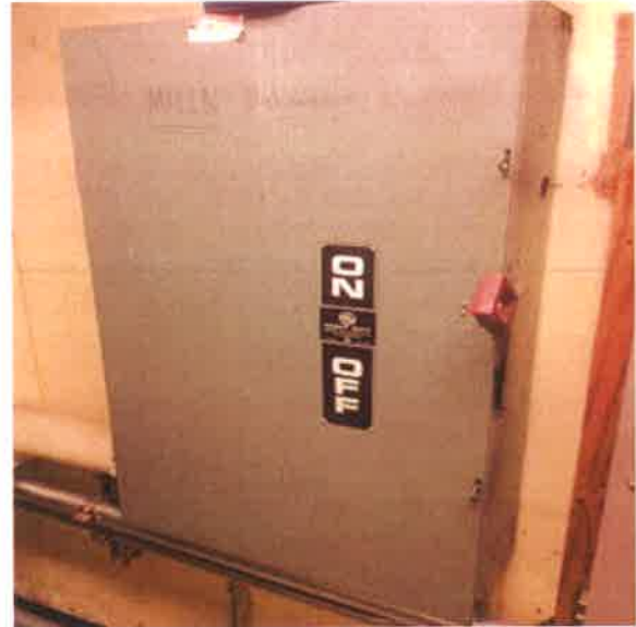
Main Electrical Service, 400 Amp, w/ Main Disconnect(s), Main Distribution Switches:- Main Electrical Disconnect
