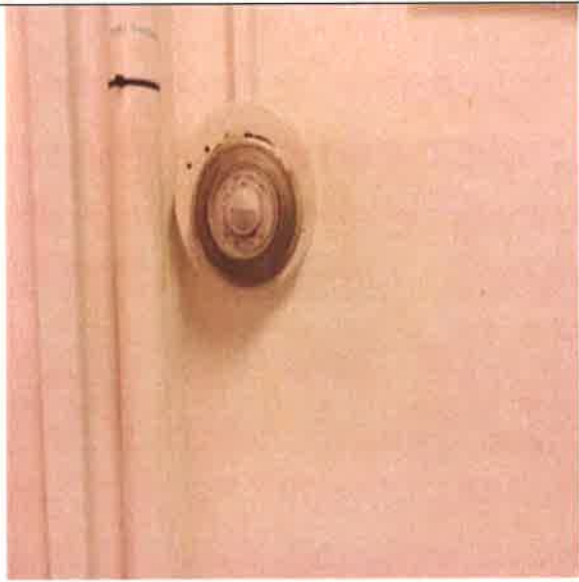
Thermostats :- Analog Thermostat
