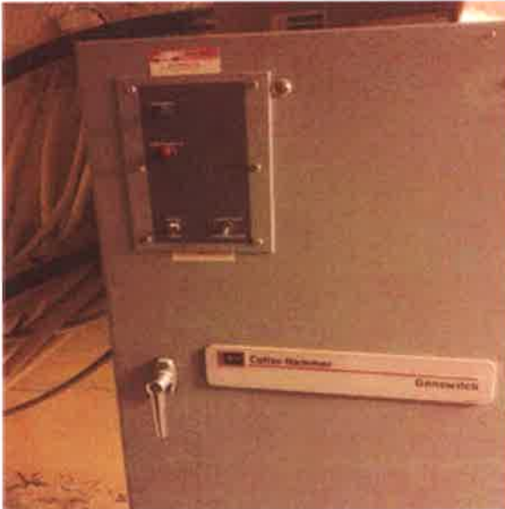
Generator Transfer Switch
