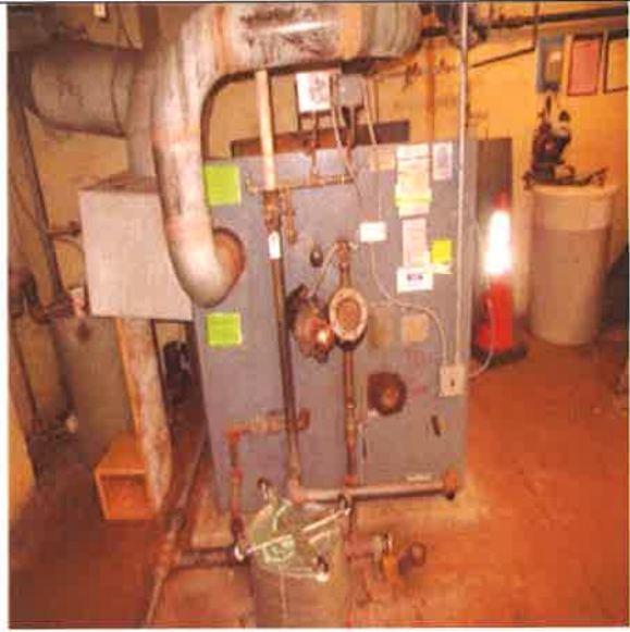
Boiler, Gas, 1,000 Mbh:- Weil McLain Boiler
