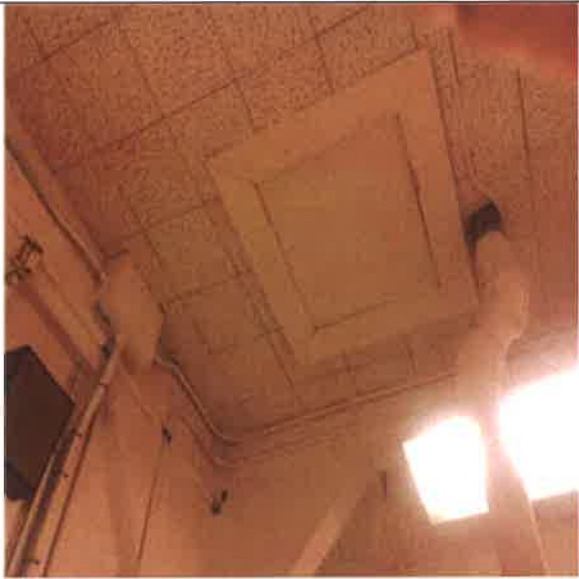
Ceiling Finish, Concealed Spline Acoustical Tile :- Acoustical Ceiling Tile
