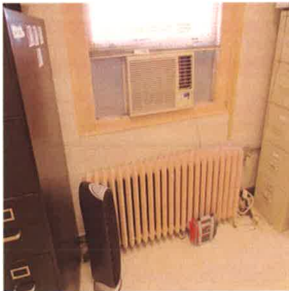
Heating, Cast Iron Radiators or Similar (per SF) :- Typical Cast Iron Hot Water Radiator
