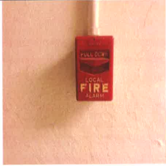
Fire Alarm System, Complete – Standard (per SF):- Fire Alarm Pull Station
