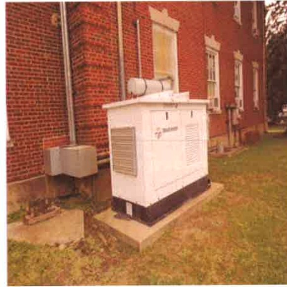
Generator, Diesel, 20 kW:- 20kW Generator
