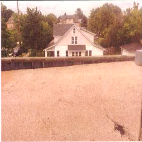
Roof Covering, Built-up Roof :- Built up roof covering with ballast
