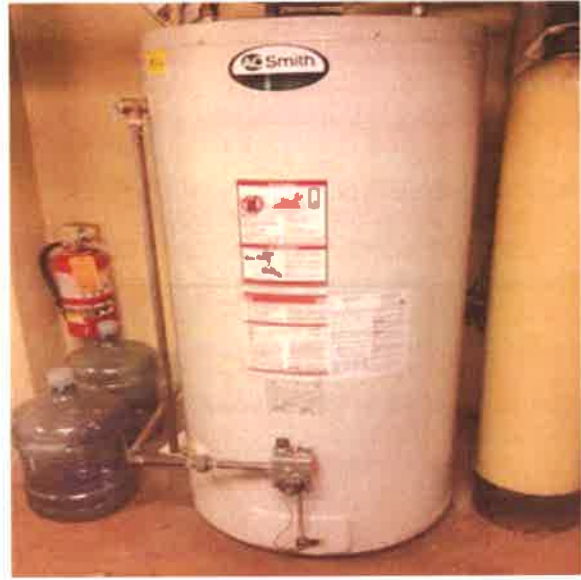
Water Heater, Domestic, Gas, 120 Gal:- A.O. Smith Water Heater
