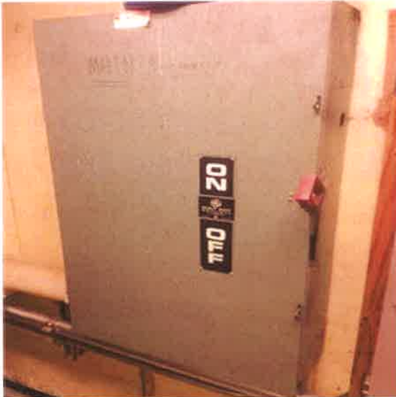
Main Electrical Disconnect
