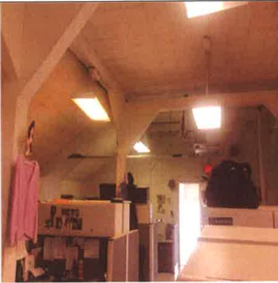
Fluorescent Lighting Fixtures, Average Density (per SF) :- Suspended Fluorescent Light Fixtures
