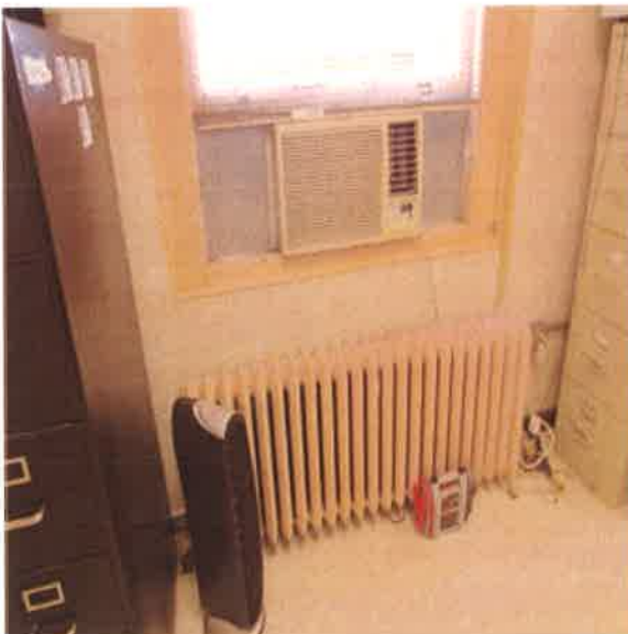
Typical Cast Iron Hot Water Radiator
