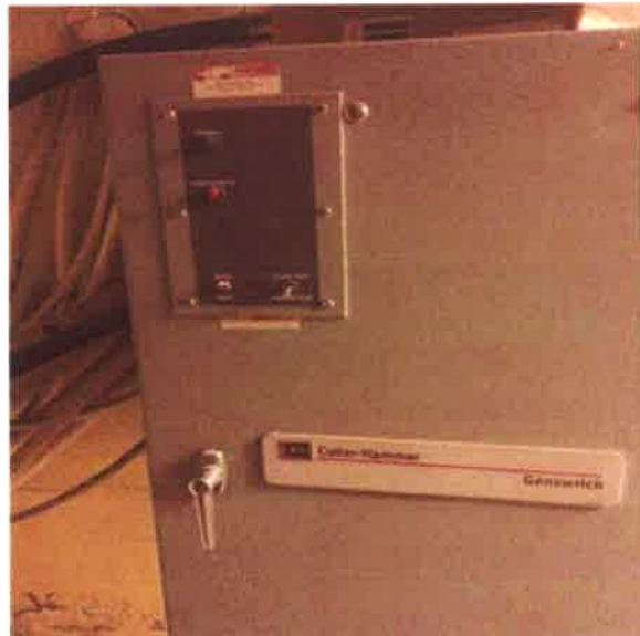
Generator Transfer Switch, Auto, 208 V, 225Amp :- Generator Transfer Switch
