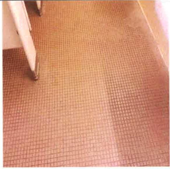
Floor Finish, Ceramic Tile:- 1x1 Bathroom floor tile
