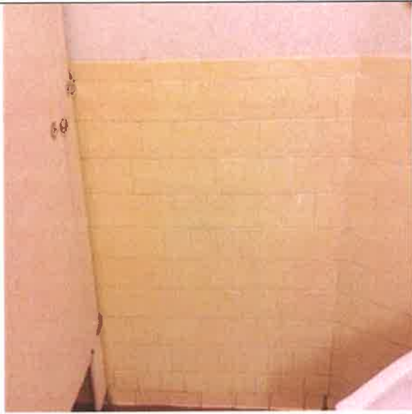
Wall Finish, Ceramic Tile :- Bathroom Wall tile
