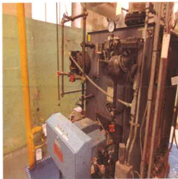
Boiler, Steam, Gas Fired, 1,000 Mbh - Boiler #1 :- Boiler number 1 that isn't functioning.
