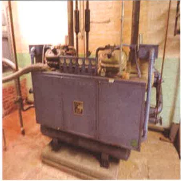
Chiller, Reciprocal, With Air-Cooled Condenser:- Chiller that is not functioning.
