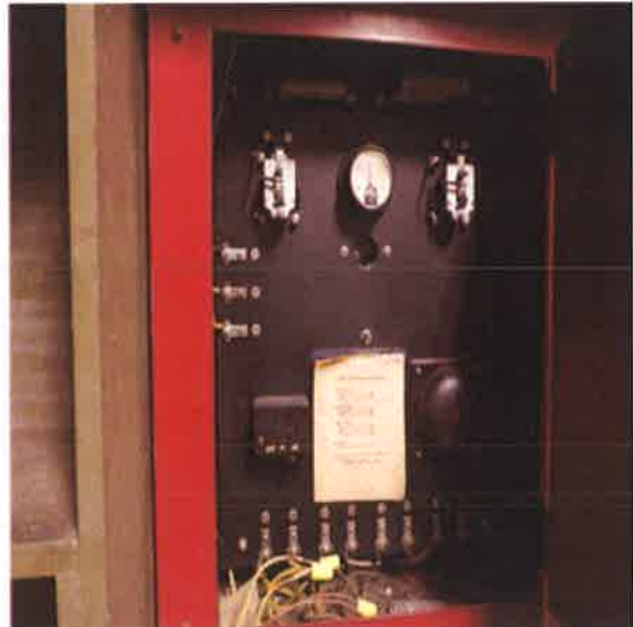
Fire Alarm Control Panel:- Fire alarm panel.
