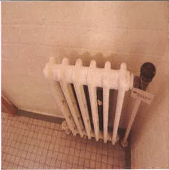
Heating, Cast Iron Radiators or Similar (per SF) :- Cast iron radiator that is found throughout the building.
