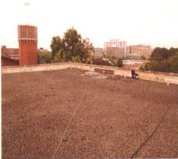
The roof covering consists of a built up roof system.
