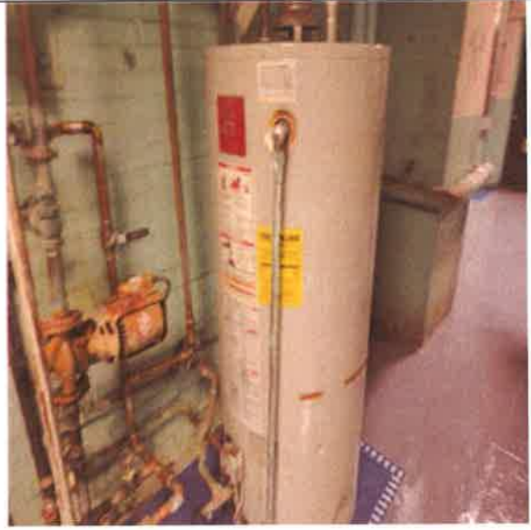
Water Heater, Domestic, Gas:- Gas fire water heater manufactured by State.
