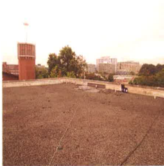
Roof Covering, Built-up Roof :- The roof covering consists of a built up roof system.
