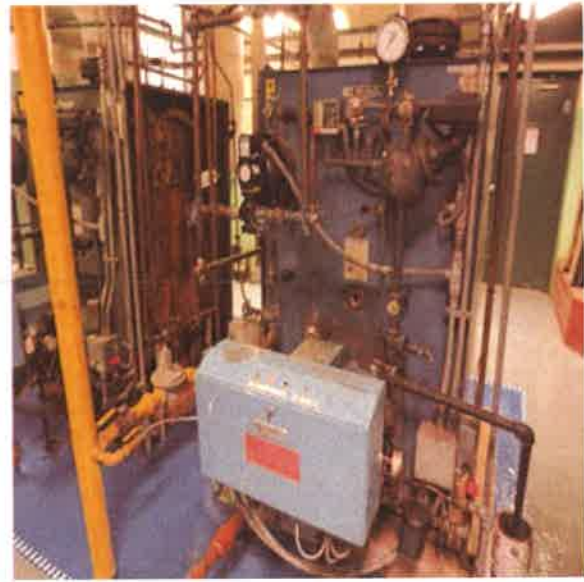
Boiler, Steam, Gas Fired, 1,000 Mbh - Boiler #2:- Boiler #2 that is functioning.
