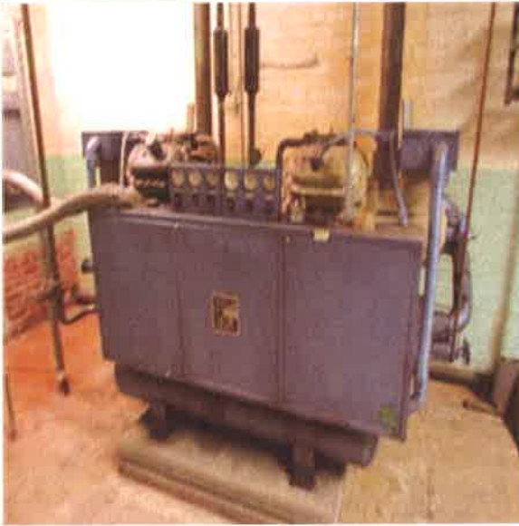
Chiller that is not functioning.
