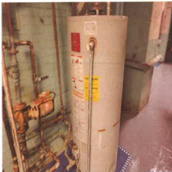
Gas fire water heater manufactured by State.
