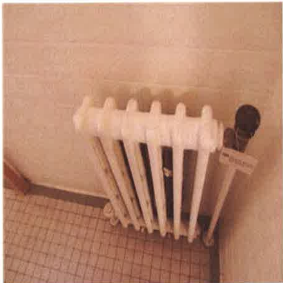
Cast iron radiator that is found throughout the building.
