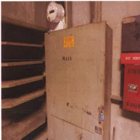
Main Electrical Service, 800 Amp, w/ Main Disconnect(s), Main Distribution Switches :- Main disconnect for the building.
