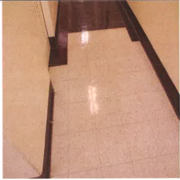
Floor Finish, Vinyl Tile - 12"x12":- Typical 12" x 12" tiles in select locations throughout the building.
