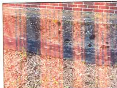
BLACK EXTERIOR WATER PROOFING (CLOSE-UP) EXTERIOR
