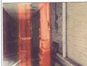
2'-0"-4'-0" PIPE INSULATION (WIDE ANGLE) NORTH MECHANICAL ROOM
