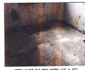
GREEN FLOOR TILE WITH MASTIC (12" X 12") (WIDE ANGLE) ROOM 411
