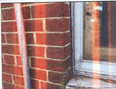
GRAY EXTERIOR WINDOW CAULKING (CLOSE-UP) NORTH EXTERIOR
