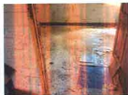
OFF WHITE FLOOR TILE WITH MASTIC (12" X 12") (WIDE ANGLE) ROOM 401
