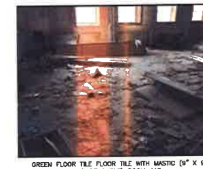
GREEN FLOOR TILE WITH MASTIC (9" X 9") (WIDE ANGLE) ROOM 413
