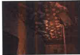
GLUE DOTS OVER 1' X 1' CEILING TILE (WIDE ANGLE) 4TH FLOOR NORTH HALLWAY
