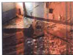
TAN FLOOR TILE WITH MASTIC (9" X 9") (WIDE ANGLE) ROOM 401
