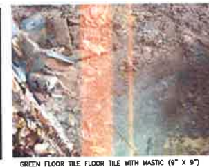
GREEN FLOOR TILE WITH MASTIC (9" X 9") (CLOSE-UP) ROOM 413
