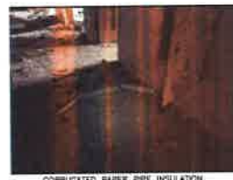
CORRUGATED PAPER PIPE INSULATION (WIDE ANGLE) ROOM 420F
