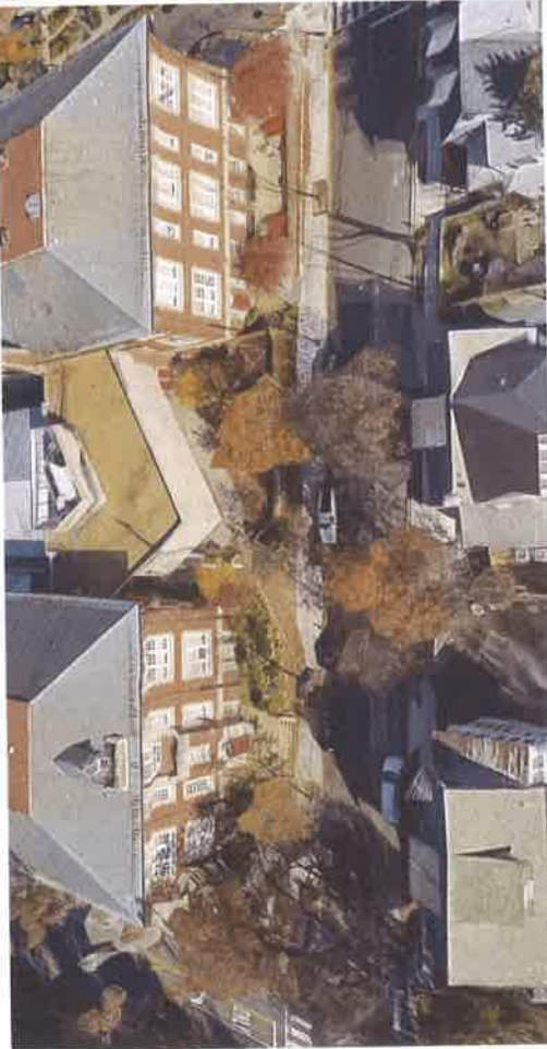
Figure 1 - Aerial view, Lowell Street
