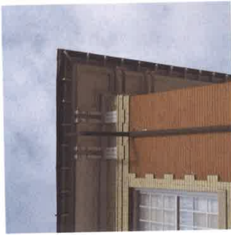
Figure 7 – Gutter distress.
