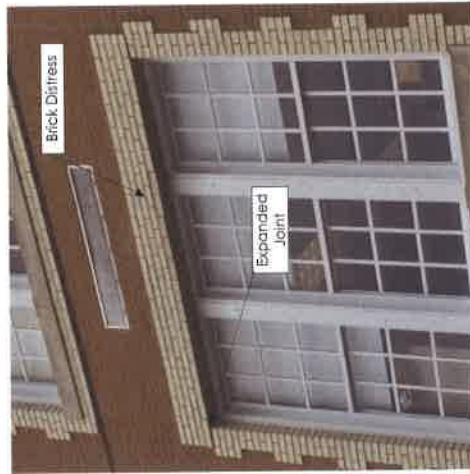
Figure 2 – Expanded joint at lintel beaming & brick distress.
