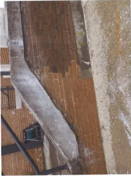
Rear pedestrian stairs and ramp showing cracking and deterioration
