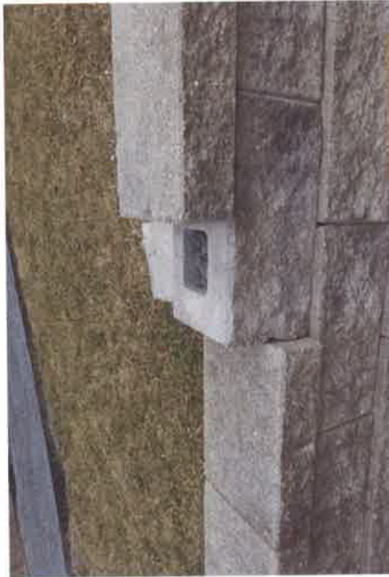
Minor, isolated exception to perimeter hardscape being in good condition
