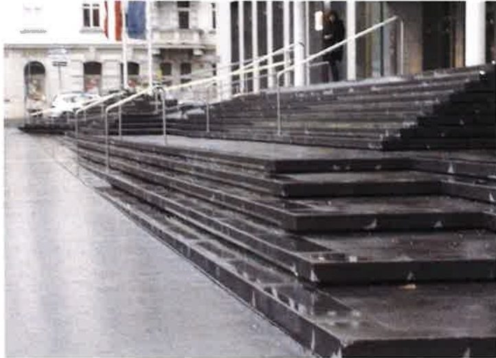
LANDSCAPE STEPS AT ENTRY PLAZA
