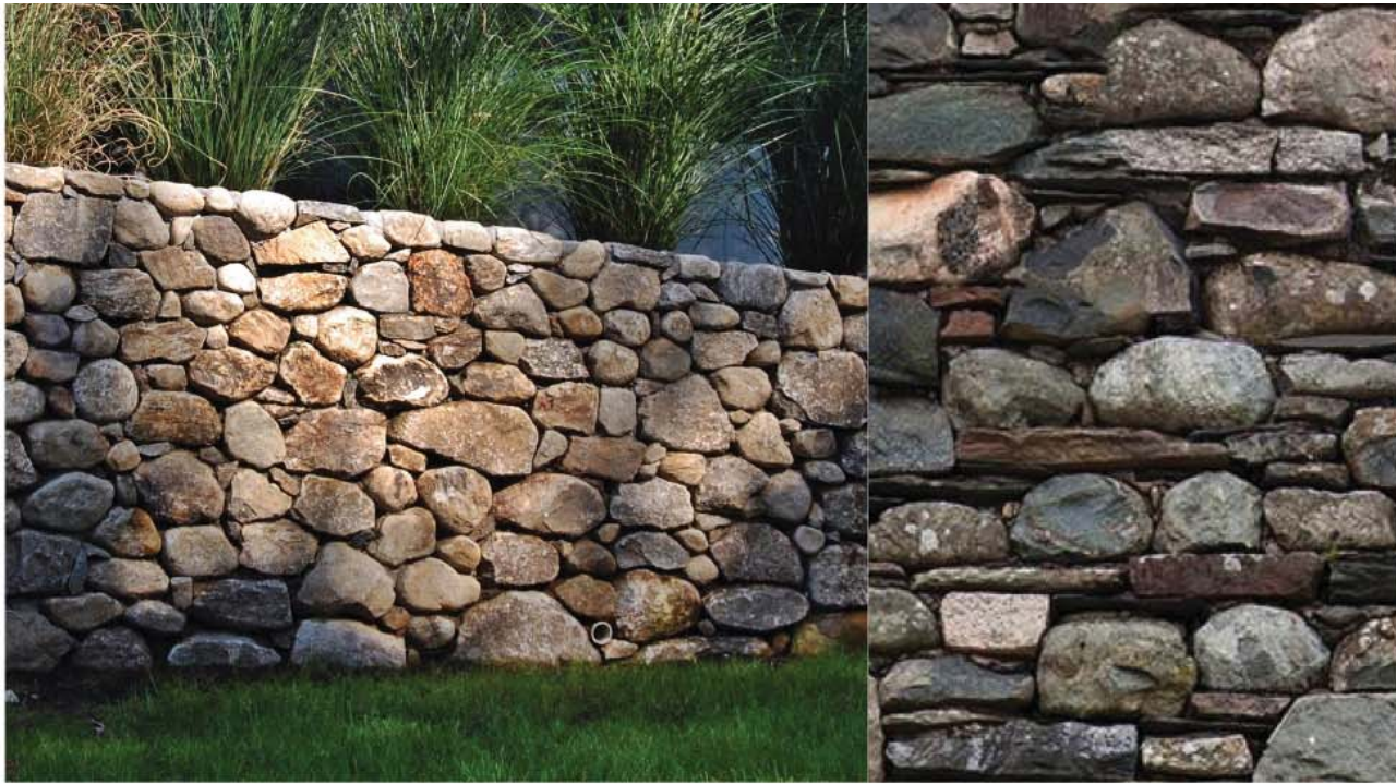
Rubble Stone Retaining Wall
