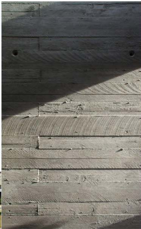
Board Formed Concrete
