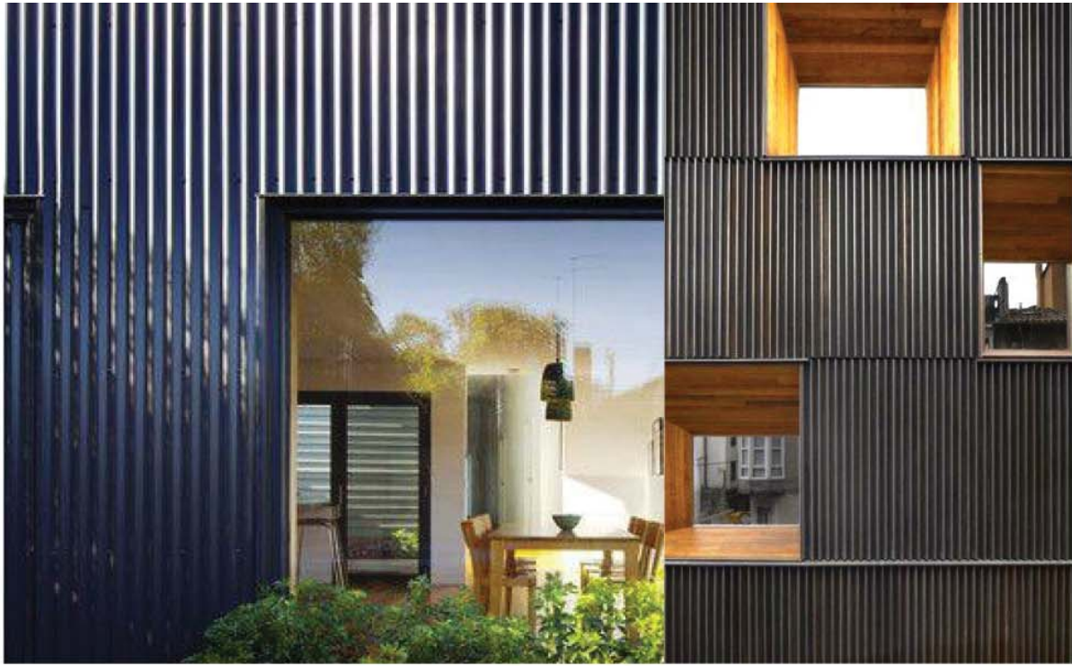
Vertical Profiled Metal Panel
