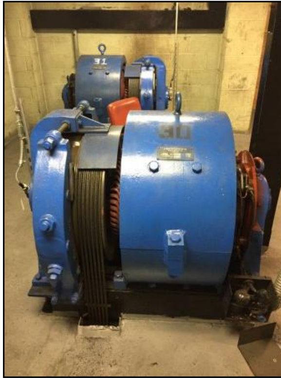
electric elevator motor
