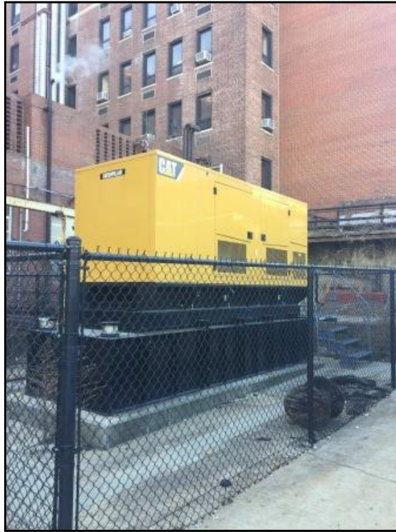
backup generator at the core buildings
