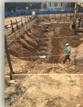
Install of Heel Blocks/Rakers/Lagging
