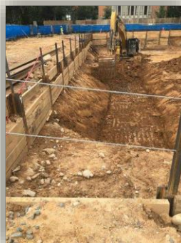
Excavation for elevator, crane and mud mat
