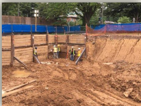
Install of Sheathing and Shoring
