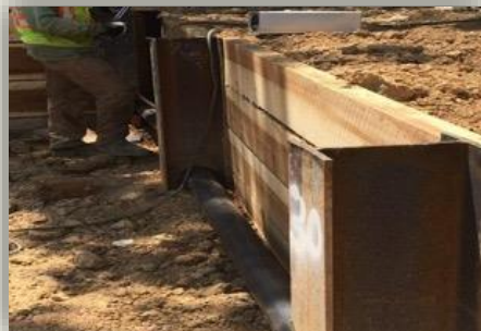
Installation of Sleeves for Utility Pipe
