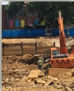
Sheathing and Shoring
