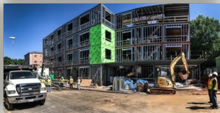
Building Fully Erected
