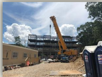
Modules Being Erected
