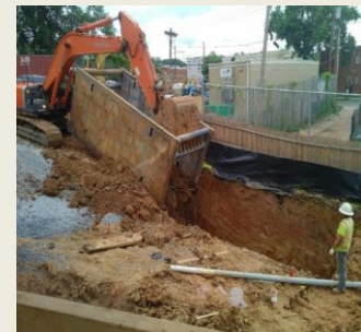
Excavating for Electrical Vault
