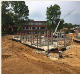
Erecting Podium Steel
