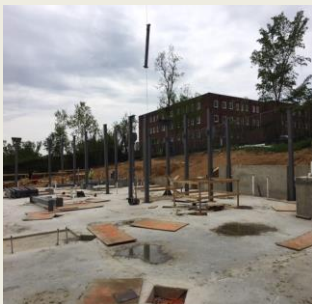
Slab on Grade Poured
