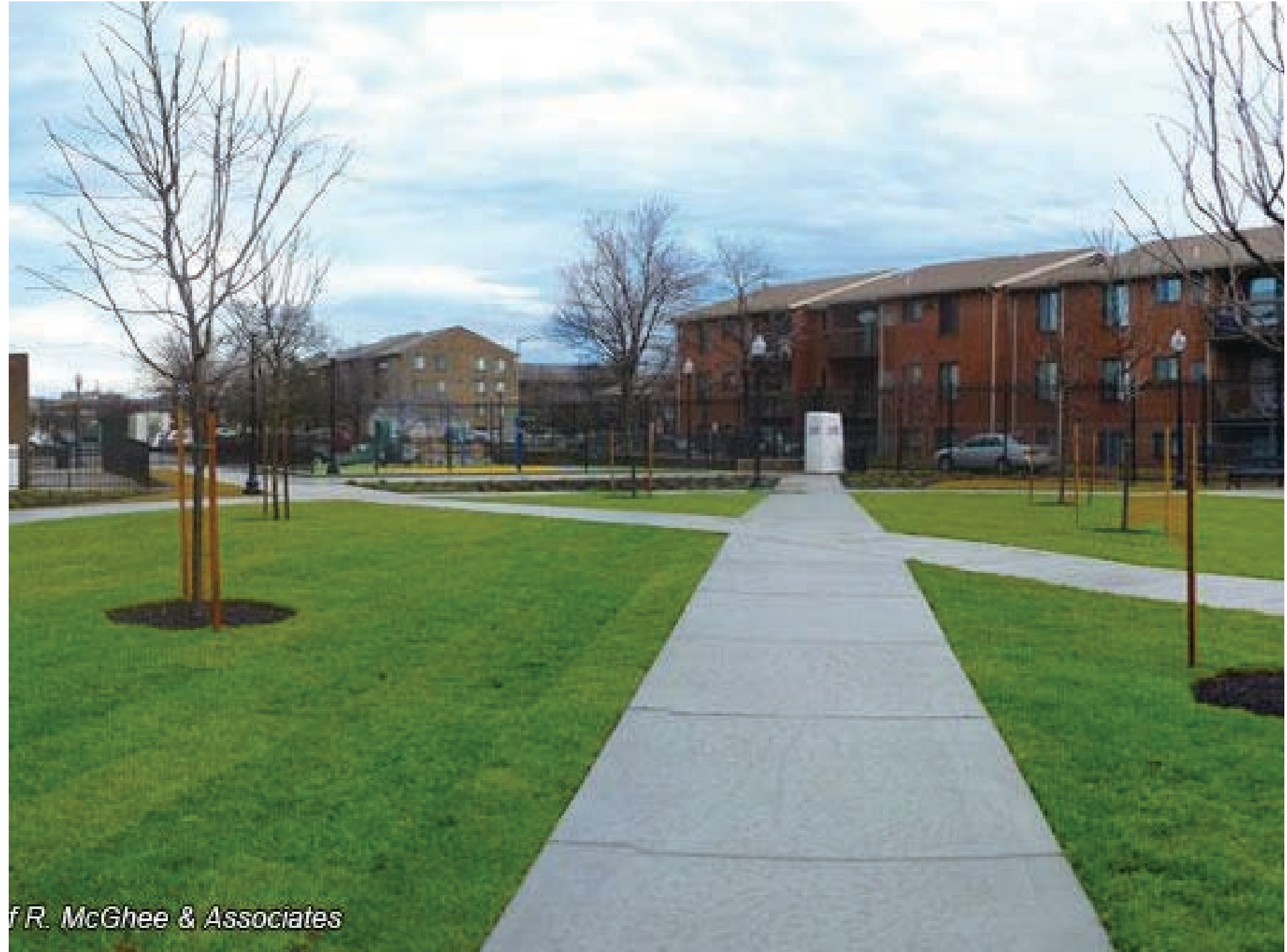
DPR Park Grass and Trees – After Remediation
