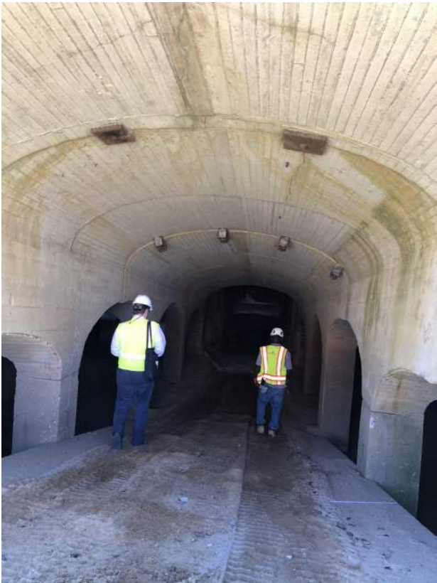
BARREL VAULT AT FILTER CELL ENTRANCE FROM SOUTH SERVICE COURT
