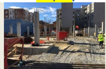
[Concrete Columns 90% Complete]
