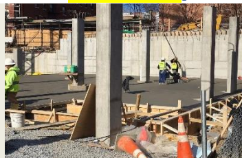
[1 st Floor Level Slab Pour Up To Column Line 3]
