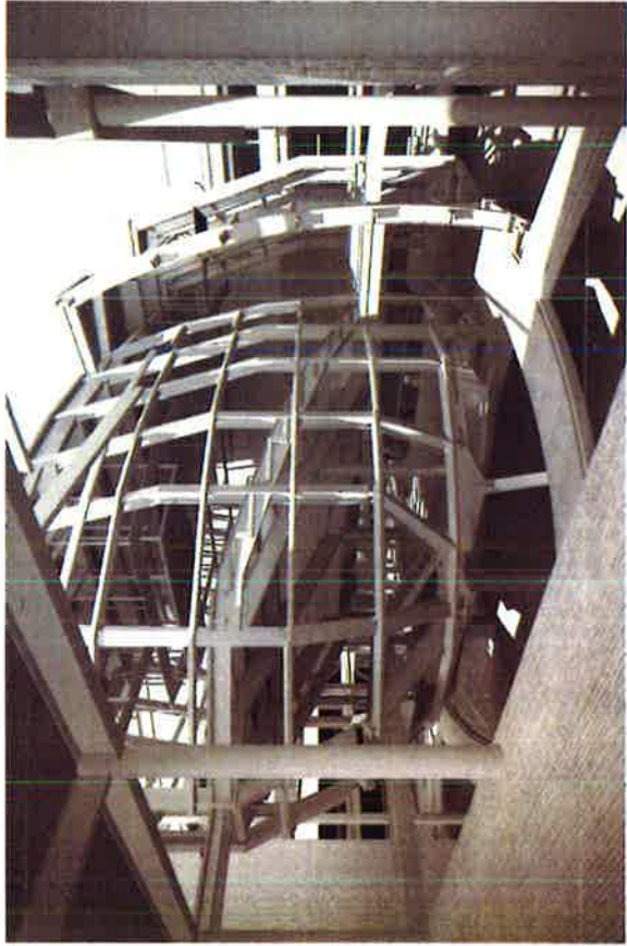
Rendering of Duke Ellington Structural Framing and Atrium
